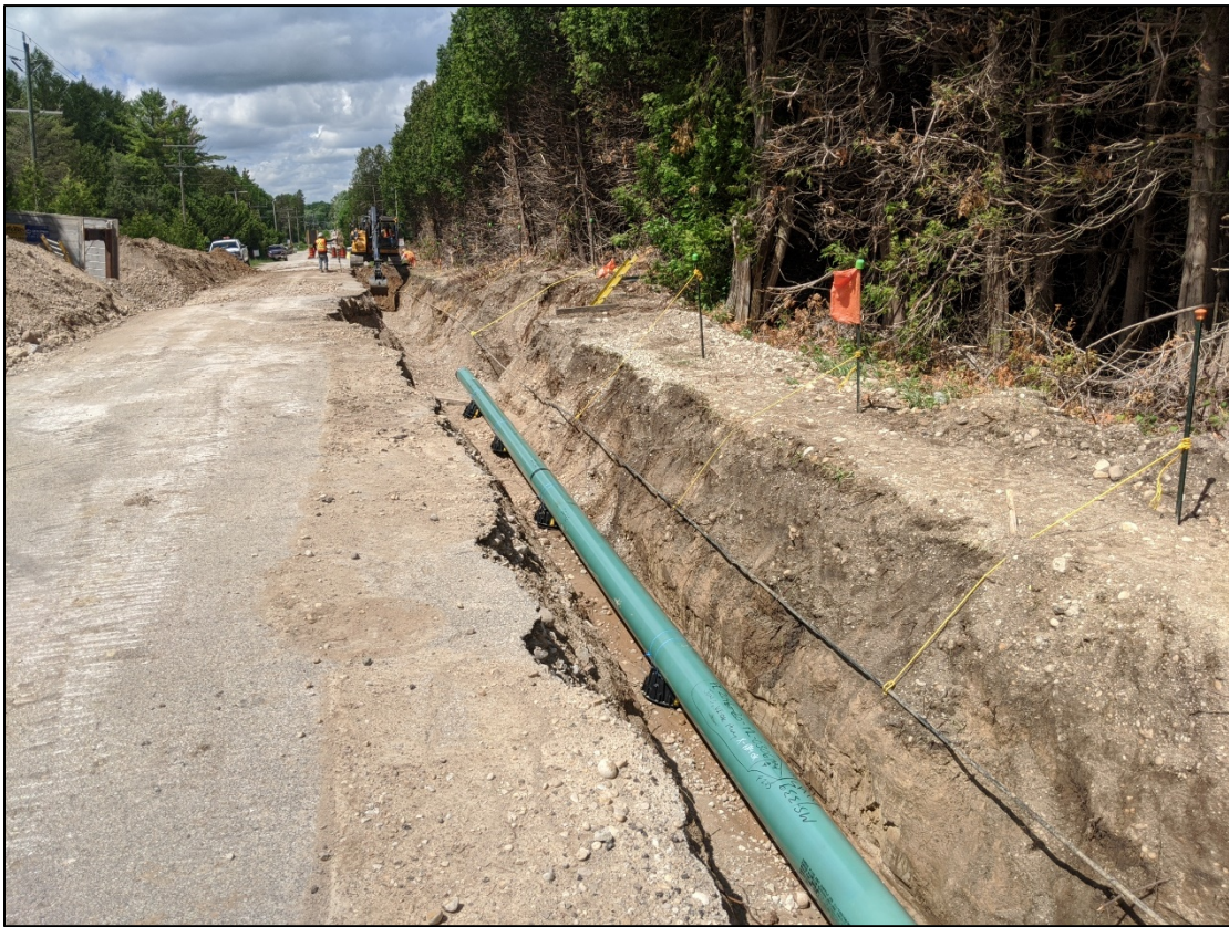
1. Pipeline being installed via trenching along Concession 2 in the Township of West Grey
