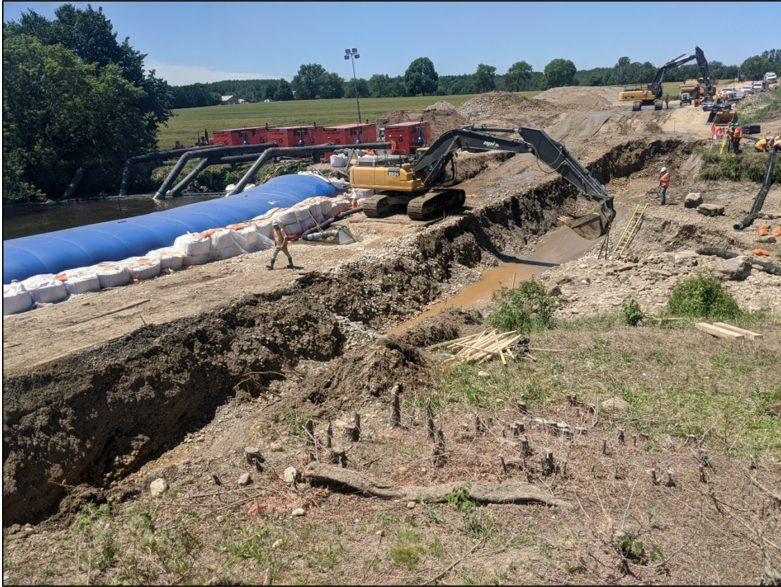
3. Open-cut pipeline installation across the Saugeen River in the Township of West Grey.
