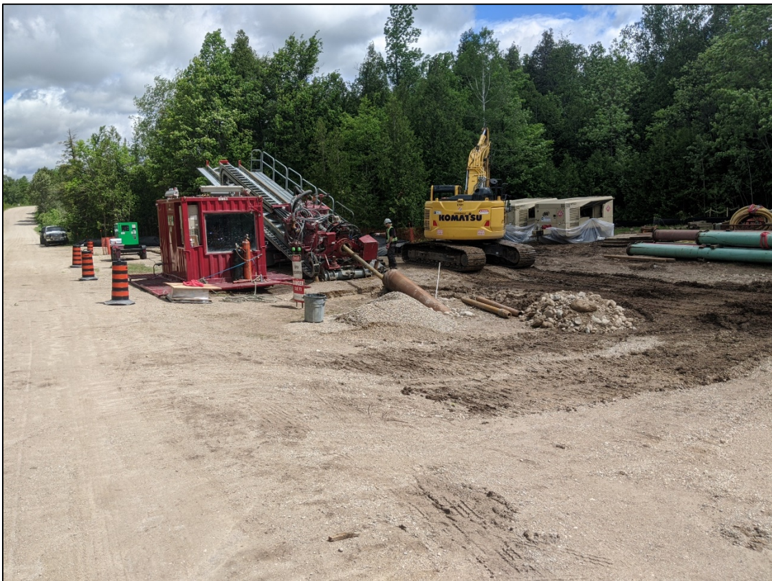
2. Pipeline installation via horizontal direction drilling under the North Saugeen River, along Concession 4.
