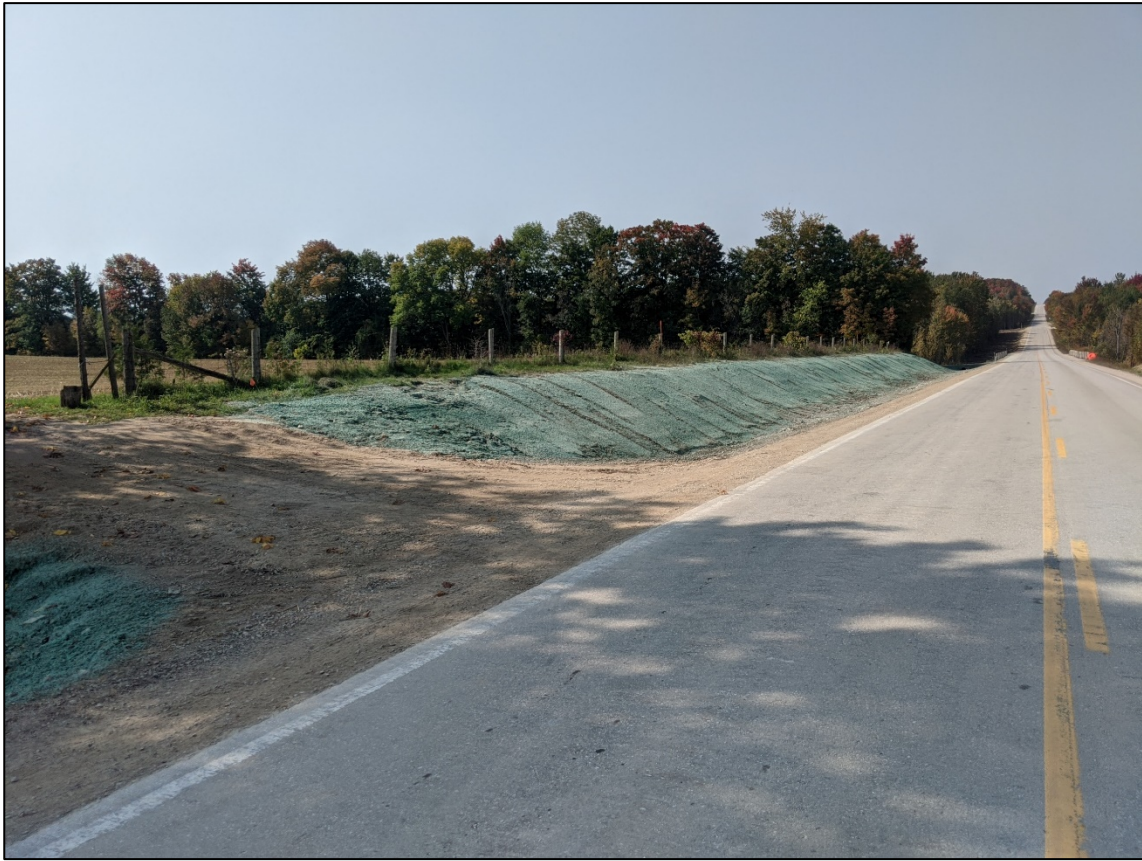
5. Hydroseeding of restored roadside banks along Highway 25, Grey County.
