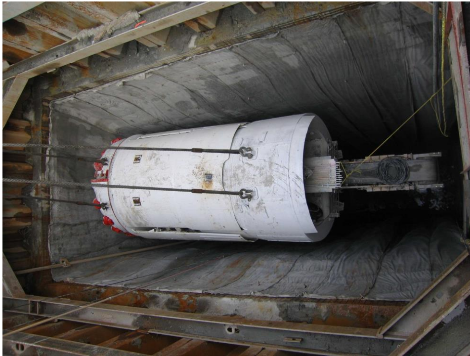
Figure 5 – Example Tunnel Boring Machine
