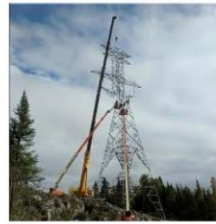
4 Tower Erection
