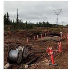
5 Stringing Conductors (Wires)
