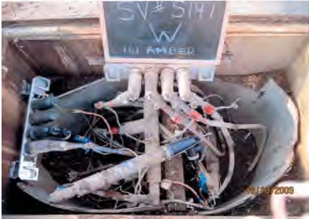
Figure 30: Typical Switching/Splice Vault on PUC Distribution System
