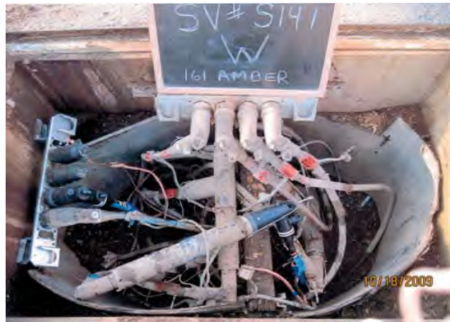
Figure 4-24: Underground Splice/Switching Vault
