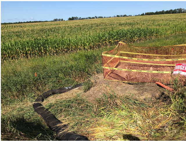
Photo 13: Silt Soxx™ installed around drill pad location at intersection of Simcoe St. and Farmstead Rd., looking west (August 2019)
