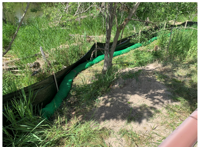
Photo 18: Inadvertent release protection measures established on Concession Rd. 6, west of Sideroad 18 (June 2020)
