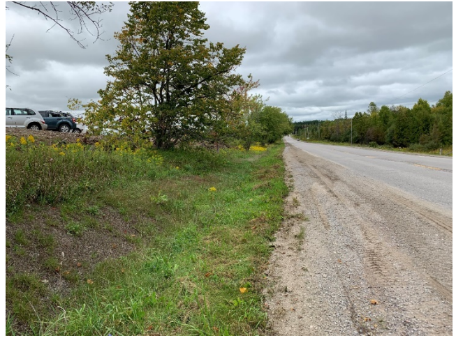
Photo 26: Reclaimed and stabilized drainage ditch in KCA Disturbed Area #2 on Simcoe St., one year after restoration, looking north (September 2020)
