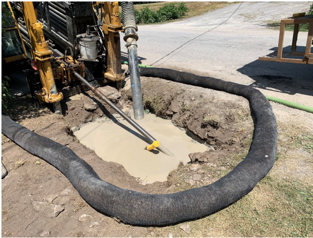
Photo 19: Silt Soxx™ containment around HDD entrance pit along Concession 6 (June 2020)
