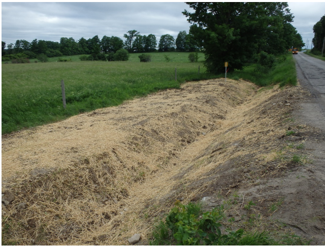
Photo 1: Placing topsoil and straw for stabilizing a road ditch on Taylors Rd., south of Quaker Rd. looking north (June 2018)
