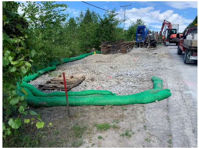
Photo 20: Silt Soxx™ established at HDD entrance pit at 1361 Concession 6, looking east (July 2020)
