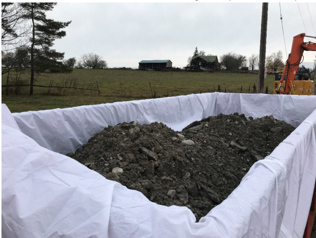
Photo 11: Storing potentially contaminated soil on Hwy. 35, south of Hwy. 121 (November 2018)
