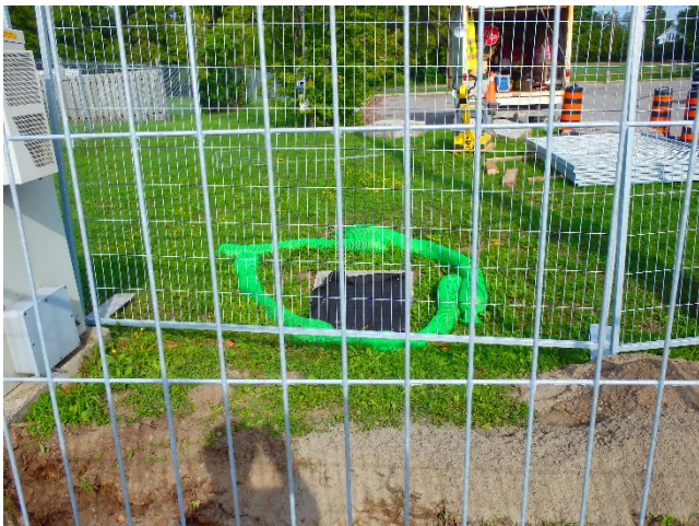
Photo 5: Protecting stormwater intakes in the Community of Fenelon Falls at North St. (August 2018)
