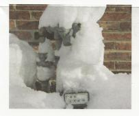
During the winter it's important to keep your outdoor natural gas meter and exhaust vents free of snow and ice. A gas meter covered in snow or ice can impede its ability to regulate the pressure of the gas supplied to your home, which could lead to serious risks for you and your family. Gently brush off snow or ice with a soft broom or brush and never use a sharp tool like an ice scraper. Also be careful not to bump your meter with a shovel or snow blower.
