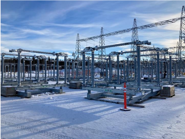
Marathon – 11 remaining switches for station expansion assembled and grounded awaiting installation
