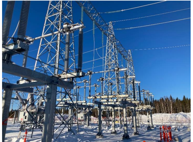
Marathon – newly installed switches on East side of yard
