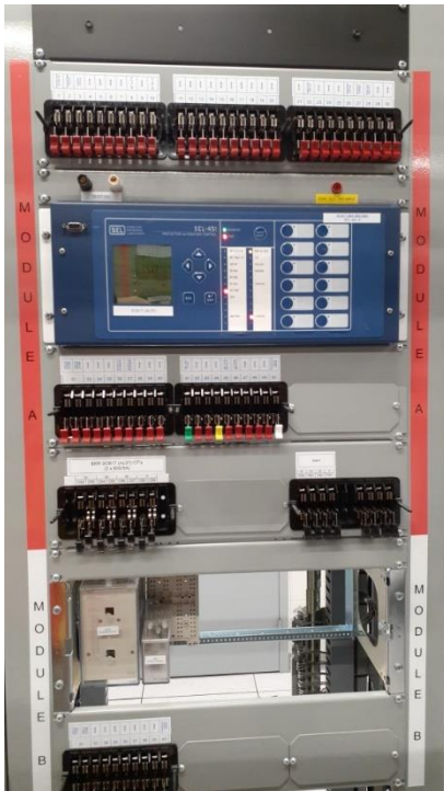
Marathon – Racks wired and powered up containing various protections and control IED (Intelligent Electronic Devices) modules to monitor lines and yard equipment as well as control of breakers and switches
