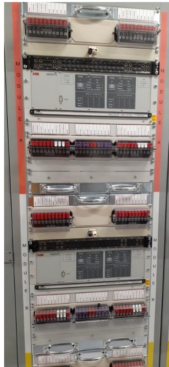
Marathon – Racks wired and powered up containing various protections and control IED (Intelligent Electronic Devices) modules to monitor lines and yard equipment as well as control of breakers and switches
