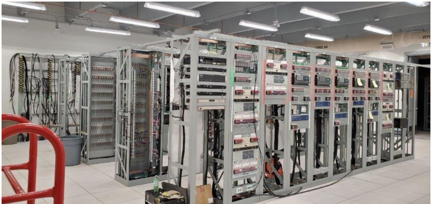
Wawa – new PCT building room 'A' protection and control panels
