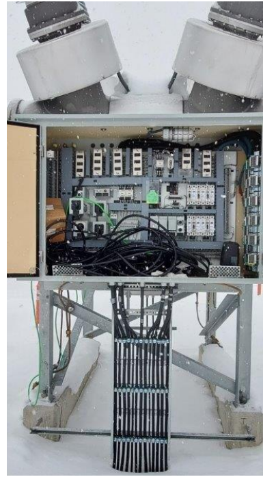
Wawa – Bay 4 breaker mechanical box wired
