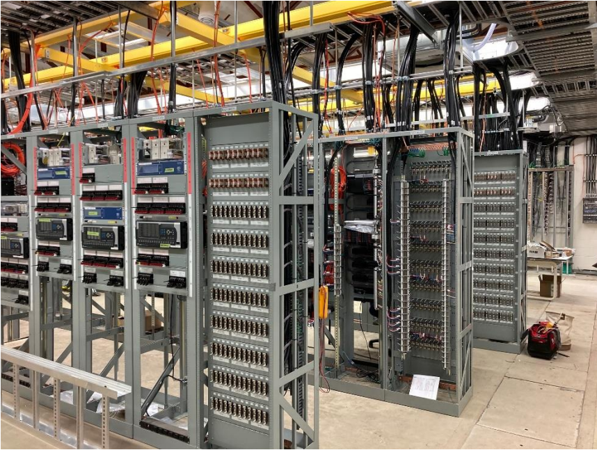
Lakehead – ongoing protection cable pulling in the A building
