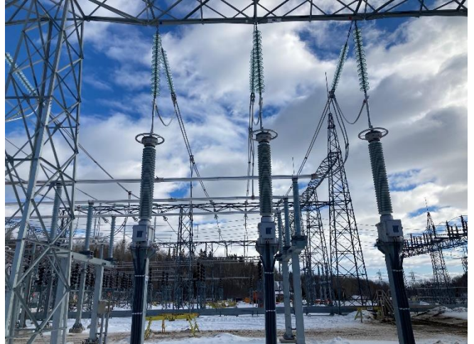
Lakehead – newly installed strain bus drops to P bus CVT's in bay 9
