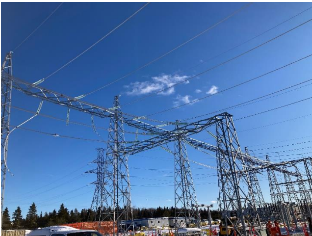
Marathon – newly installed L35.L36,W1,W2 strain bus
