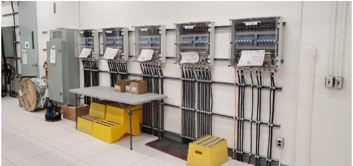
Wawa – new PCT building DC monitoring cabinets
