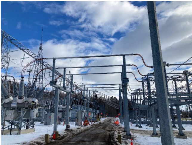
Lakehead – newly installed rigid/strain bus over road crossing in Bay 9,10
