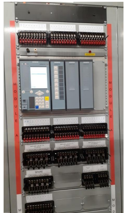
Marathon – Racks wired and powered up containing various protections and control IED (Intelligent Electronic Devices) modules to monitor lines and yard equipment as well as control of breakers and switches
