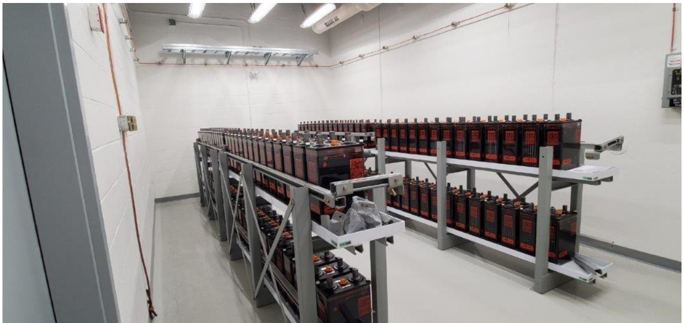
Wawa – new PCT building room A' batteries
