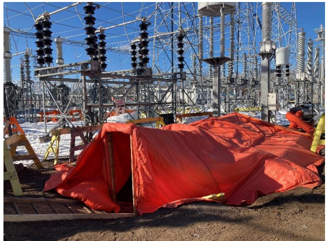
Lakehead – heating & hoarding of rock anchor install at section 14
