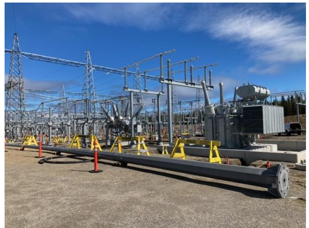
Marathon TS - lightning spike ready to be lifted, R3 steel, rigid bus and breaker installed
