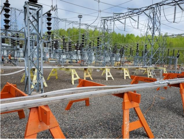
Lakehead TS - newly assembled strain bus prepped for H and P bus outages
