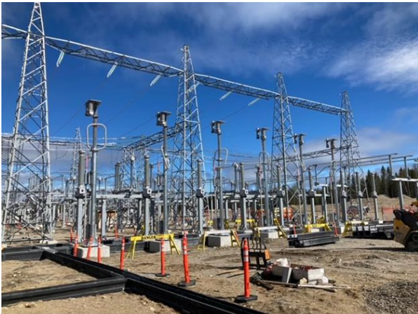
Marathon TS - W35M, W36M GRI ground switches freshly installed
