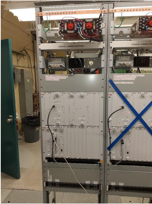
Marathon TS – Telecommunications racks to communicate over fiber networks
