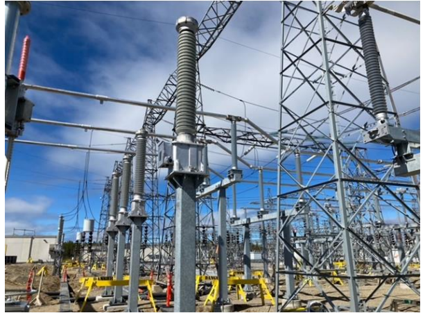
Marathon TS - R3 CVT's and rigid bus work/ expansion joint welded
