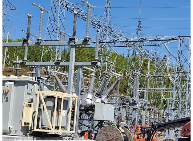
Lakehead TS - R1 reactor, CB-R1 breaker, and R1 switch assembled and installed
