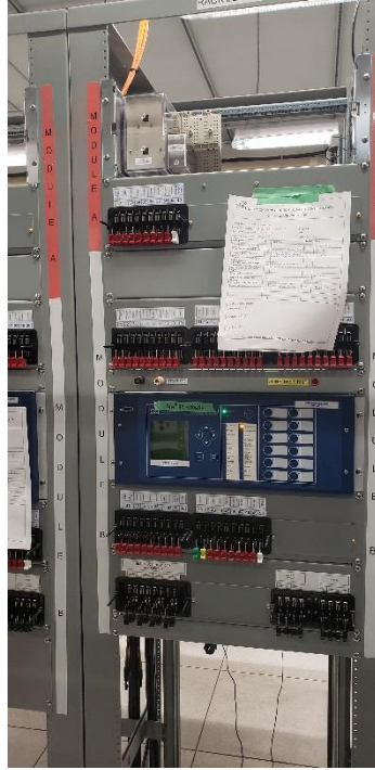
Lakehead – Breaker Fail “A” (left) and Breaker Fail “B” (right)
