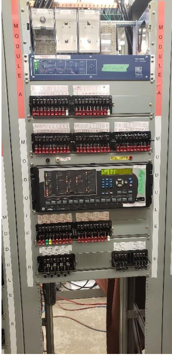
Lakehead – Breaker Fail “A” (left) and Breaker Fail “B” (right)
