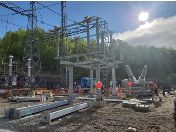
Lakehead TS - newly installed switches and steel installed in bay 14
