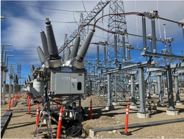
Marathon TS - Cables pulled to a newly installed breaker with half the strain bus drops
