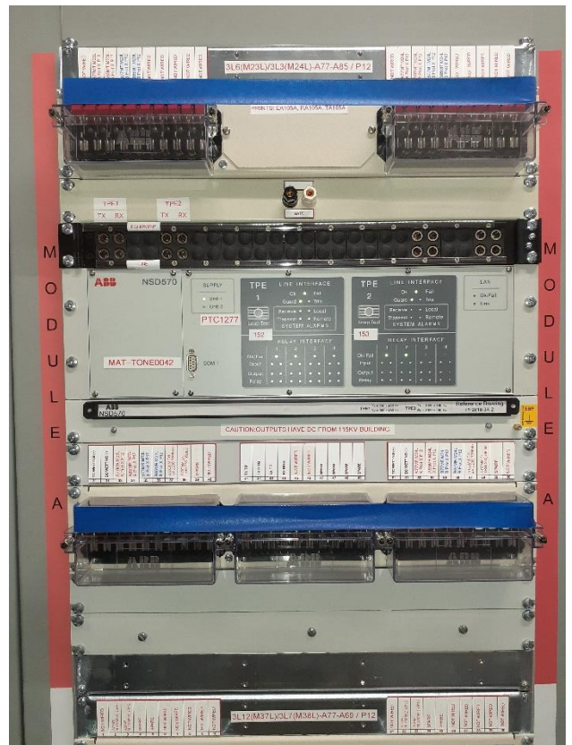
Marathon TS – Telecommunications racks to communicate over bell copper networks
