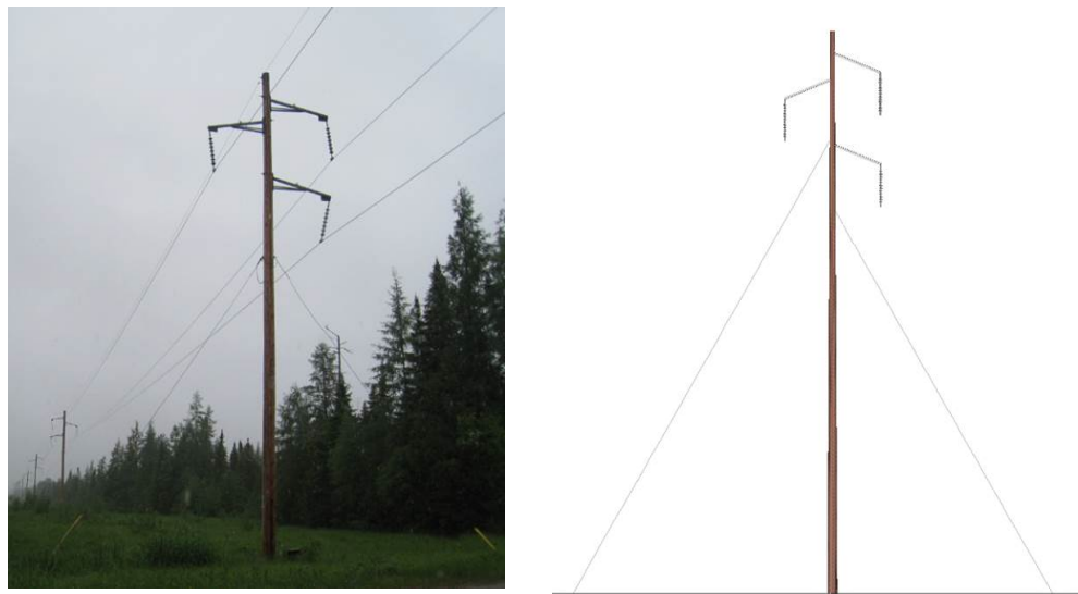
Figure 1: Picture of a single-pole suspension structure along the A8K and A9K circuit with steel harp arms adjacent to a virtual rendition of the same structure.
