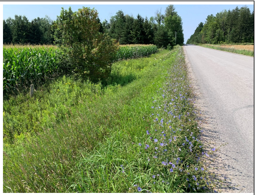
Photo 5b: Reclaimed ditch between Flos Road 6 and Flos Road 5 (July 2021).
