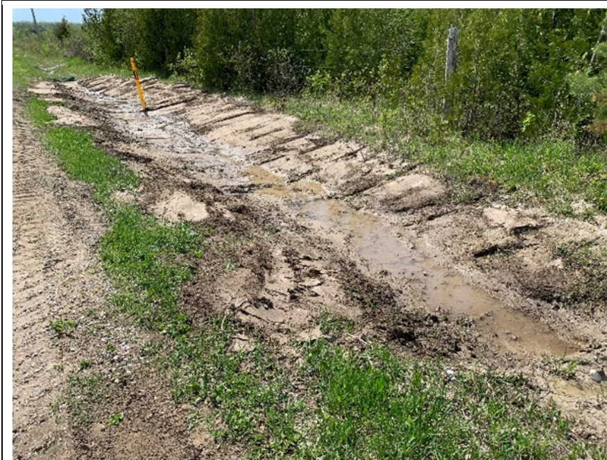
Photo 1a: Soft ditch on Flos Road 8, reclaimed and seeded (May 2020).
