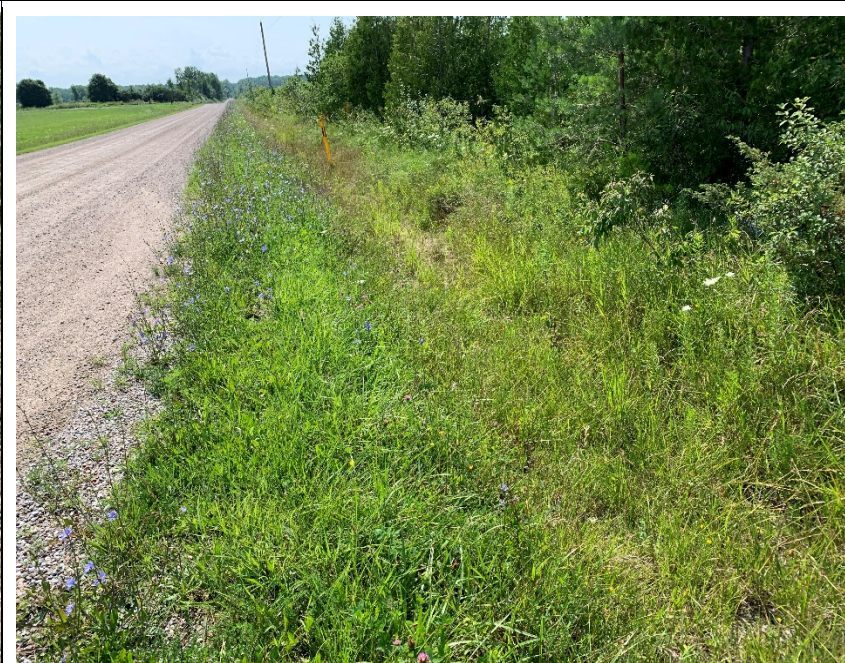
Photo 1b: Road ditch on Flos Road 8 with excellent vegetation establishment (July 2021).
