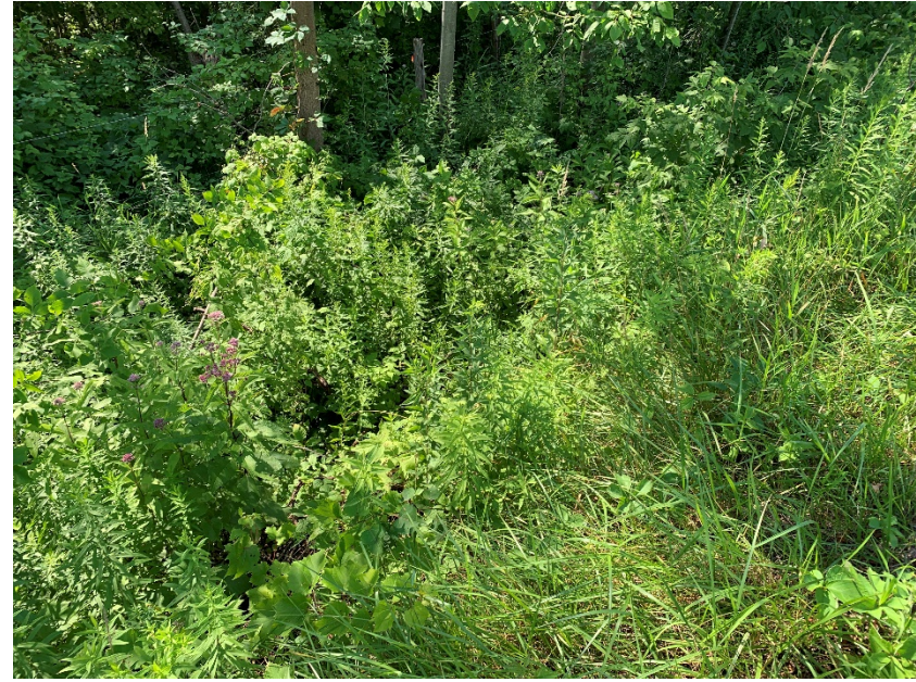
Photo 4b: Stabilized road ditch in the general location where the Silt Soxx™ was installed between Flos Road 7 and Flos Road 8 (July 2021).
