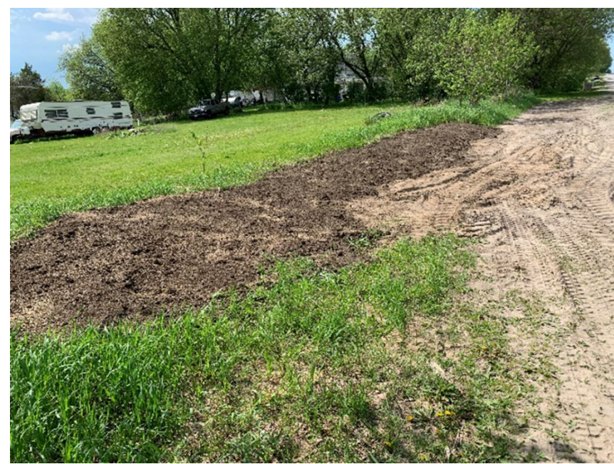
Photo 3a: Topsoil and seed placed on sandy embankment just south of Flos Road 8 (May 2020).
