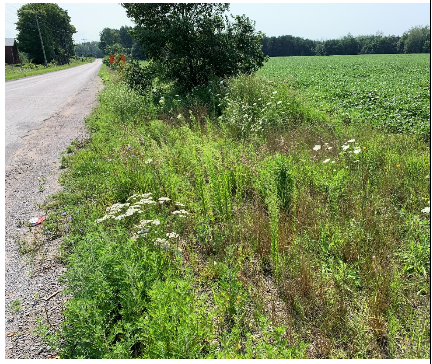
Photo 10: Reclaimed ditch at the tie-in location at Flos Road 4 (July 2021).
