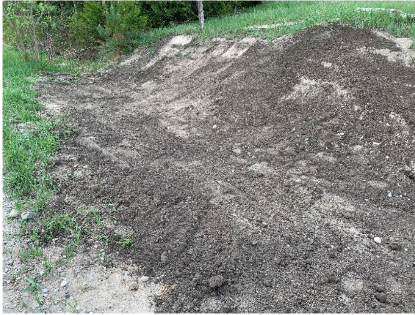
Photo 2a: Sandy embankment on Flos Road 8 which has topsoil and seed applied (May 2020).
