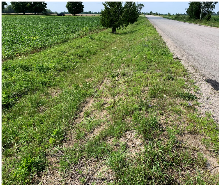
Photo 9: Reclaimed ditch between Flos Road 5 and Flos Road 4 with moderate vegetation establishment anticipated to naturally revegetate over time (July 2021).
