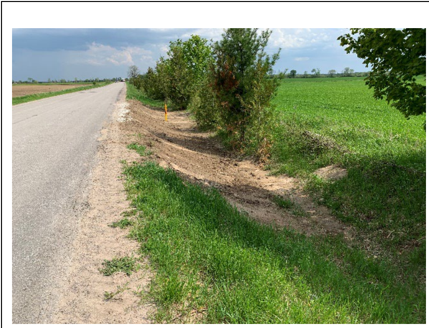
Photo 5a: Road ditch between Flos Road 6 and Flos Road 5 (May 2020).
