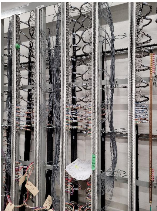
Wawa – terminal racks for cable pulling and terminations
