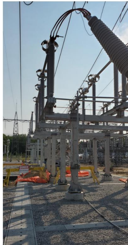
Wawa – Bay 3 1000MCM strain bus installation
