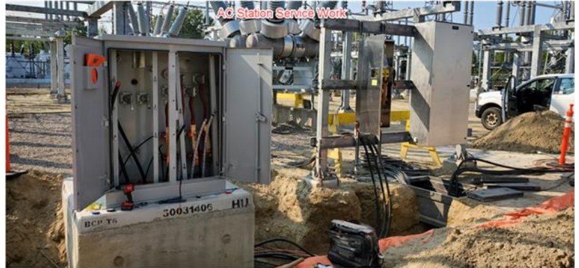
Wawa – AC Station work
