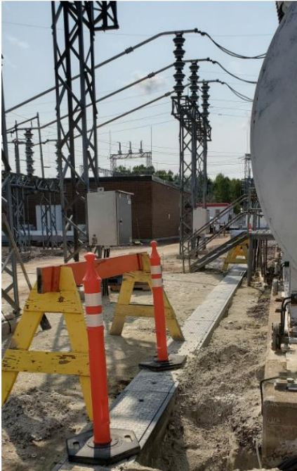
Wawa - ATS install for existing breakers
