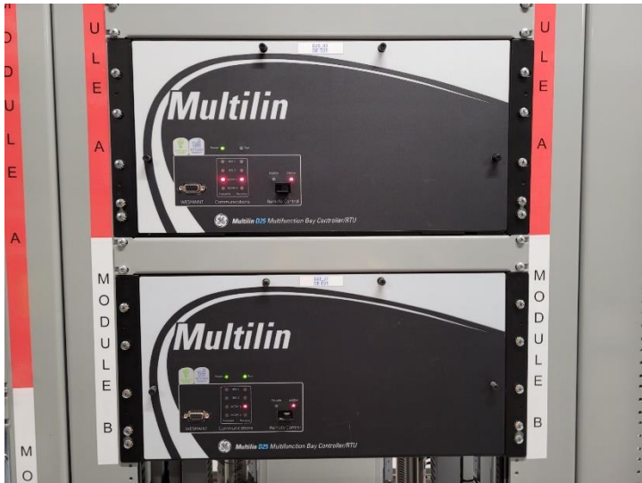
Marathon TS – D25 RTU X 10 controller
