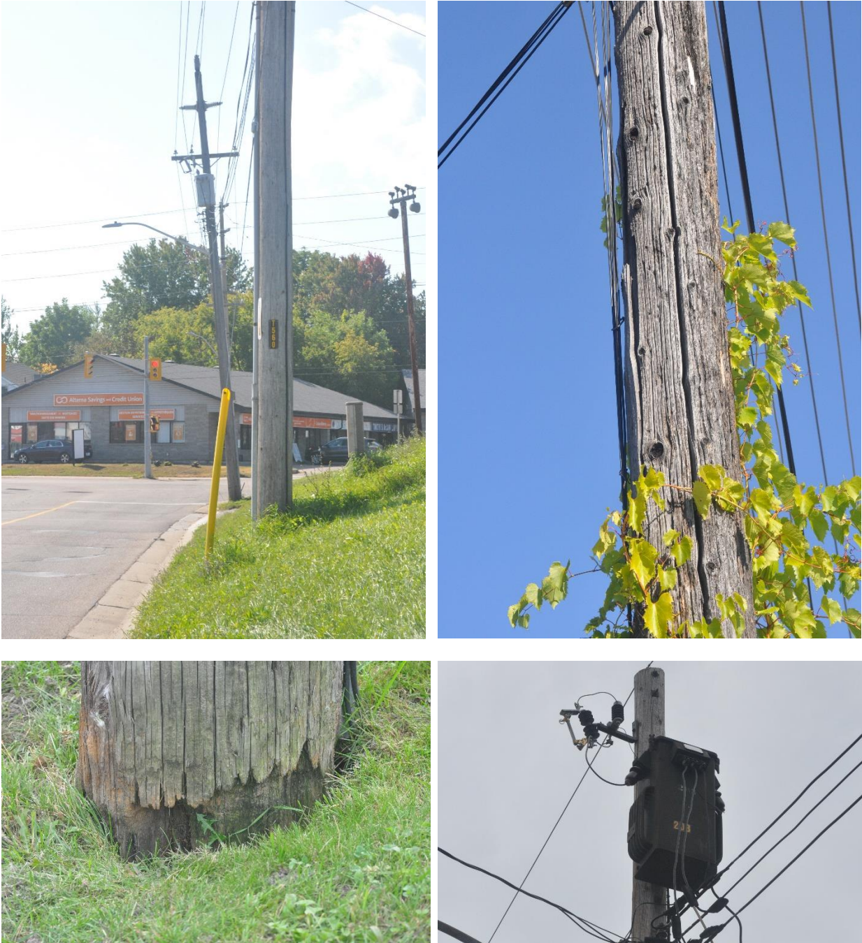
Figure 6-3: Examples of Deteriorated & Aging Overhead Assets
