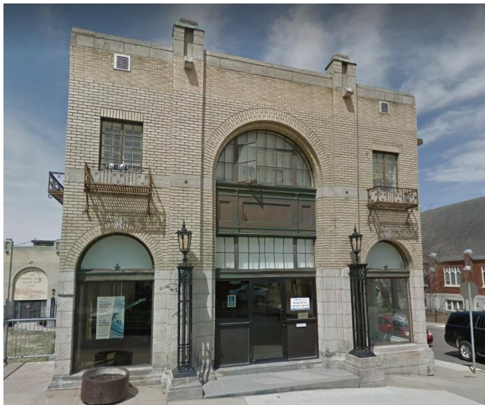
Figure 8-1: Pembroke Service Centre / Main Office Building
