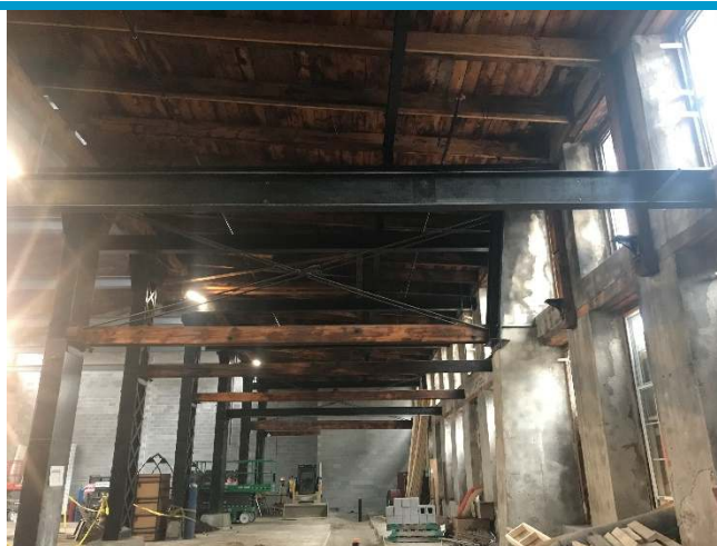
Figure 2 – Structural Roof Reinforcing.
