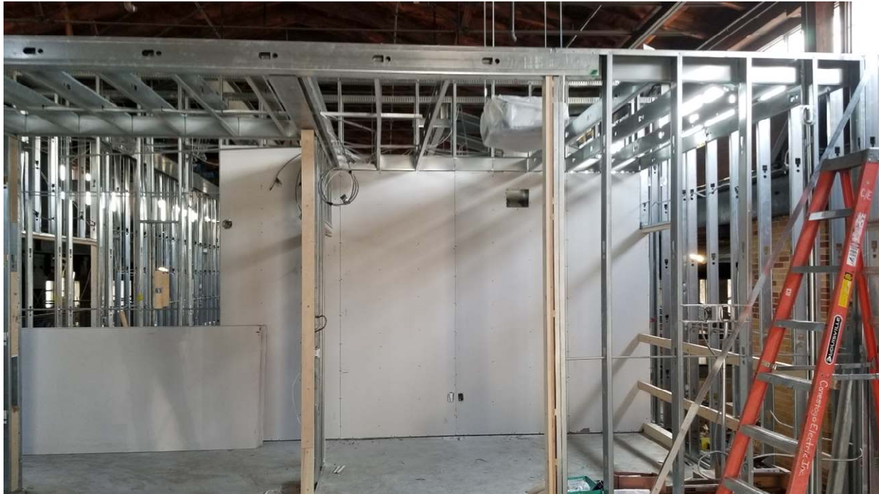
Figure 1 – Stud and Board Installations (Level 2)
