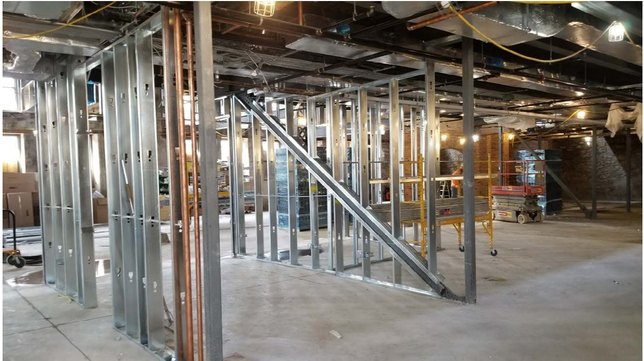
Figure 4 – Laydown area and stud framing (Level 1)
