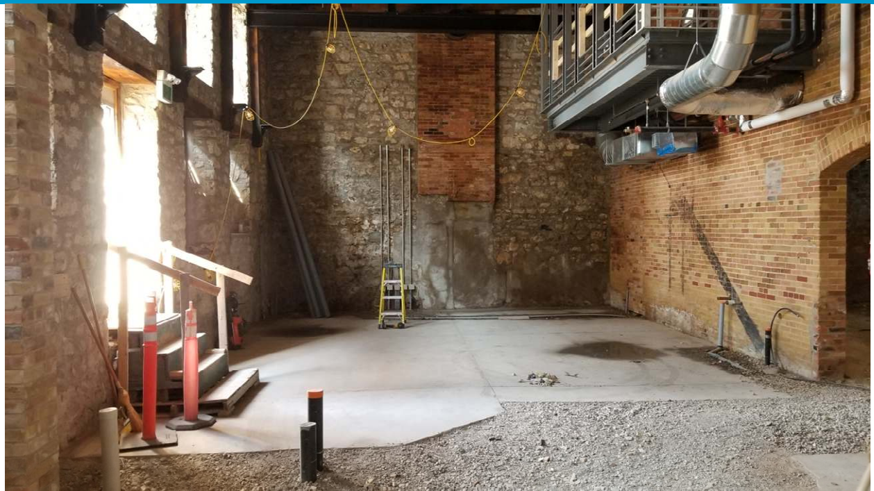
Figure 2 – Floor Clearing in Preparation of Cupolex Installation (Level 1)
