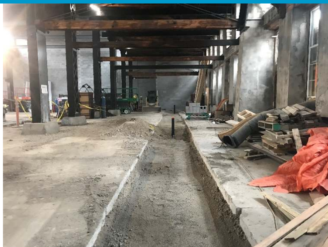
Figure 1 – Underground plumbing
