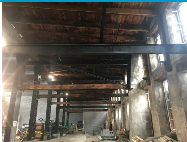
Figure 2 – Structural Roof Reinforcing.
