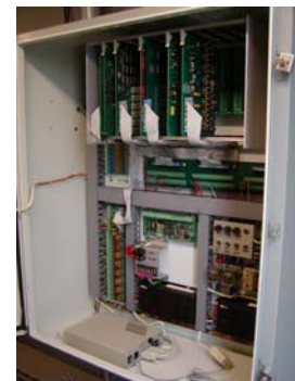
Figure 4-5, Typical Supervisory RTU
