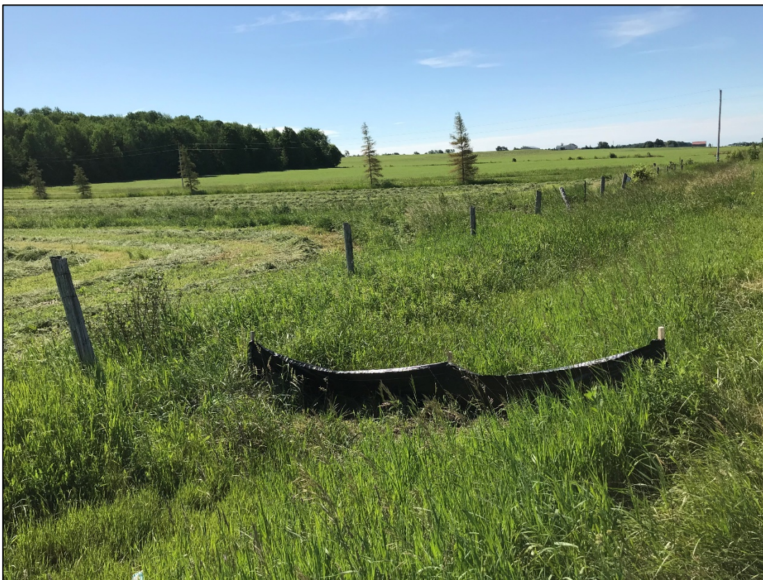
4. Silt fencing was left in place until disturbed areas were fully re-vegetated.
