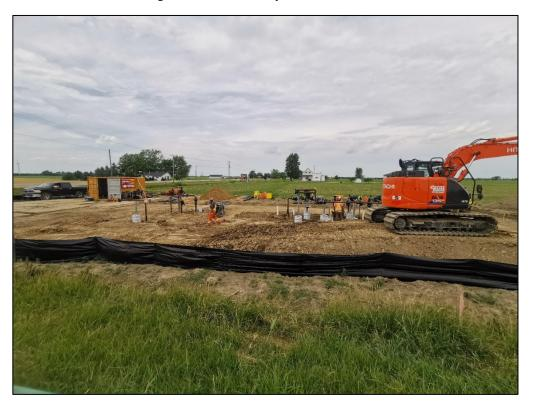
2. Topsoil was stripped and separated for station construction and erosion and sediment controls installed.
