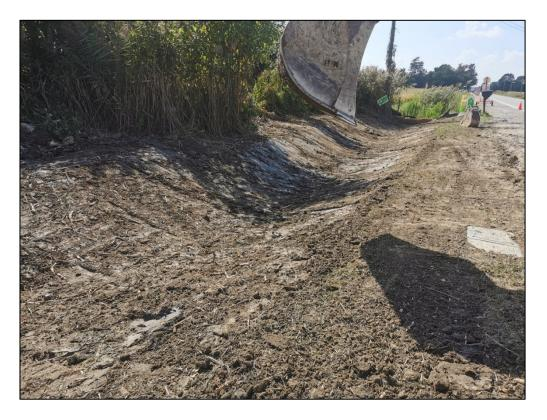
4. Once work is completed at each location swales, drains and watercourses were restored to profile, seeded and erosion sediment controls remained in place until adequate vegetation grew.
