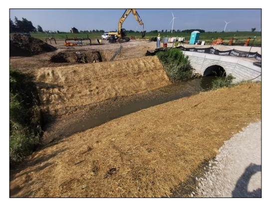
1. Watercourse restoration work – Bank profile was restored to pre-construction profile, area was seeded and erosion matting was installed and keyed in.
