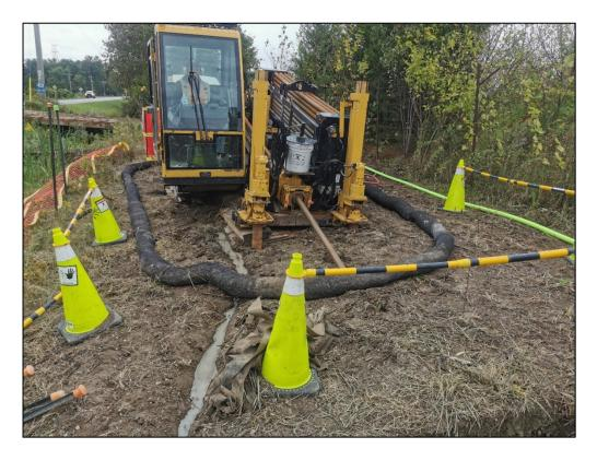
3. Standard controls for equipment included fencing and erosion and sediment controls were installed.
