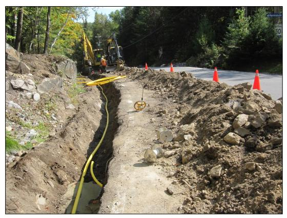
2. Where rocky conditions were encountered, a trench was excavated to allow for pipeline installation.
