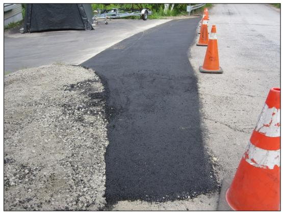
5. Where it was necessary to open cut driveways, they were restored as soon as possible following pipeline installation.
