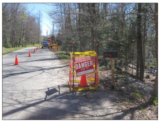
4. Protective fencing and signage were used around open excavations as a public safety measure.
