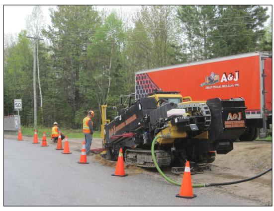
1. The pipeline was installed via horizontal directional drilling where ground conditions allowed.
