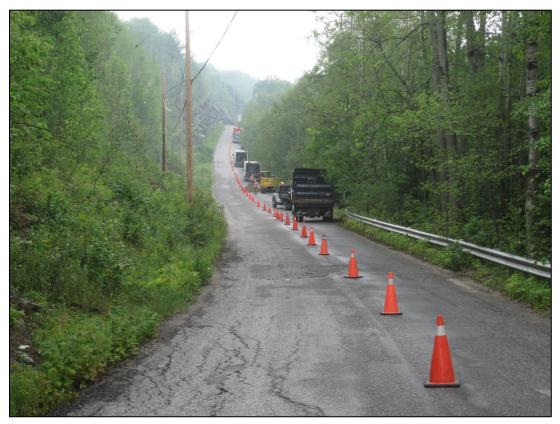
3. At least one lane of traffic was maintained and flag persons and warning devices were used to notify traffic of construction in accordance with Ministry of Transportation standards.
