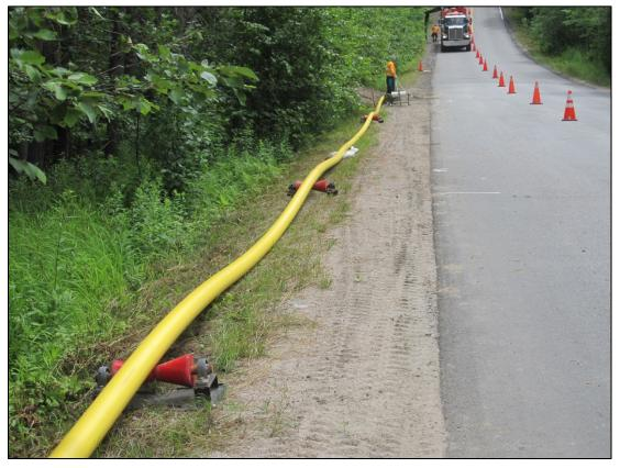
6. The pipeline was installed along existing roadways which minimized environmental impacts.
