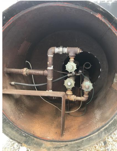
Figure 2: Three burners connected without throttle valves
