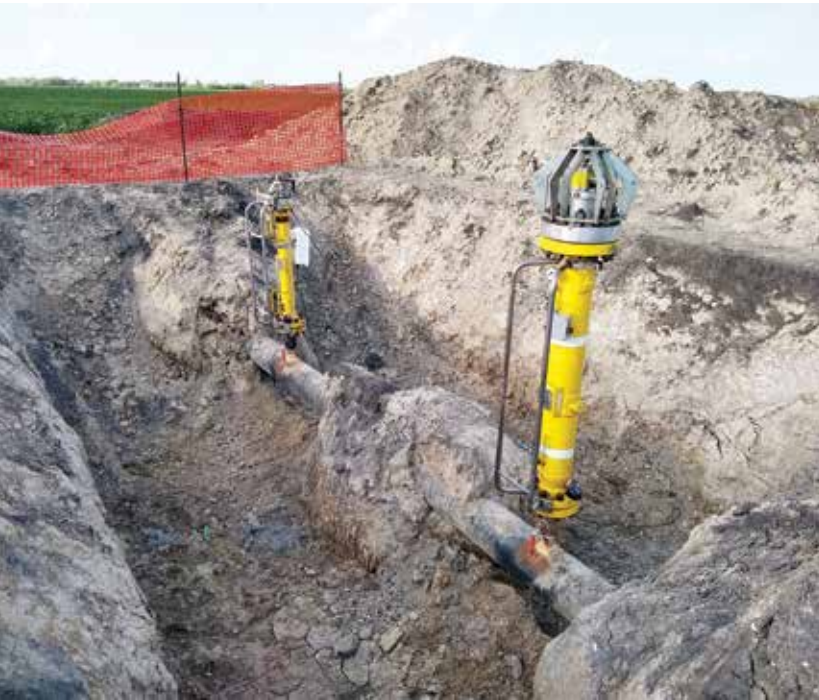
Figure 5: In-line Charge Site on 10 inch Pipeline
