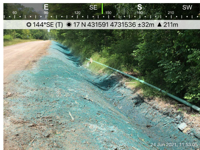
Photo 16: Mossie Line west of Watterworth Road. Hydroseeded road shoulder.
