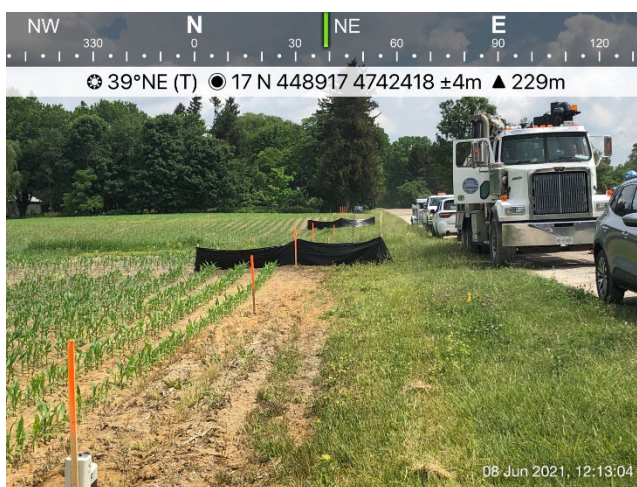
Photo 21: Silt fencing installed adjacent to Falconbridge Drive on both sides of WC80 as a precaution while conducting HDD installation of pipe.
