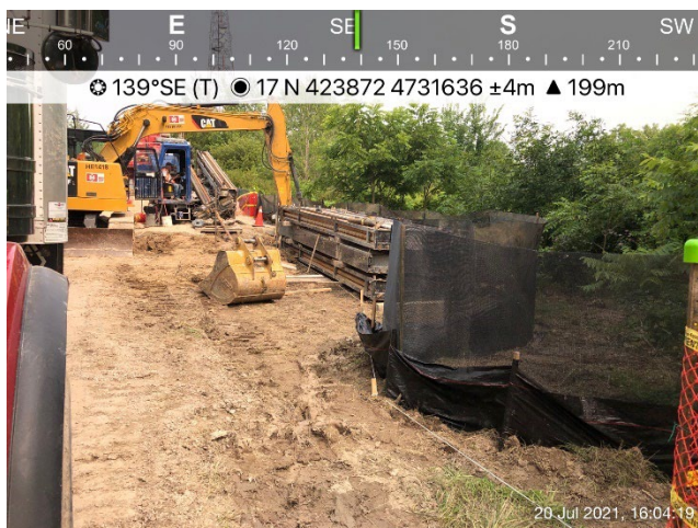
Photo 5: Sydenham River; HDD drill set up; Silt fencing & turtle exclusion fencing has been set in place.
