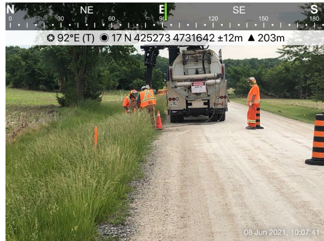
Photo 10: Hydrovacing out drilling mud from relief pit while conducting HDD along Mossie Line under Downie Road.
