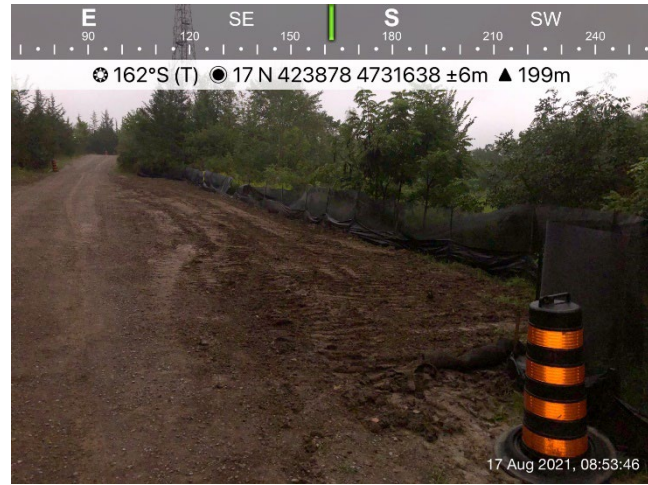
Photo 8: Sydenham River; HDD rig has been removed; Area has been graded and ready for seeding.
