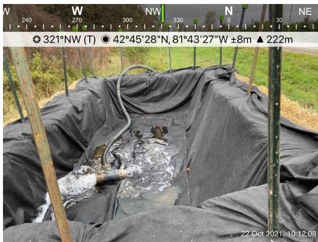
Photo 19: Dundonald Road. Hydrostatic test water that was stored at Glencoe Station is being released.
