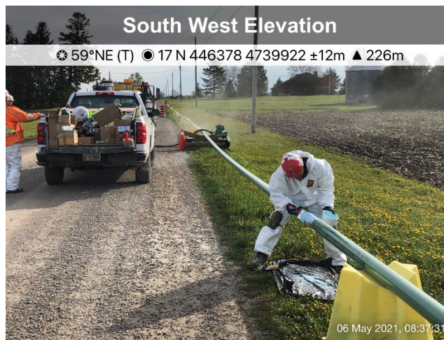
Photo 20: Sandblasting and coating welded pipe along Falconbridge Drive, east of Thames Road. Drop sheet used to collect any dripping epoxy coating.
