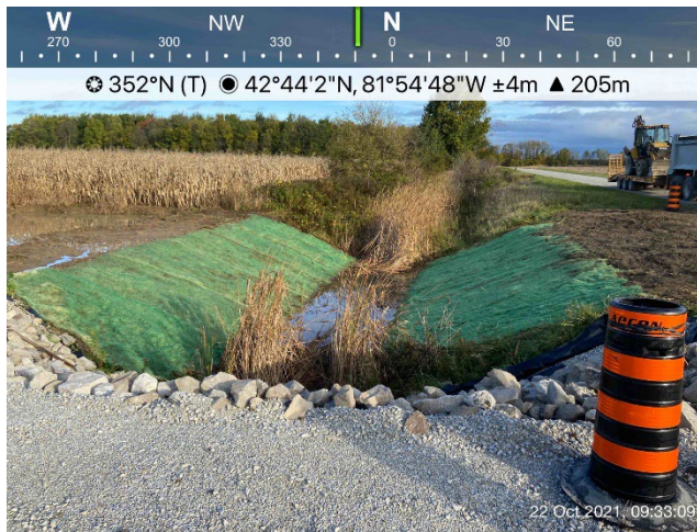
Photo 13: Downie Road Station; Location of temporary bridge has been graded, seeded and covered with erosion control blanket.
