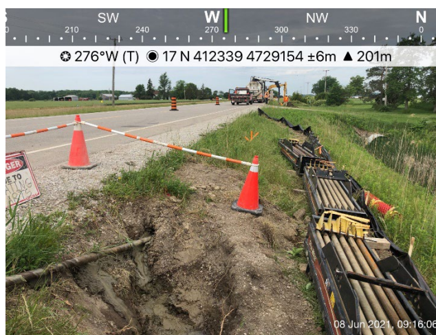
Photo 4: Silt fencing along with sump pit installed around HDD drill rig at Bentpath Line while boring under Huffs Corners Road.
