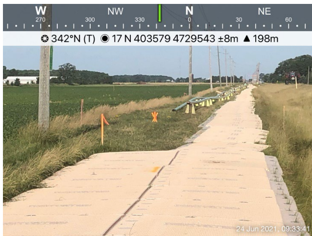
Photo 1: Rubber-polymer rig mats installed in farm field along Bentpath Line, west of Marthaville Road. Used to reduce soil compaction while installing new pipe.
