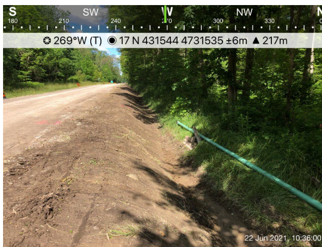
Photo 15: Mossie Line west of Watterworth Road. Reshaped road shoulder after pipe installation with Spider Plough.
