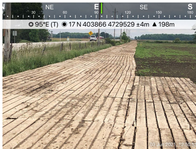
Photo 2: Wood rig mats installed in farm field along Bentpath Line, east of Marthaville Road. Used to reduce soil compaction while installing new pipe.
