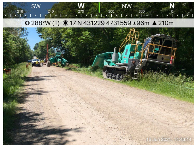
Photo 14: Installation of pipe with Spider Plough Crawler along Mossie Line west of Watterworth Road.
