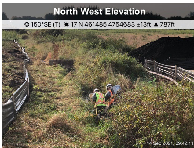
Photo 29: WC105 open cut/dam and pump; Aquatics crew conducting fish rescue near downstream metal dam.
