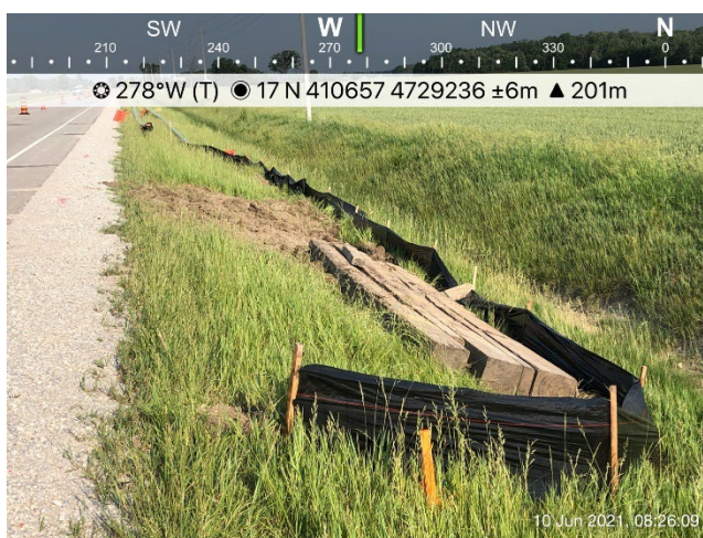
Photo 3: Silt fencing installed around HDD exit hole at Bentpath Line while boring under Gould Road.
