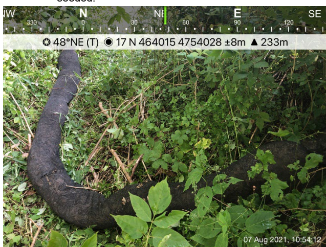
Photo 33: HDD along Glendon Dr under Crowe Creek; Silt Soxx™ on east bank of Crowe Creek.
