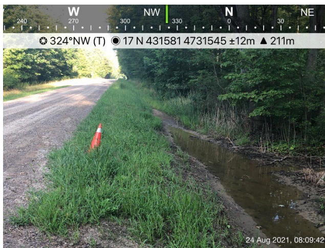
Photo 17: Mossie Line west of Watterworth Road. Vegetation on hydroseeded road shoulder is well established.
