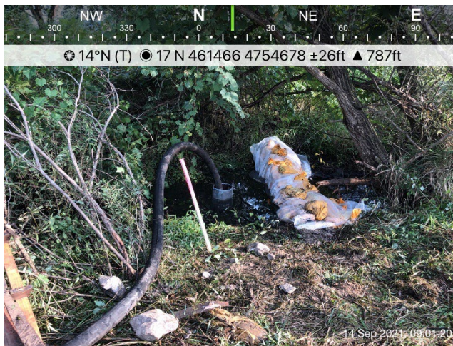
Photo 27: WC105 open cut/dam and pump; Upstream dam and pump hose with fish screen.
