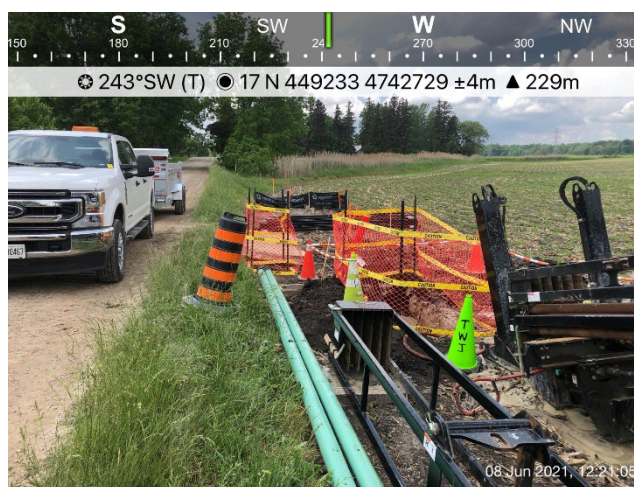
Photo 22: HDD setup while boring under WC81. Double silt fencing to capture inadvertent returns. Safety fencing around drill mud sump pit.
