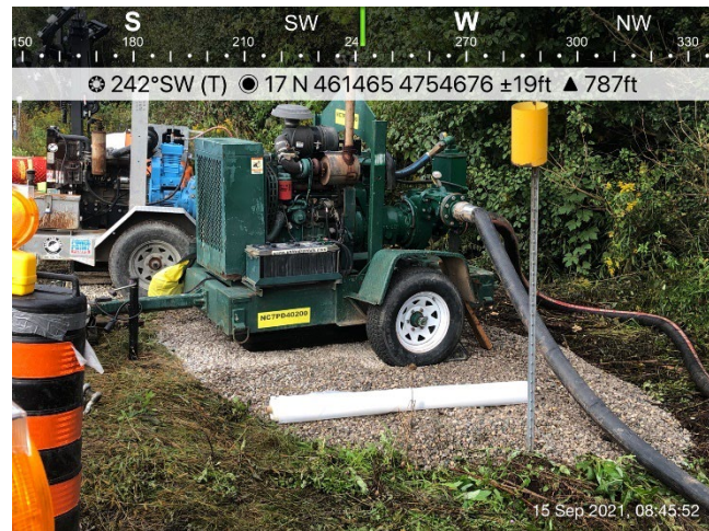
Photo 26: WC105 open cut/dam and pump; Upstream dewatering generator pump with spill tray underneath.
