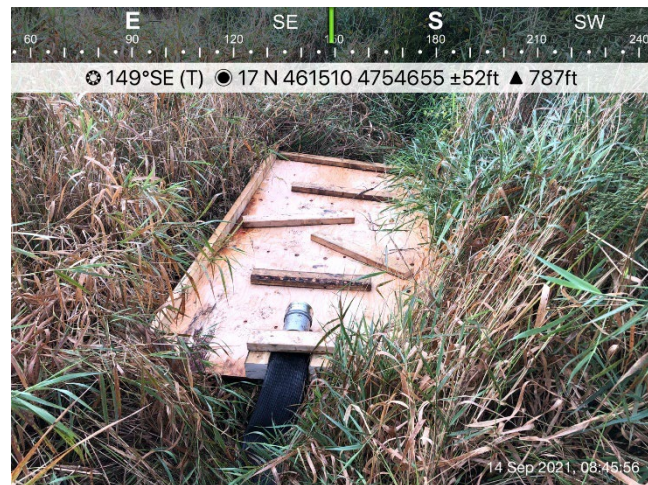
Photo 28: WC105 open cut/dam and pump; Upstream dewatering hose attached to water energy deflector in grassy area.
