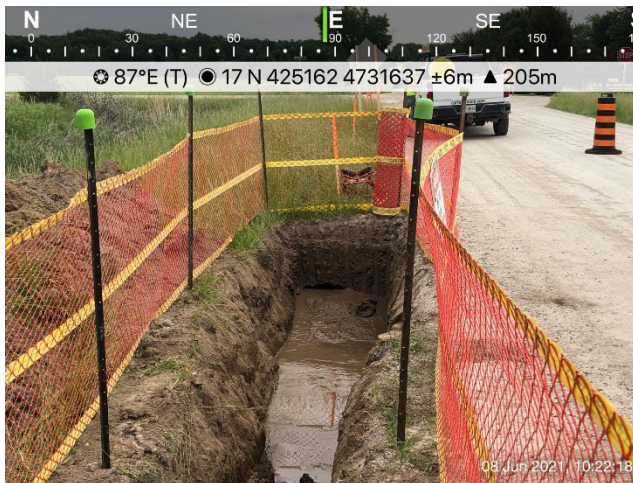
Photo 11: Safety fencing installed at HDD exit trench along Mossie Line while boring under Downie Road.
