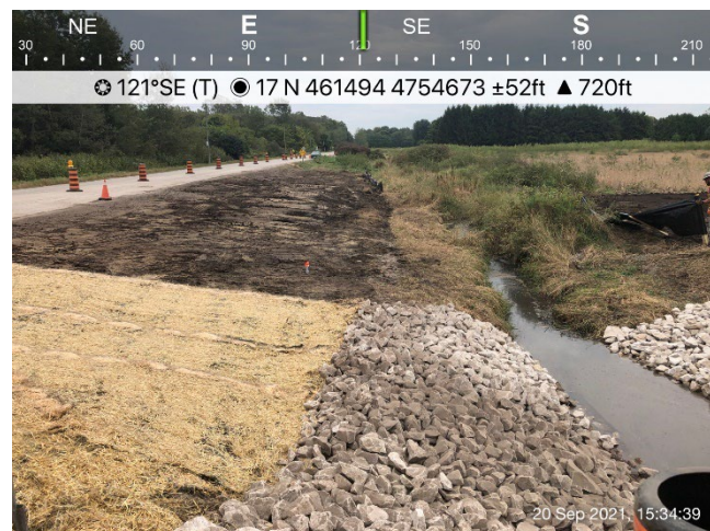
Photo 30: WC105 open cut/dam and pump; Stream channel stabilized; Excavated banks have ECB. Remainder has been seeded.
