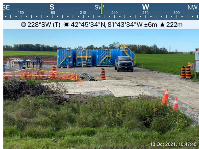
Photo 18: Glencoe Station; Hydrostatic test water being stored on frac tanks until release.
