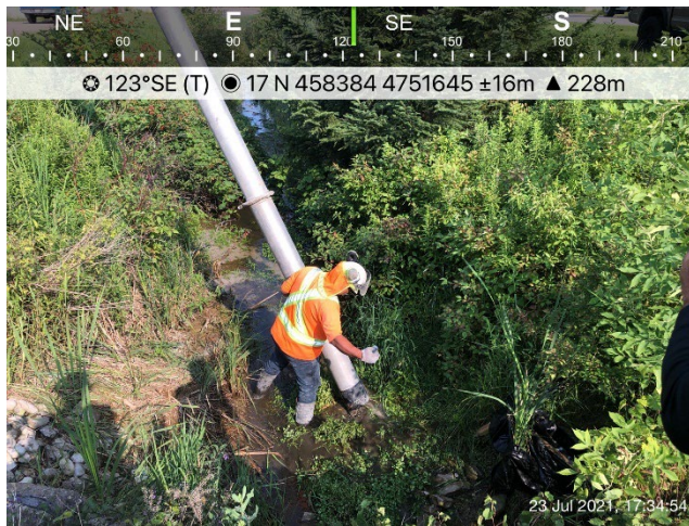
Photo 25: HDD along Falconbridge Drive under WC98. Inadvertent release being removed with hydrovac.
