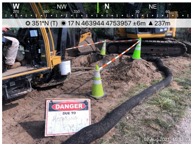
Photo 32: Crowe Creek; HDD drill set up; Silt Soxx™ has been set in place in foreground. The dark silt fencing and turtle exclusion fencing are installed behind the hoe and drill rig.
