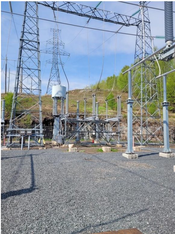
Lakehead TS – CVT installation and tower connections
