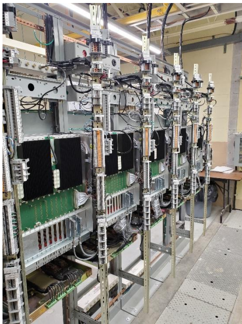
Marathon TS – back side of JMUX communications racks
