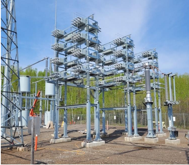
Lakehead TS – Capacitor Bank installation
