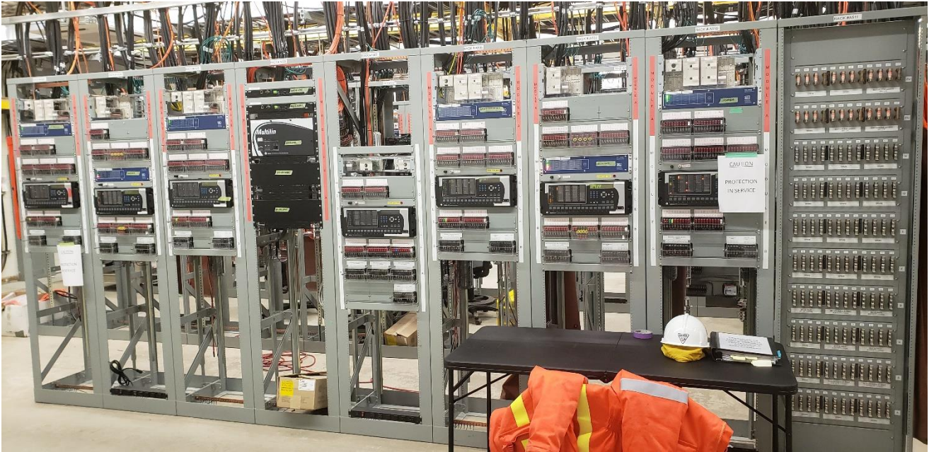
Lakehead – various protection and telecom racks – JMUX controls
