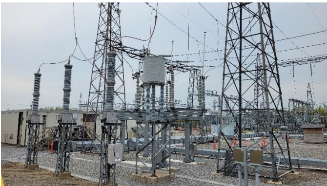
Marathon TS – switch and CVT installation
