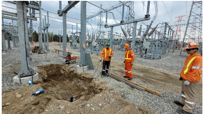
Marathon TS – grid grounding installation
