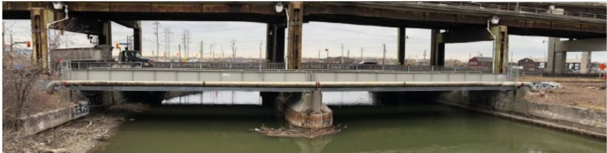
Figure 2. NPS 20 HP Steel Main Crossing the Don River
