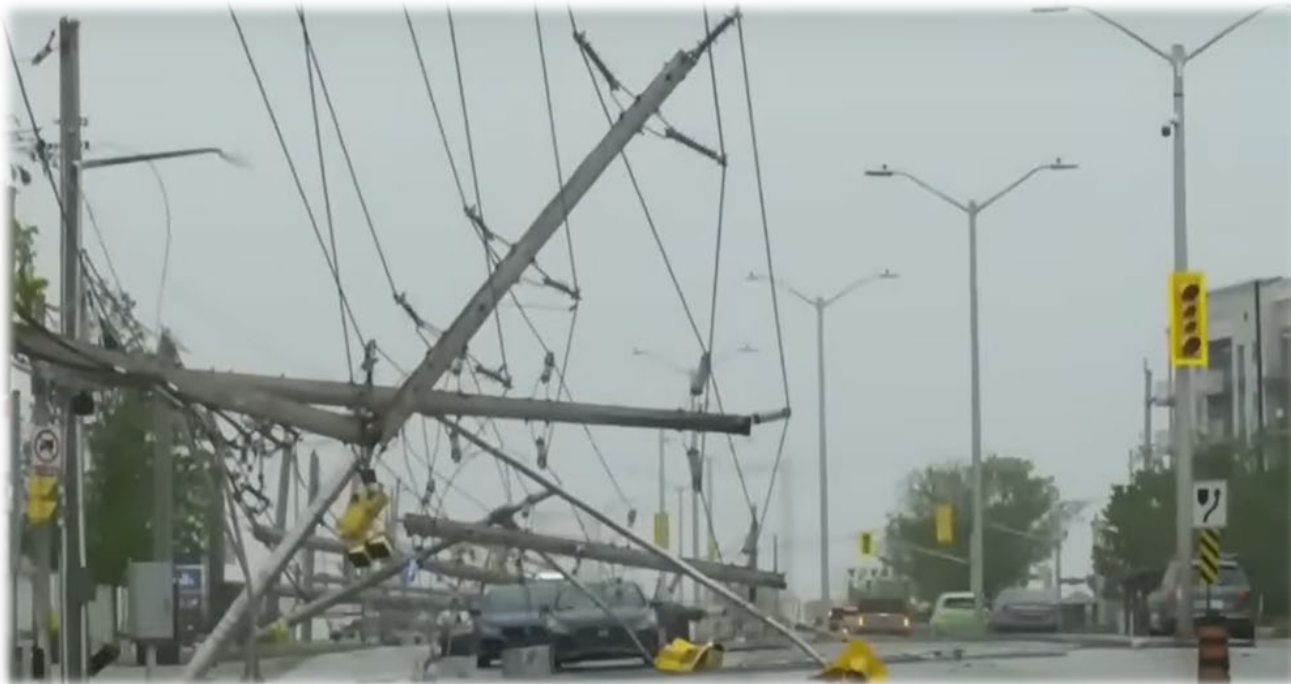
May 21, 2022 Storm – Downed Poles and Conductor Damage
