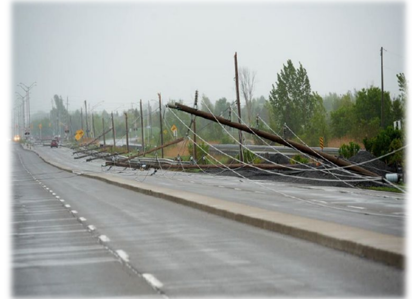
May 21, 2022 Storm – Downed Poles and Conductor Damage
