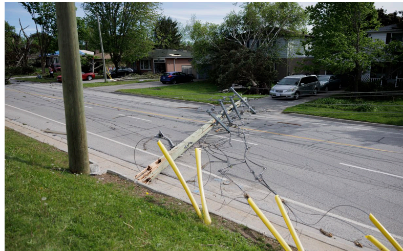
May 21, 2022 Storm – Broken Distribution Pole
