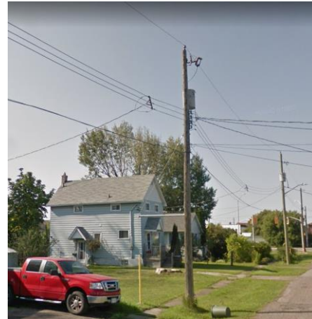
Figure 2: Typical Pole in Project
