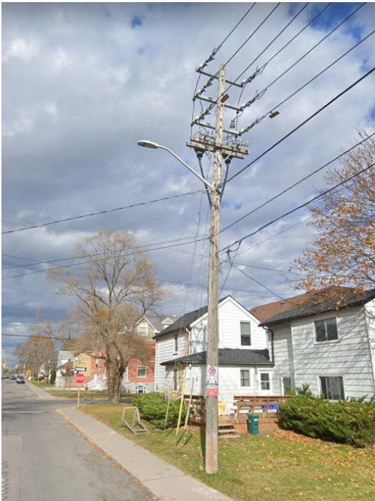
Figure 1 – Existing 203 and 206 Circuit riser pole showing legacy and non-standard construction with reduced working clearances and pole congestion
