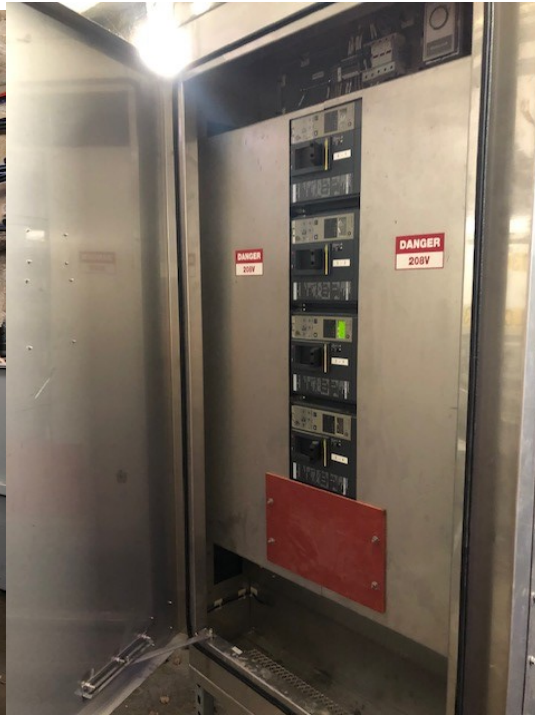
New Gas switches and Secondary Breaker
