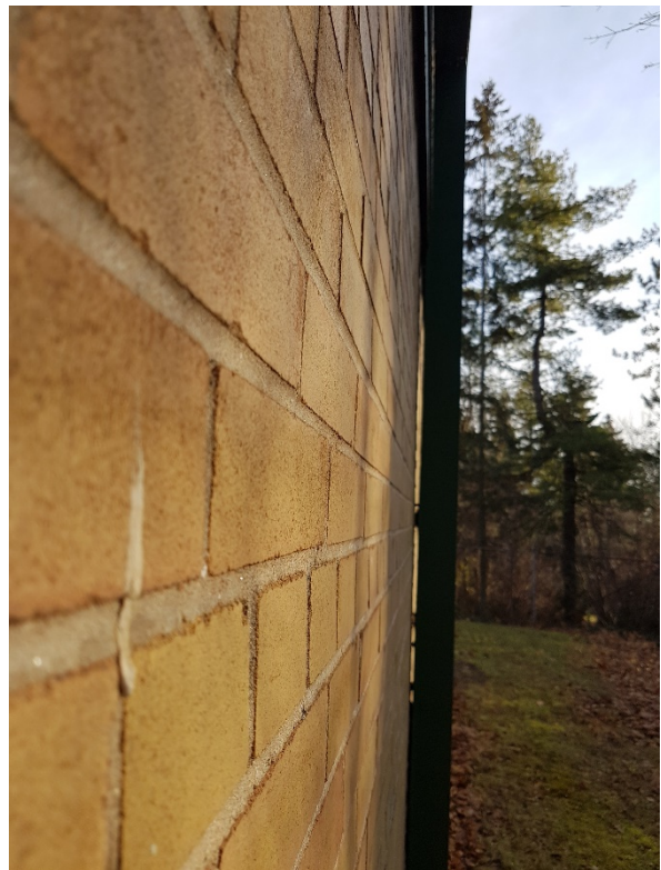
Fig. 2 – MS6 – Masonry Walls and Structural Steel Frame Shifted (Laterally Displaced)
