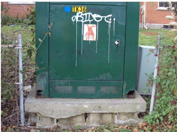
Figure 2: Rusty Enclosure & Deteriorated Foundation at TK36
