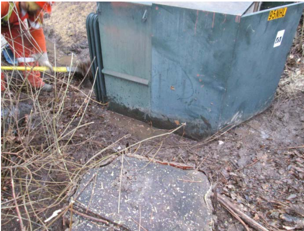
Figure 1: Flooded Pad Transformer at 95 Notch Hill Rd.
