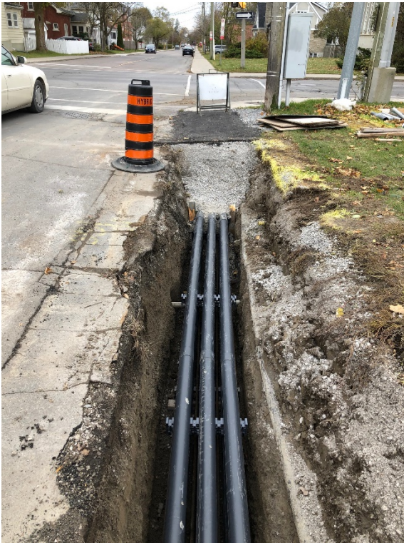
104 Figure 3 & Figure 4 – New 207 circuit ducts, future use 201 and 208 circuit ducts installed on MacDonnell Street
