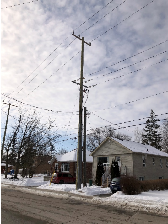
101 Figure 2 – New 207 Circuit riser constructed to modern standards and increased clearances, note additional space 102 on poles for future 201 and 208 circuit extensions
