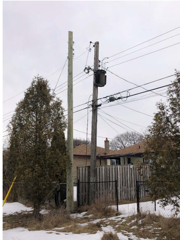
Figure 1 & 2 – Existing poles showing legacy construction standards, limited working space and poor pole conditions
