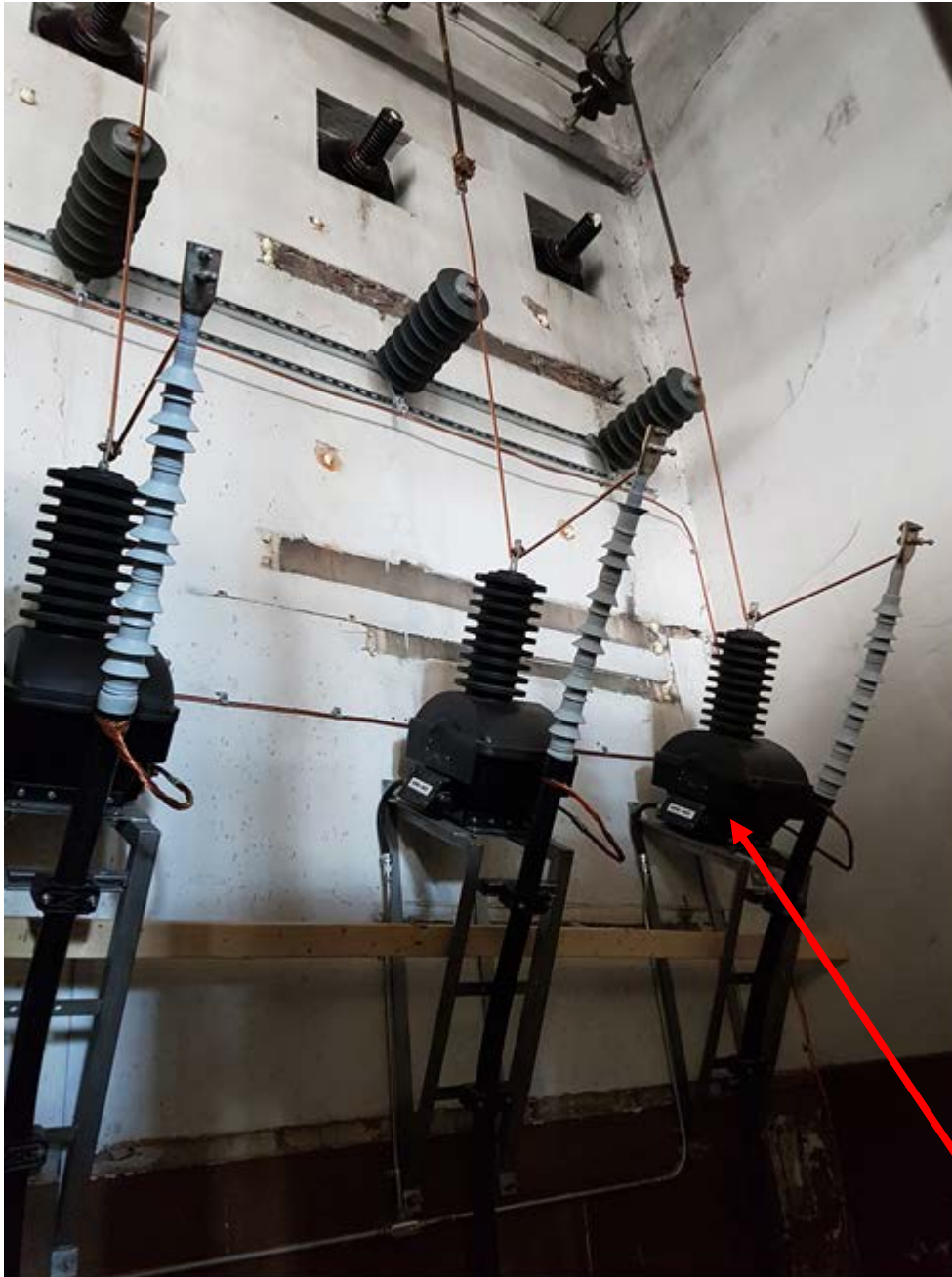
Interior View of North Wall After 44kV Cable Riser Relocation & New Instrument Transformer Installation
