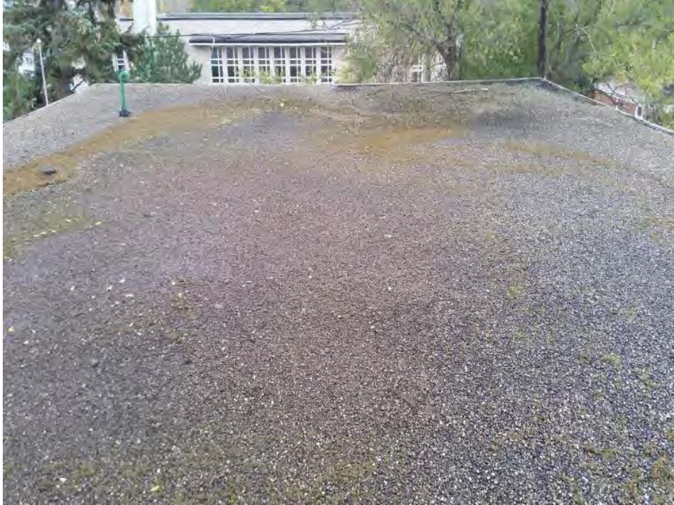
Fig. 2 – MS2 – View of existing deteriorated higher roof
