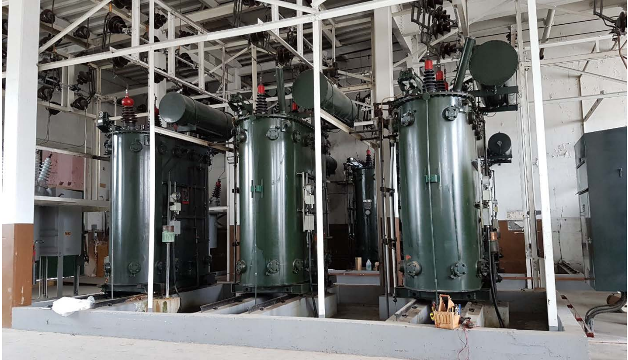
Existing Water-Cooling Transformers T1, T2 and T3
