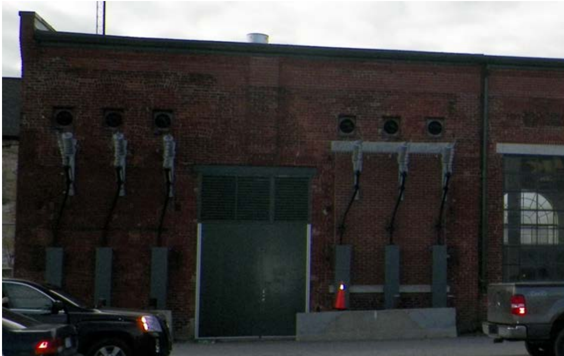
Exterior View of North Wall Before Relocating 44kV Cable Risers
