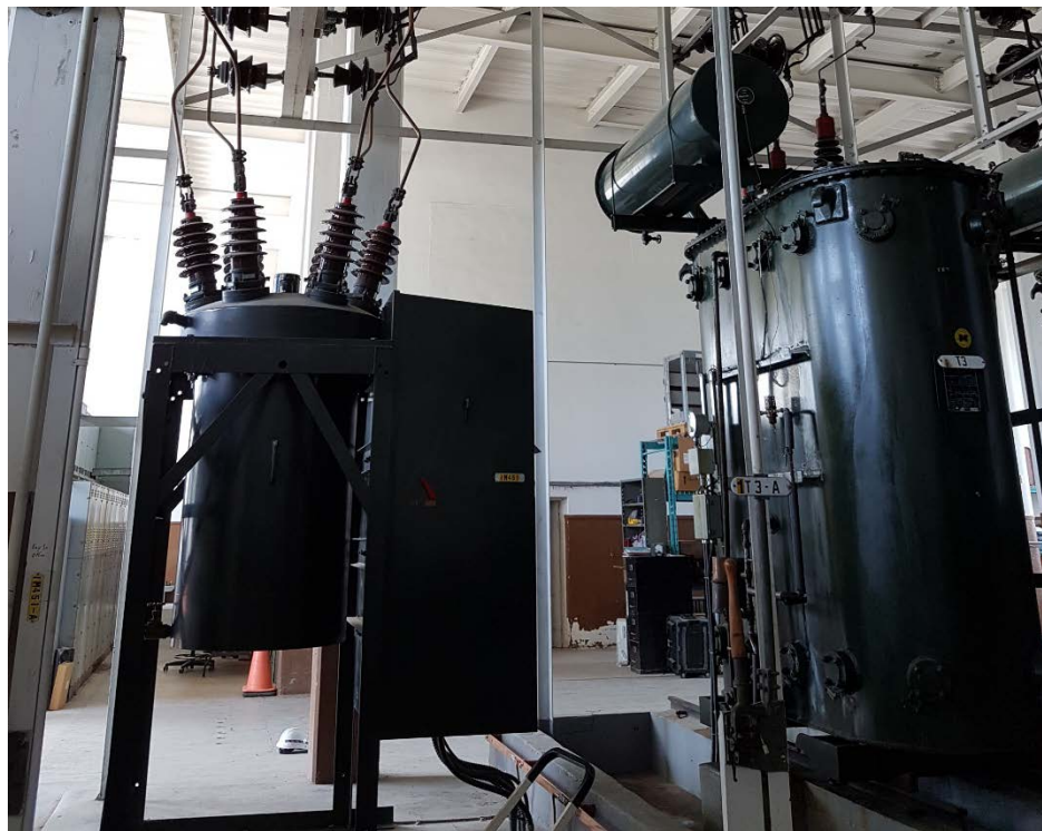
Existing 44kV Oil Circuit Breaker
