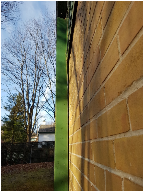
Fig. 2 – MS6 – Masonry Walls and Structural Steel Frame Shifted (Laterally Displaced)
