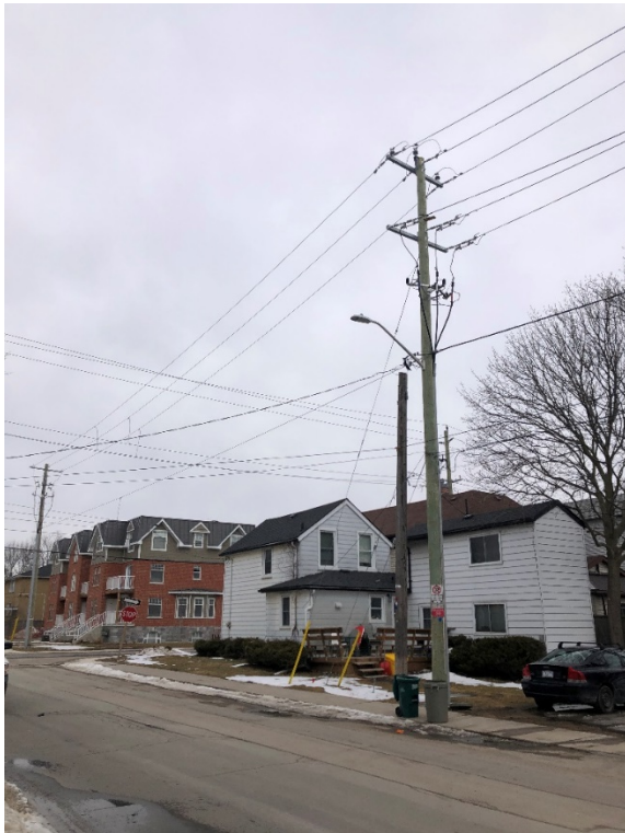
106 Figure 3 – New 206 Circuit riser pole constructed to modern standards and increased clearances
