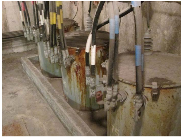
Figure 5: Leaking Vault Transformers at 2 Bay St.
