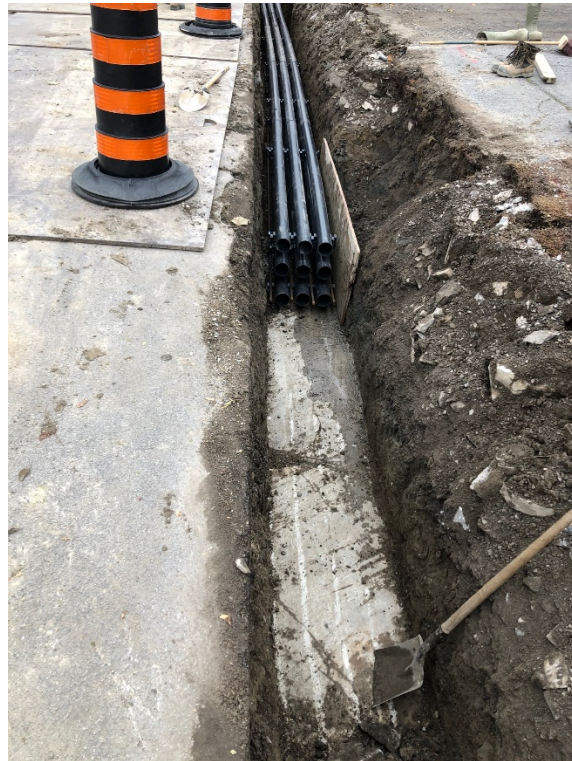
104 Figure 3 & Figure 4 – New 207 circuit ducts, future use 201 and 208 circuit ducts installed on MacDonnell Street
