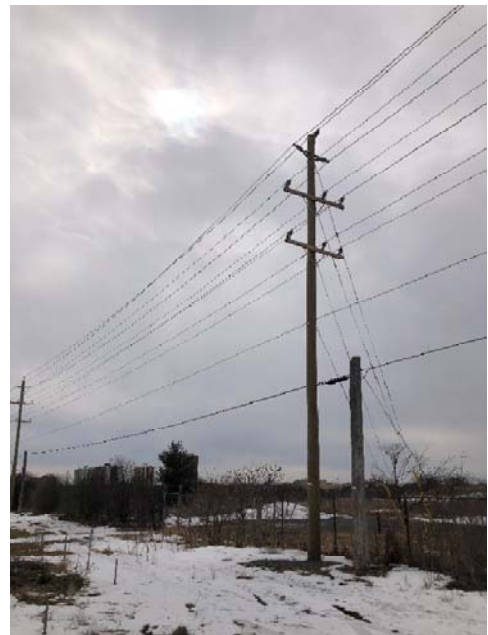
Figure 3 & 4 – New poles constructed to modern standards and improved clearances.
