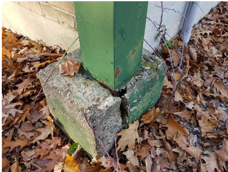
Fig. 5 – MS6 – Cracked Footing for Steel Column
