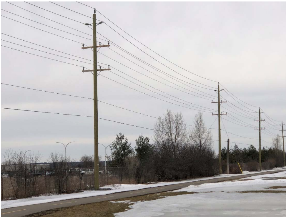
Figure 1 – New poles installed along the Leroy Grant Drive Trail with new 13.8kV circuit installed
