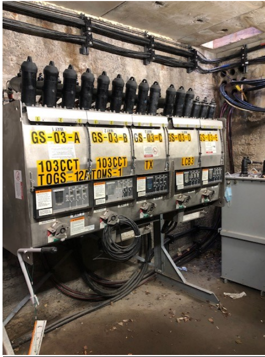
New Gas switches and Secondary Breaker
