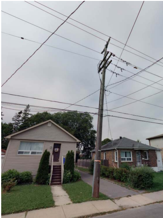
Figure 1 – Existing 207 Circuit riser pole showing legacy and non-standard construction with reduced working clearances
