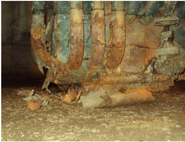
Figure 4: Rusted Vault Transformer at 180 Queen Mary Rd.
