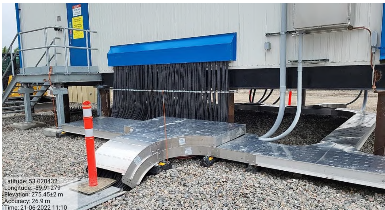
Photo 20: Substation J – Kingfisher cable entrance to Control Building
