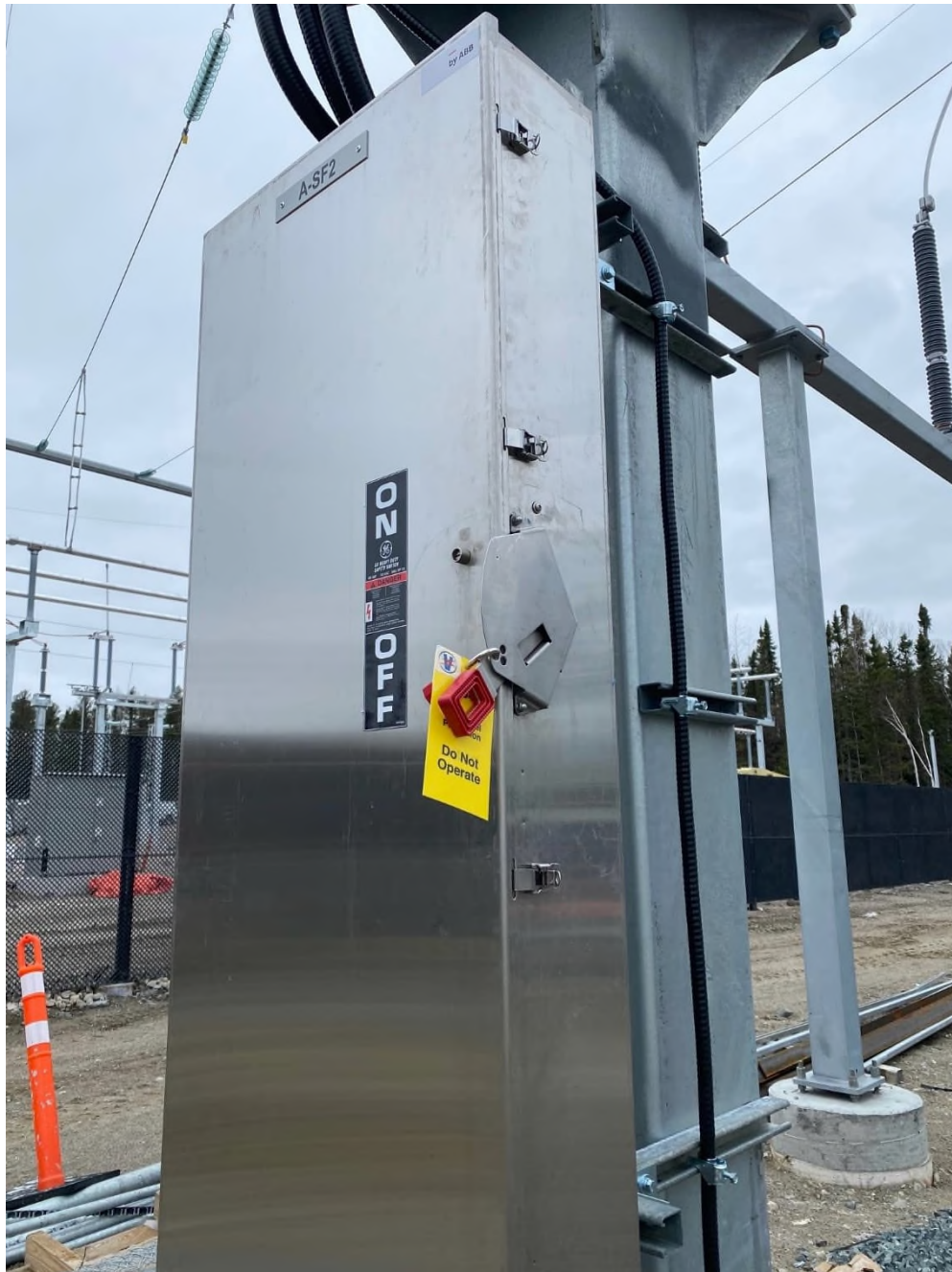
Photo 5: Substation A SSVT panel locked and tagged
