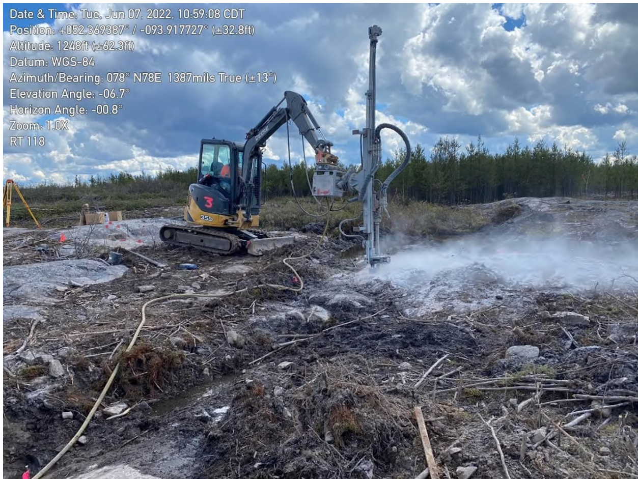
Photo 5: RT-0118 drilling foundations
