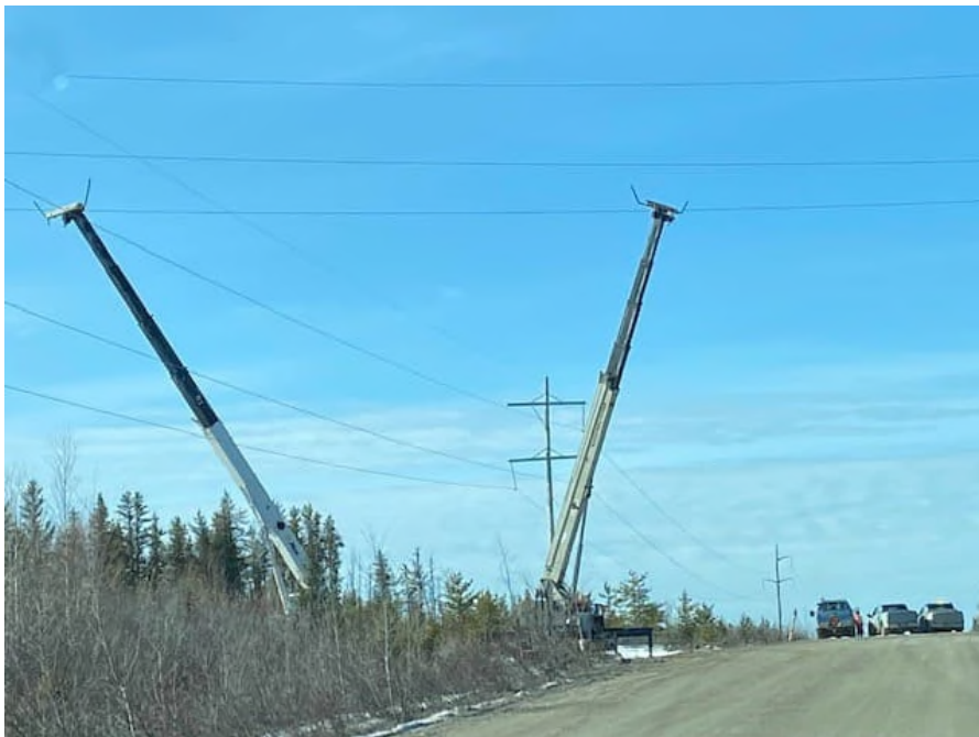
Photo 2: Cranes used when crossing existing lines
