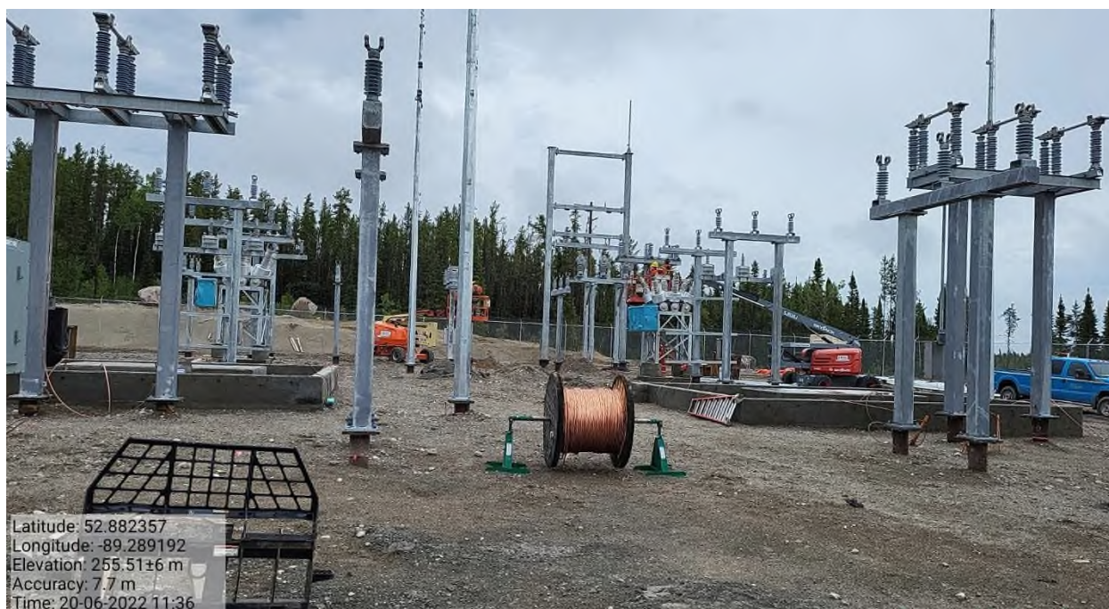
Photo 18: Substation I – Wunnumin Steel structures and insulators
