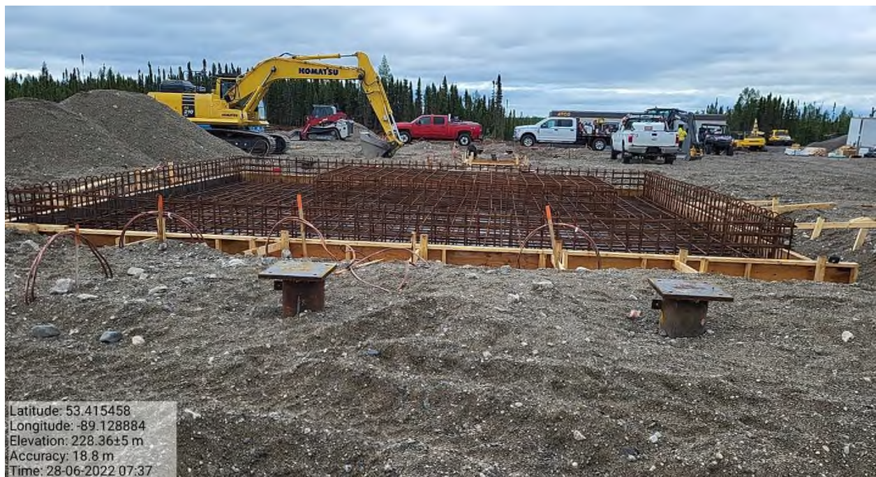
Photo 21: Substation K – transformer containment rebar
