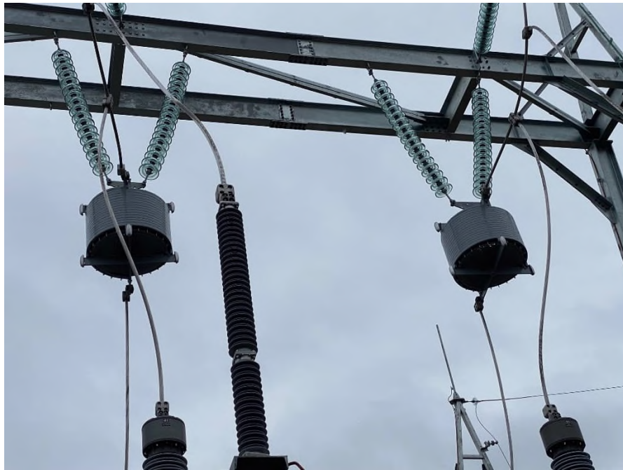
Photo 1: Substation A Air traps Sub A
