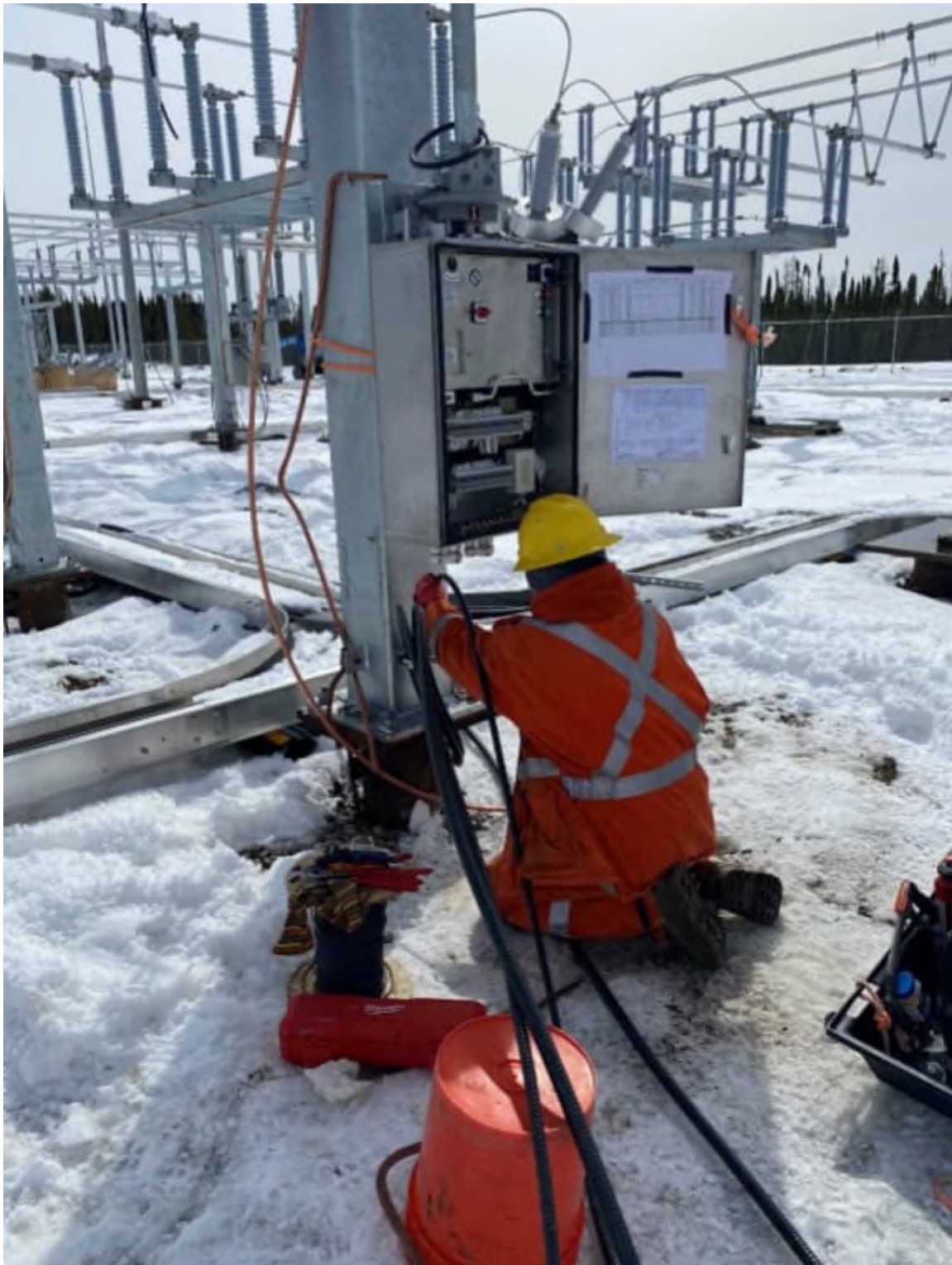
Photo 8: Crew glanding control cables at Sub J
