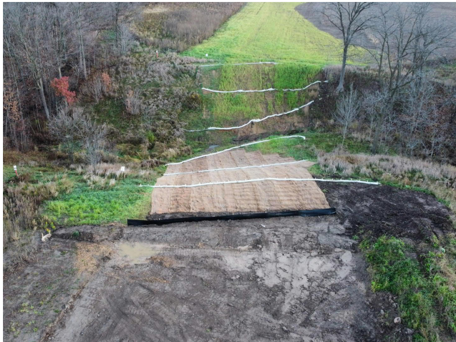
Photo 8: Open-cut watercourse crossing (WC_9.1), restored after construction, view facing northeast.
