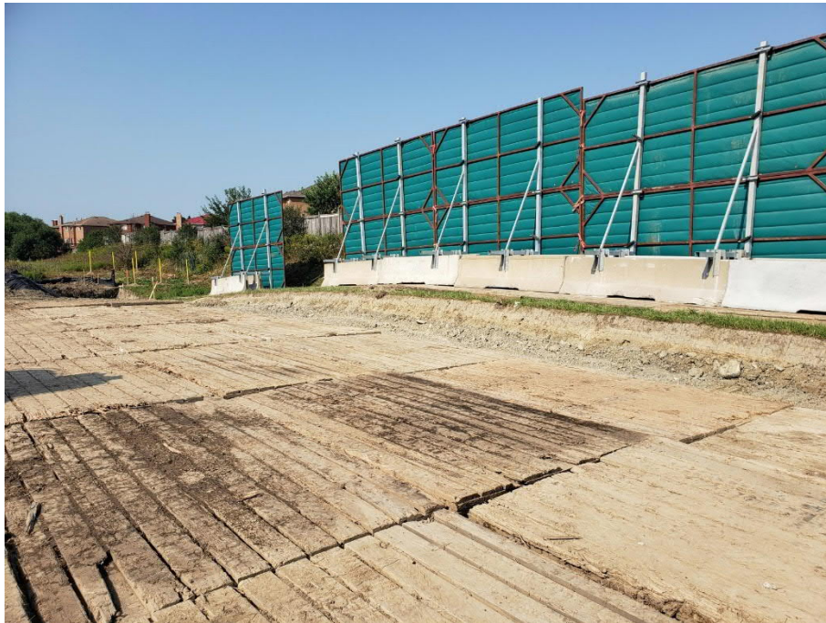
Photo 14: Engineered sound wall installed at the Mavis Road HDD.
