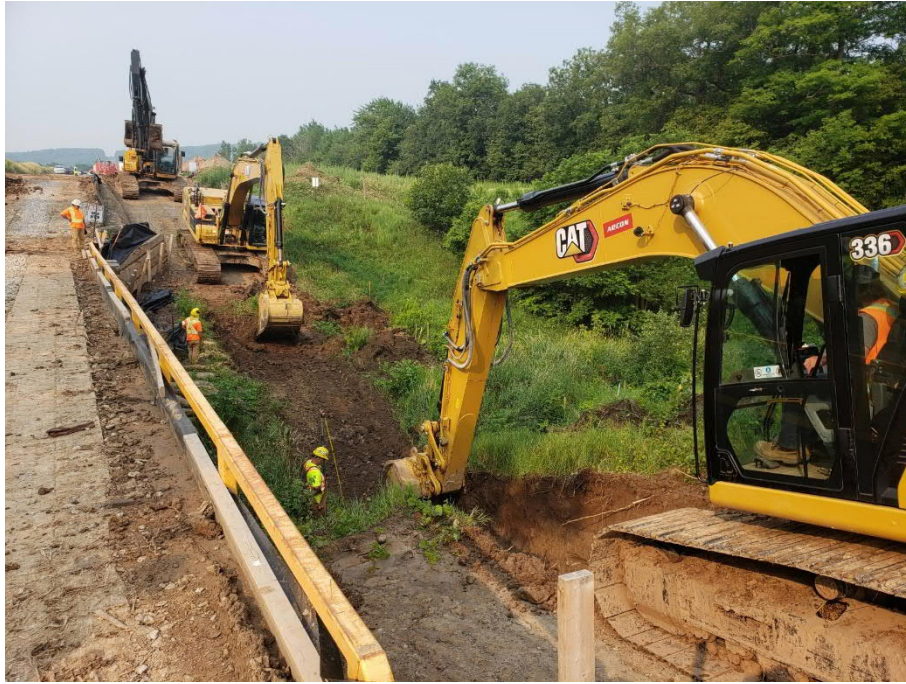
Photo 7: Open-cut watercourse crossing (WC_9.1), excavation during construction, view facing northeast.
