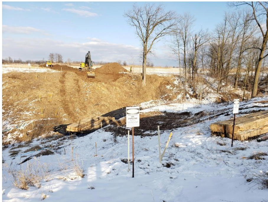
Photo 6: Open-cut watercourse crossing (WC_9.1), pre-construction, view facing east.
