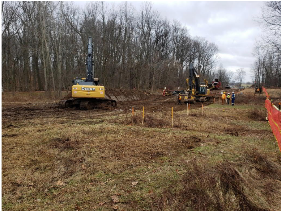
Photo 2: Topsoil stripping activities at KP 0+150, view facing southwest.
