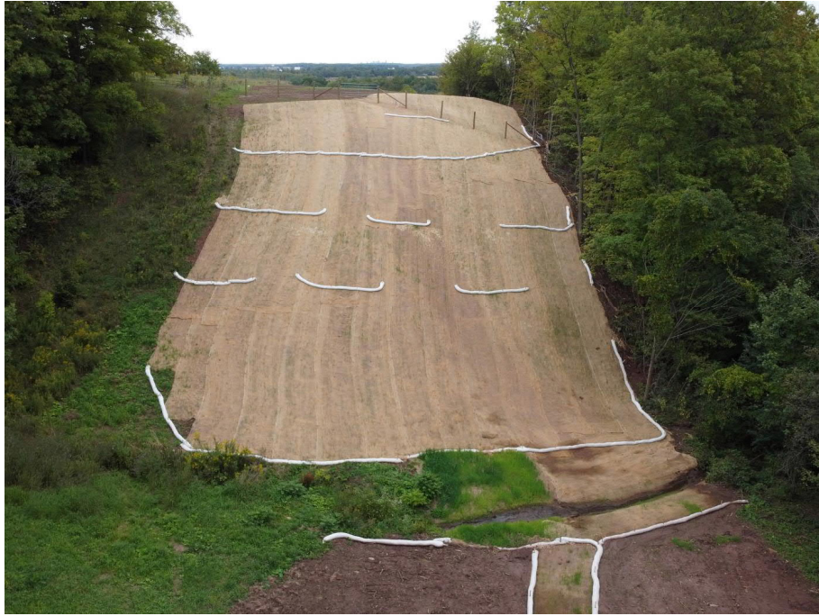
Photo 1: Steep slope restoration at KP 10+530, view facing northeast.
