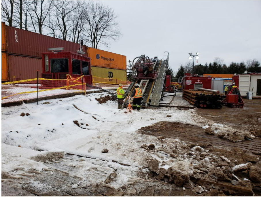
Photo 13: Sound wall constructed of sea cans at the Robson Road HDD.
