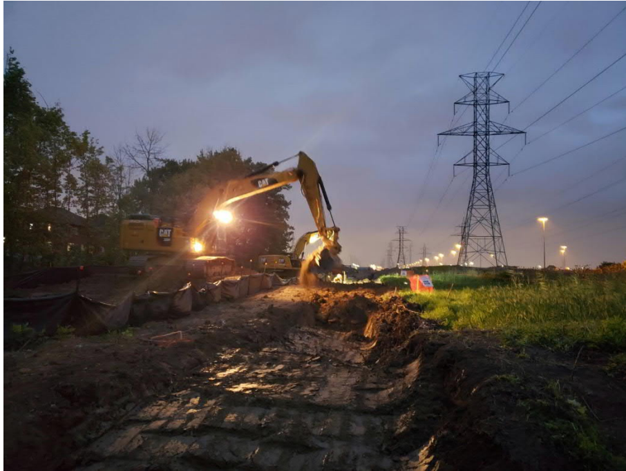
Photo 3: Wetland crossing during backfilling (WT_8.1), view facing northeast.
