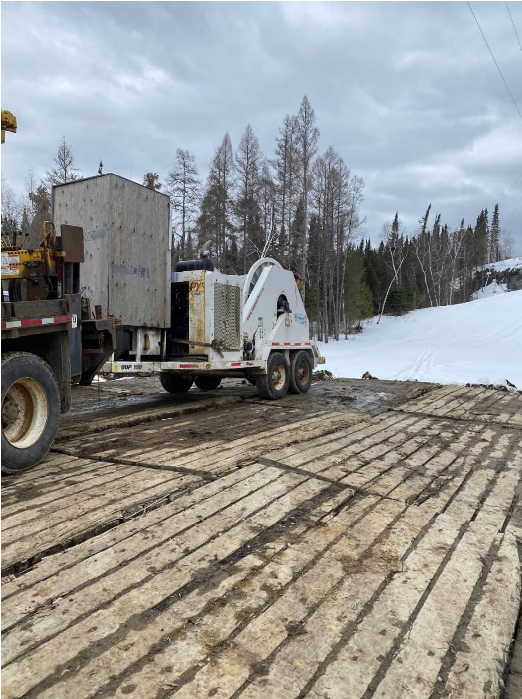
Photo 3: Puller set up at AB-024
