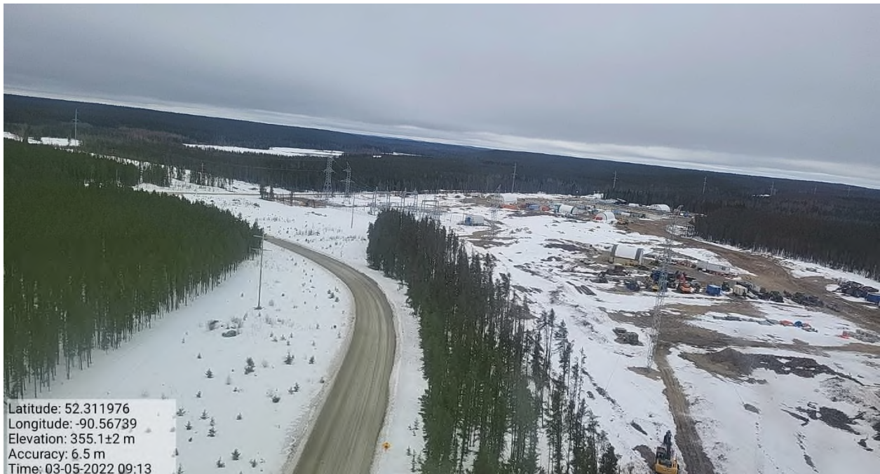
Photo 8: Substation C and CD and BC lines
