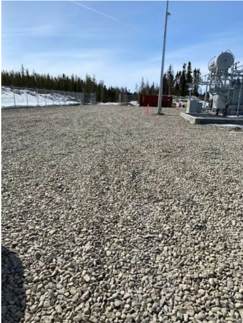
Photo 7: Insulating stone installed at Sub D North Caribou
