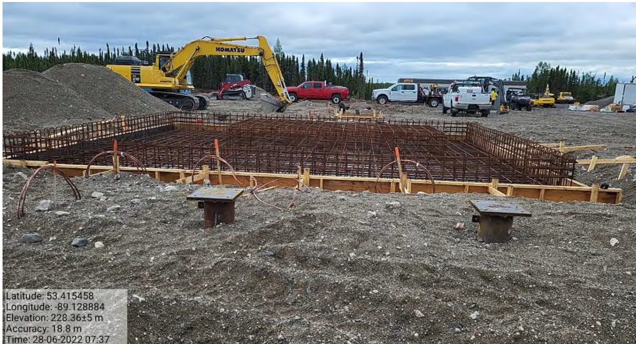
Photo 21: Substation K – transformer containment rebar
