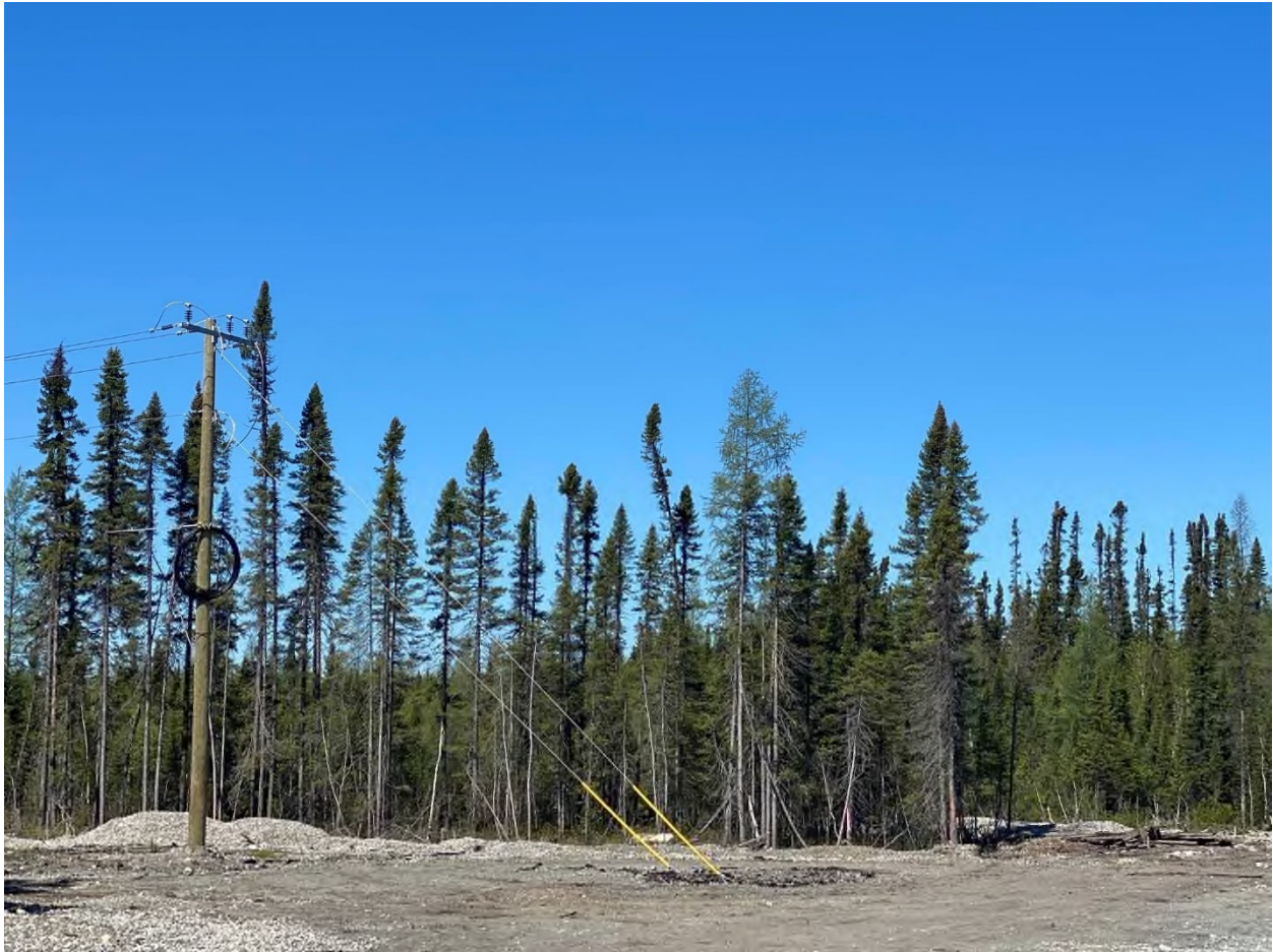
Photo 2: D1 - 25kV Substation D
