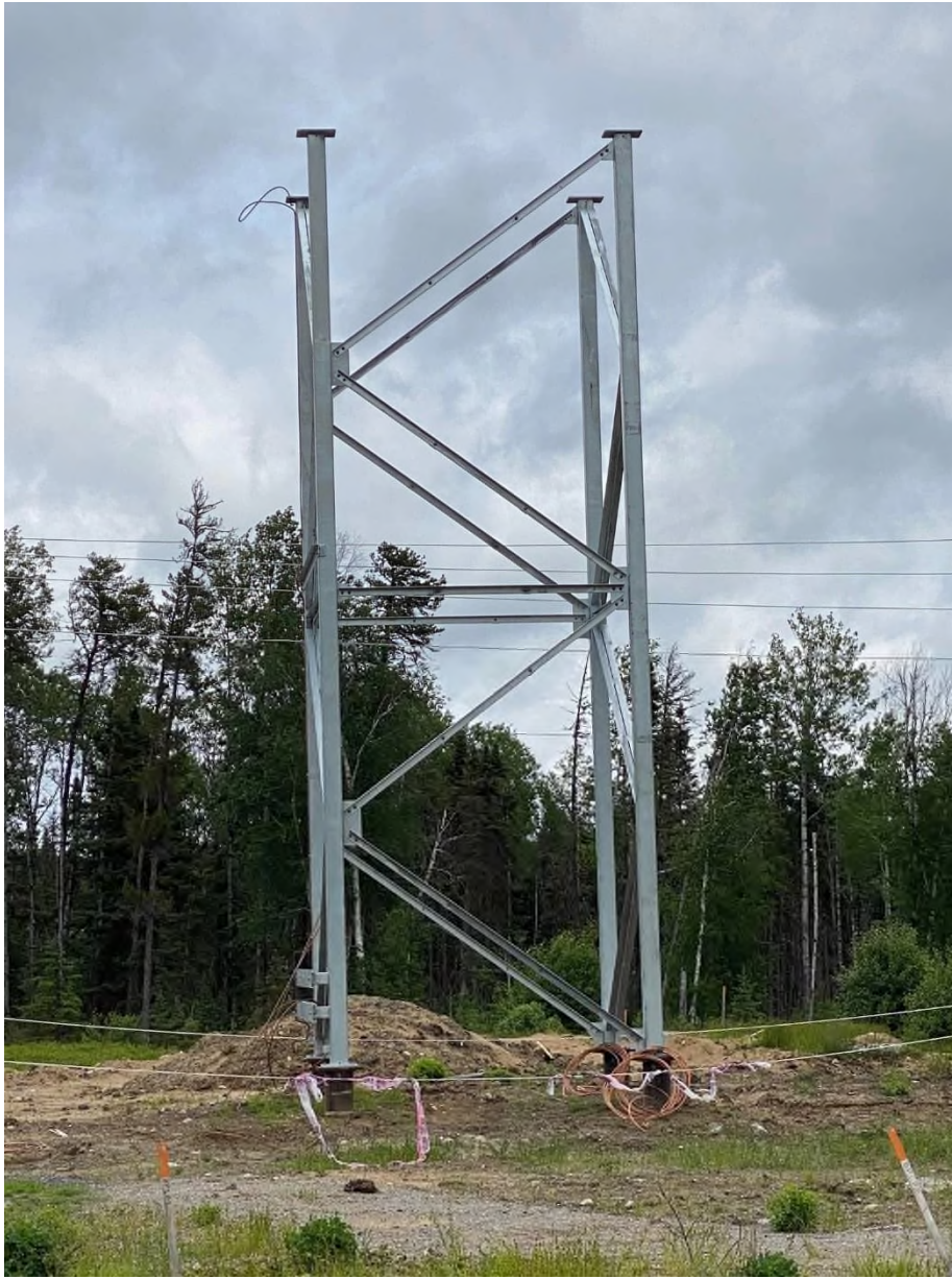
Photo 14: Substation Q – new structure
