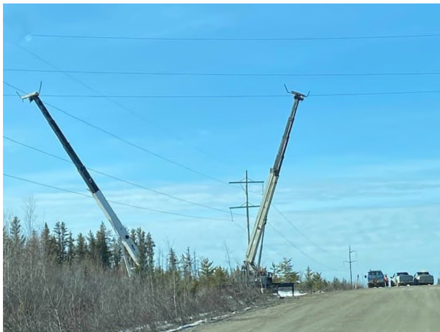
Photo 2: Cranes used when crossing existing lines
