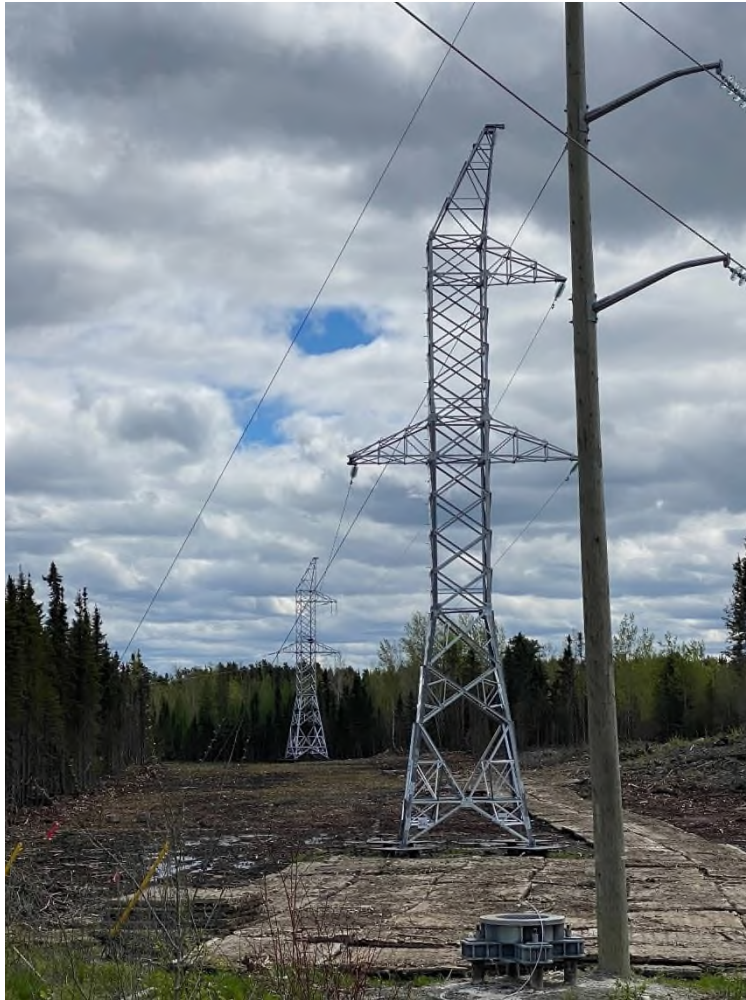
Photo 1: PQ-60 – mats laid for monopole erection
