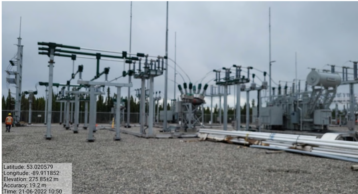
Photo 19: Substation J – 44kV station equipment complete
