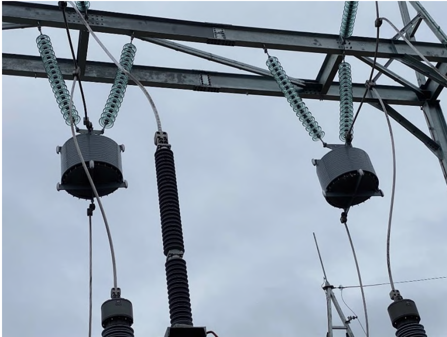
Photo 1: Substation A Air traps Sub A
