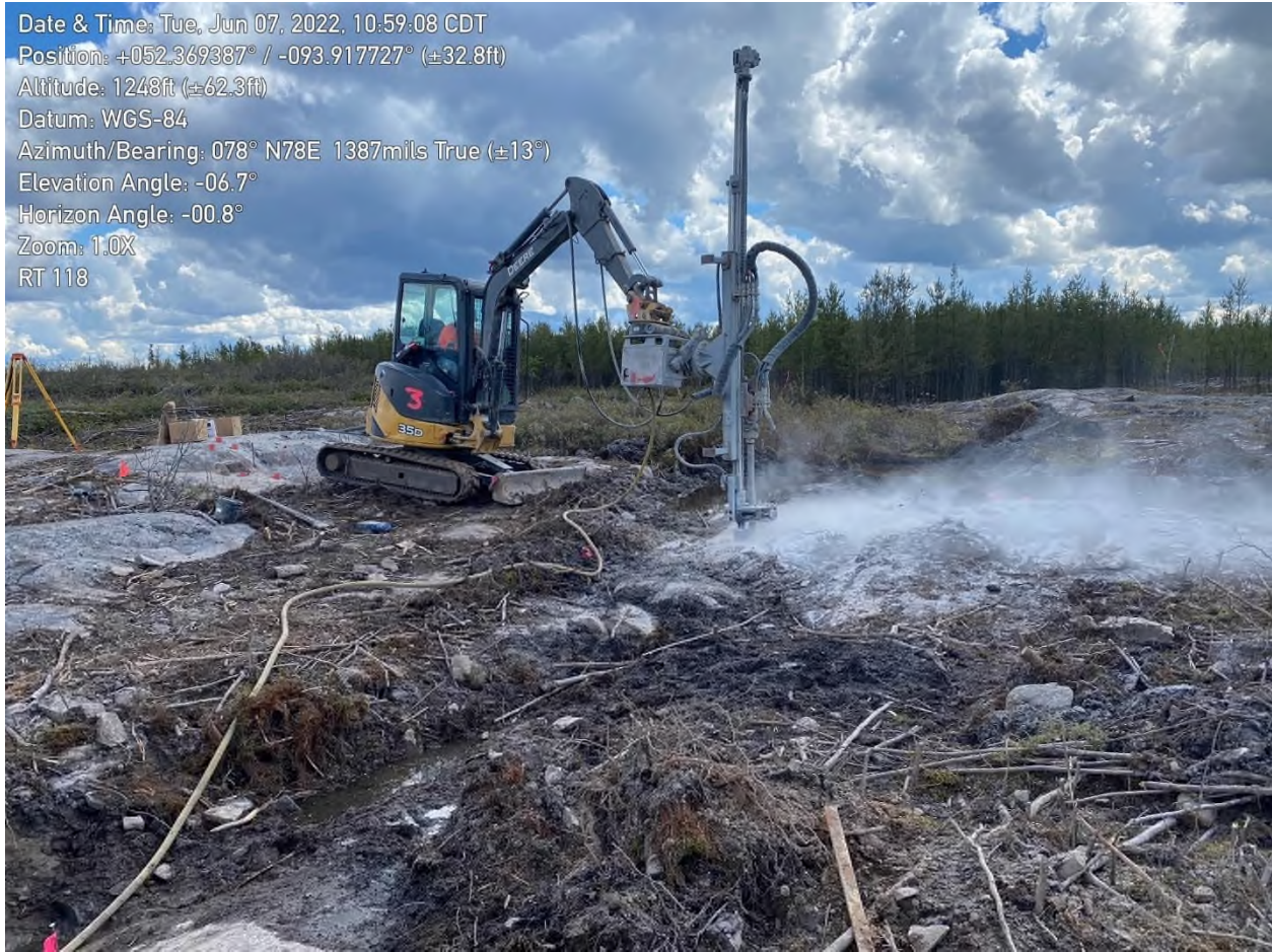
Photo 5: RT-0118 drilling foundations
