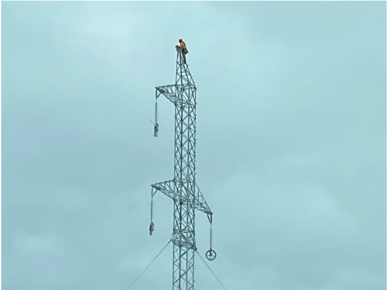
Photo 6: CJ Stringing – Crew to be picked up by helicopter
