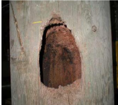
Figure 15: Woodpecker Damage
