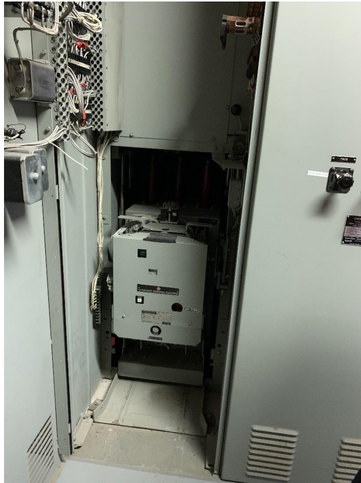
Figure 10: Metalclad Breaker at Peterborough Erskine DS
