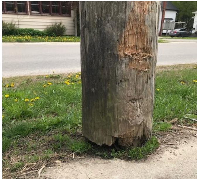
Figure 16: Ground Line Surface Rot
