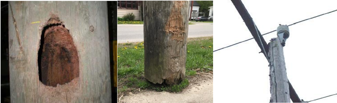
Figure 1: Examples of Poor-Condition Poles
