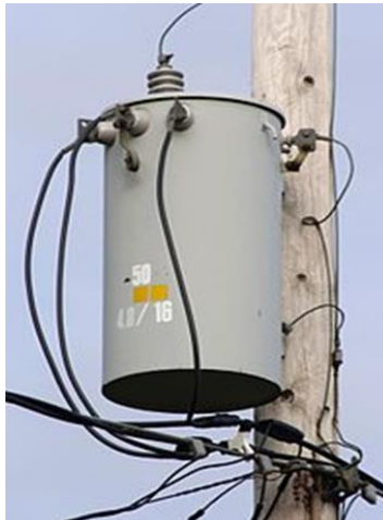
Figure 21: Picture of a Pole-Top Line Transformer
