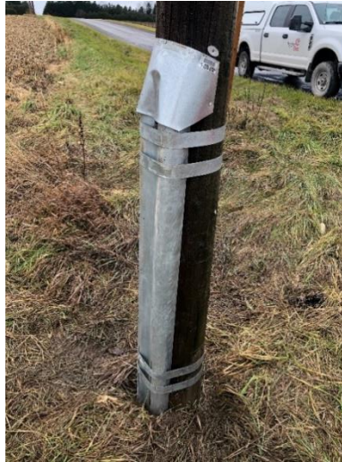
Figure 20: Mechanically Refurbished Pole
