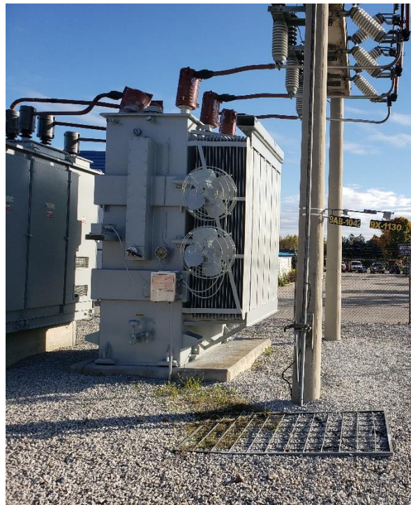
Figure 5: 7.5/10 MVA, 44-13.8 kV Station Transformer at Orillia James DS
