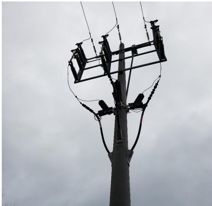
Figure 11: Orillia Jarvis DS Switch and Fuse Combination
