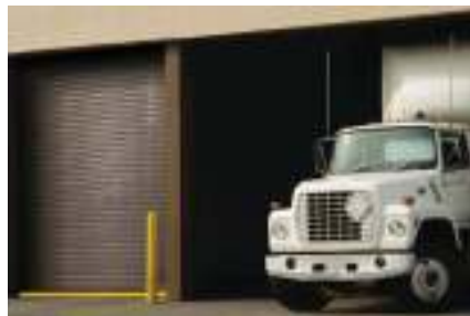
Figure 2 Example of "Drive-in" Shipping and Receiving doors 2
