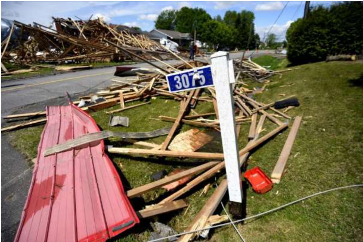
The remains of the roof of a hardware store that lifted off and crashed into neighbouring houses during a major storm is seen spread across residences in the community of Hammond in Clarence-Rockland, Ont., Monday, May 23, 2022. THE CANADIAN PRESS/Justin Tang Justin Tang.
