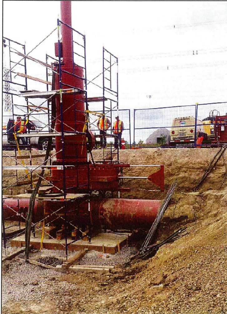
Figure 1: Stopple Fitting
