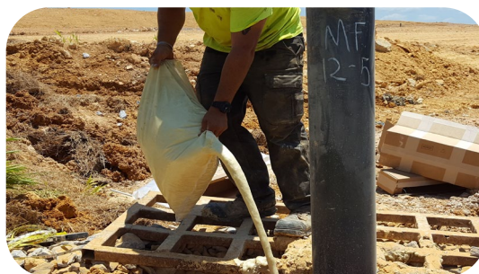
Pouring foam around a well casing
