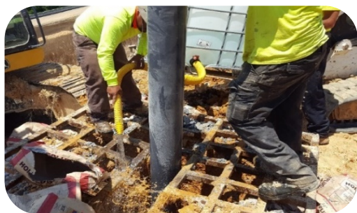
Hydrating bentonite to seal a well
