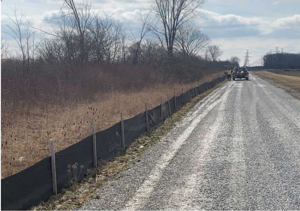
Photo 1: Exclusion fence in good condition throughout construction activities.
