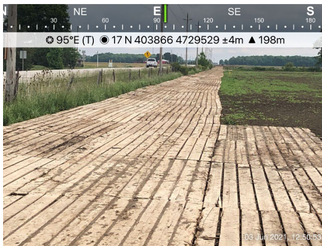
Photo 3: Wood rig mats installed in farm field along Bentpath Line, east of Marthaville Road. Used to reduce soil compaction while installing new pipe.
