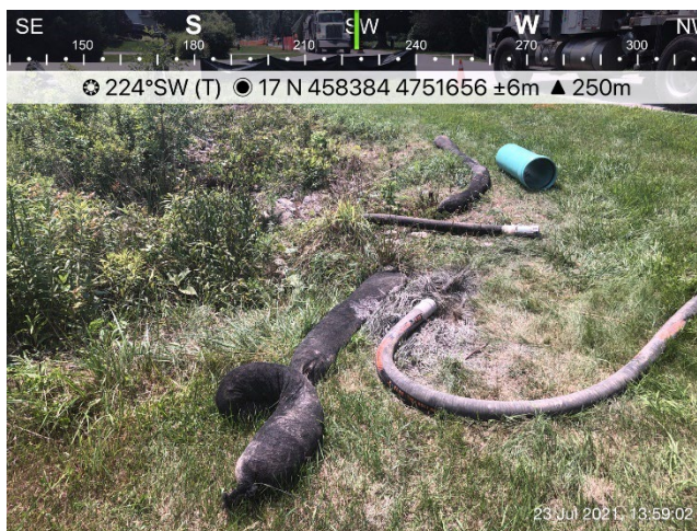
Photo 33: HDD along Falconbridge Drive under WC98 just east of Adelaide Road. Inadvertent release occurred in cobbly road culvert fill. Silt Soxx™ used to contain spill.
