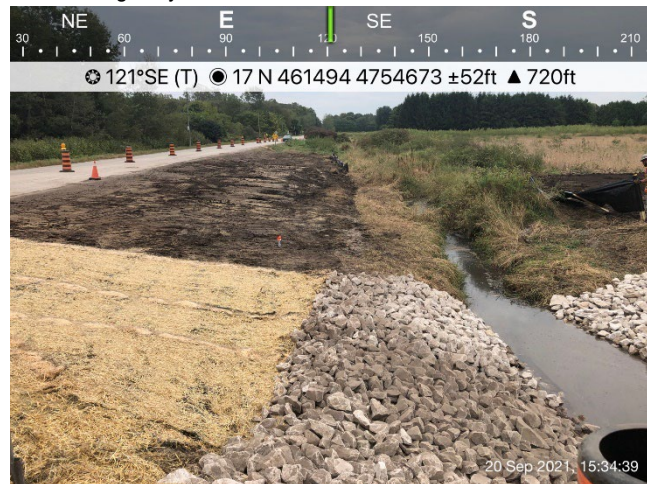
Photo 40: WC105 open cut/dam and pump; Stream channel stabilized; Excavated banks have ECB. Remainder has been seeded. View of Amiens Road
