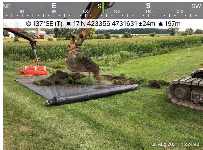
Photo 8: Sydenham River; HDD bore exit location. Hoe excavating exit pit.
