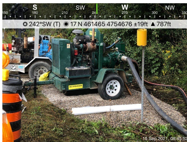
Photo 36: WC105 open cut/dam and pump at Avro Drive and Amiens Road. Upstream dewatering generator pump with spill tray underneath.
