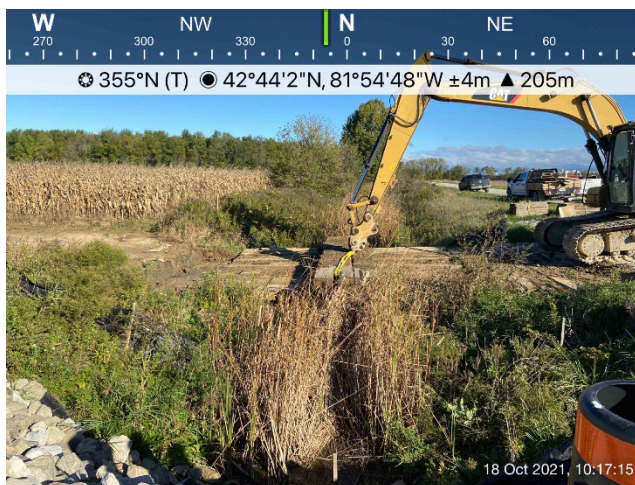
Photo 17: Downie Road Station; Temporary swamp mat bridge is being removed.
