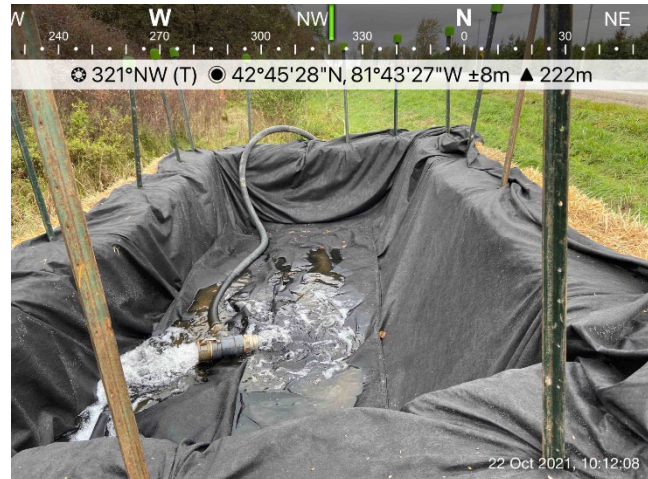
Photo 26: Dundonald Road. Hydrostatic test water that was stored at Glencoe Station is being released.
