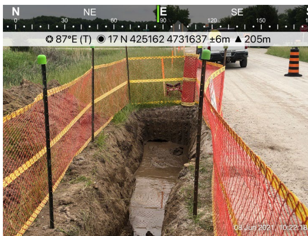
Photo 15: Safety fencing installed at HDD exit trench along Mossie Line while boring under Downie Road.
