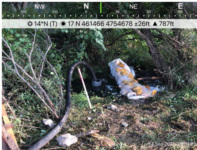
Photo 37: WC105 open cut/dam and pump; Upstream dam and pump hose with fish screen.
