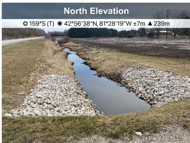
Photo 4141: Location of WC105 open cut/dam and pump; Stream channel stabilized; Vegetation growing well two seasons after construction. View of Amiens Road.
