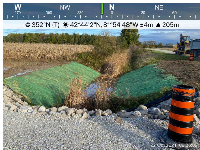
Photo 18: Downie Road Station; Location of temporary bridge has been graded, seeded and covered with erosion control blanket.
