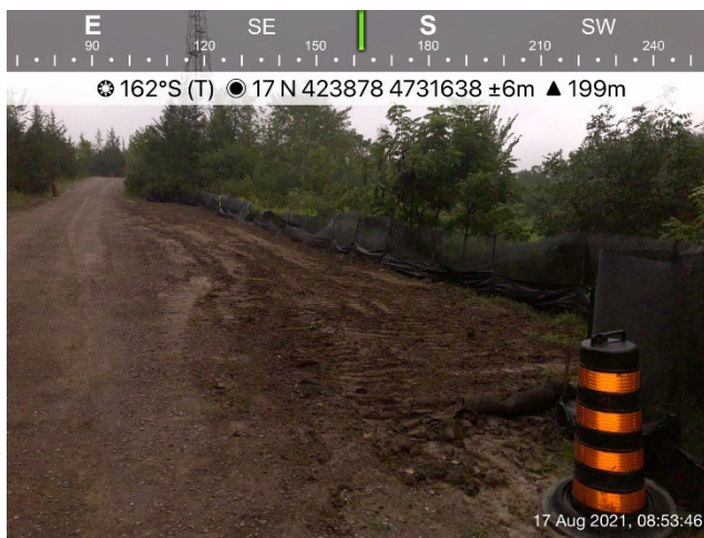
Photo 11: Sydenham River; HDD rig has been removed; Area has been graded and ready for seeding.
