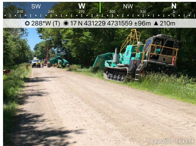
Photo 20: Installation of pipe with Spider Plough Crawler along Mossie Line west of Watterworth Road.
