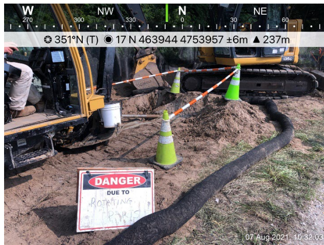
Photo 44: Crowe Creek; HDD drill set up along Glendon Drive.; Silt Soxx™ has been set in place in foreground. The dark silt fencing and turtle exclusion fencing are installed behind the hoe and drill rig.
