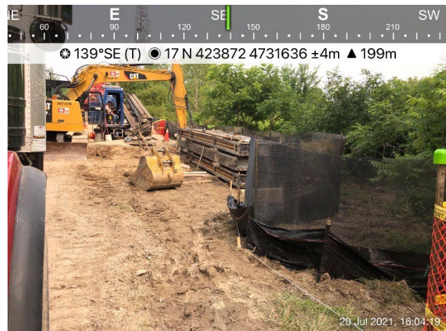
Photo 10: Sydenham River; HDD drill set up; Silt fencing & turtle exclusion fencing has been set in place.
