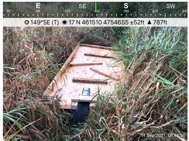
Photo 3839: WC105 open cut/dam and pump; Upstream dewatering hose attached to water energy deflector in grassy area.
