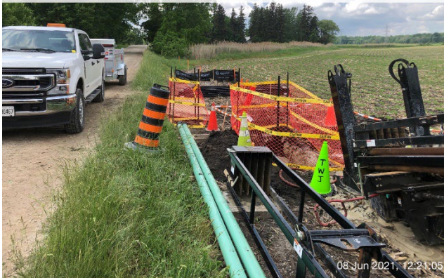
Photo 29: HDD setup while boring under WC81. Double silt fencing to capture inadvertent returns. Safety fencing around drill mud sump pit.
