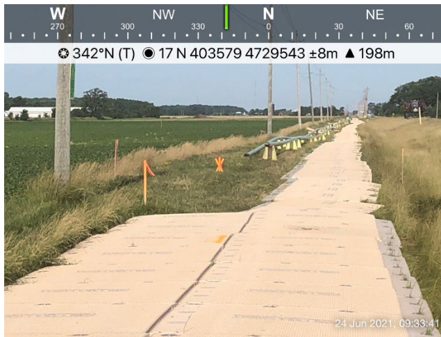
Photo 1: Rubber-polymer rig mats installed in farm field along Bentpath Line, west of Marthaville Road. Used to reduce soil compaction while installing new pipe.
