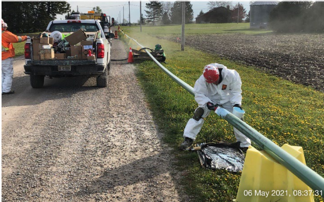
Photo 27: Sandblasting and coating welded pipe along Falconbridge Drive, east of Thames Road. Drop sheet used to collect any dripping epoxy coating.
