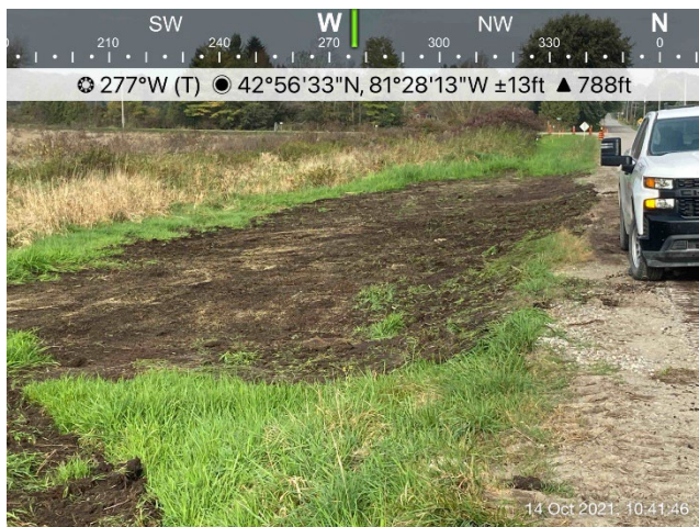
Photo 43: WC105 open cut/dam and pump in background. In foreground, tie in north of WC106; has been graded, topsoil added and seeded. Along Amiens Road,
