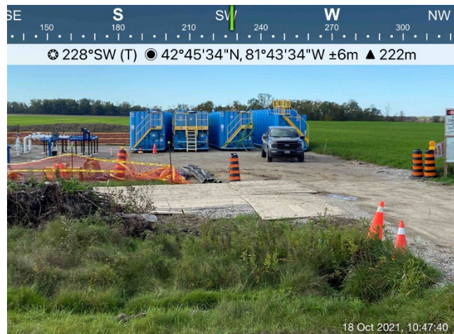
Photo 24: Glencoe Station; Hydrostatic test water being stored on frac tanks until release.
