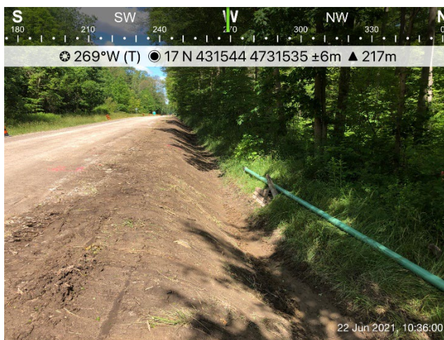
Photo 21: Mossie Line west of Watterworth Road. Reshaped road shoulder after pipe installation with Spider Plough. Ready for seeding..
