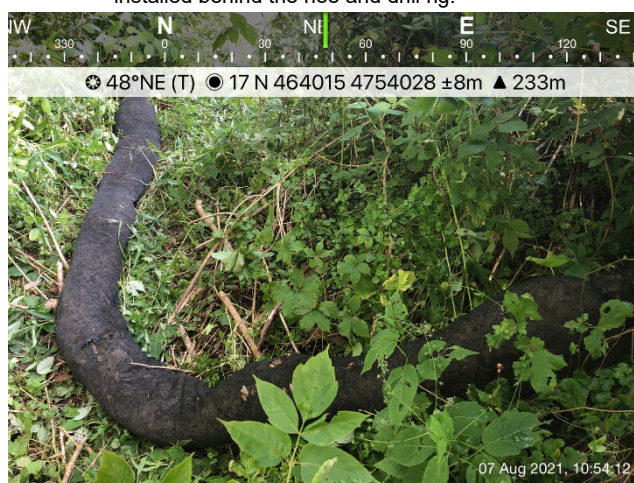
Photo 46: HDD along Glendon Dr under Crowe Creek; Silt Soxx™ on east bank of Crowe Creek.
