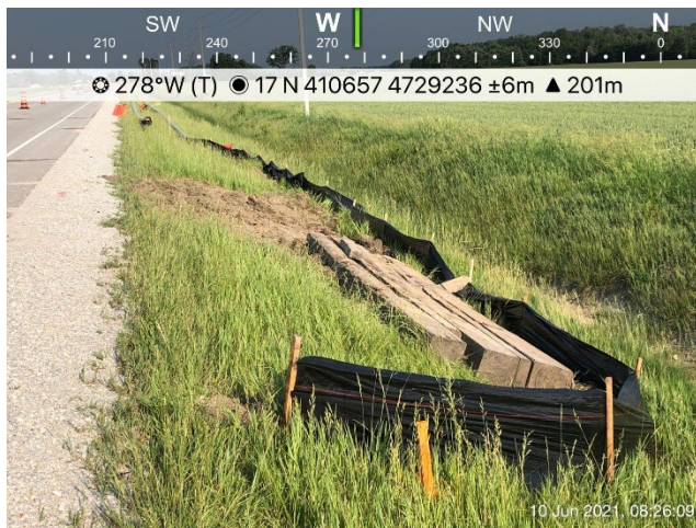
Photo 5: Silt fencing installed around HDD exit hole at Bentpath Line while boring under Gould Road.
