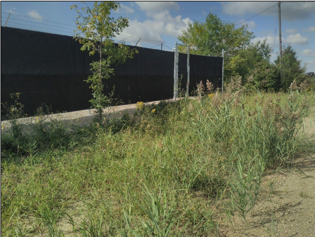
4. Restoration of drainage feature in road easement along Hwy 46.
