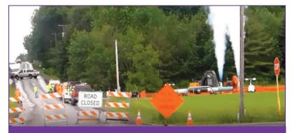
**Figure 3.** Blowdown for maintenance of a natural gas pipeline in Yates County, New York. Methane is an invisible gas, but the cooling from the rapid blowdown condenses water vapor, leading to the obvious cloud. Phot courtesy of Jack Ossont. Reprinted from Howarth (2019).<sup>3</sup>
