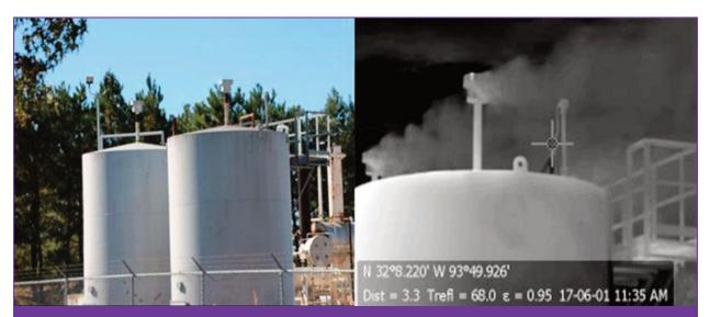
**Figure 2.** Natural gas storage tanks at the Haynseville, Texas, shale fields. Picture on left taken with a normal camera. Picture on right was taken with forward-looking infrared (FLIR) camera tuned to the infrared spectrum of methane, which allows visualization of methane emissions. Photo courtesy of Sharon Wilson. Reprinted from Howarth (2019).<sup>3</sup>
