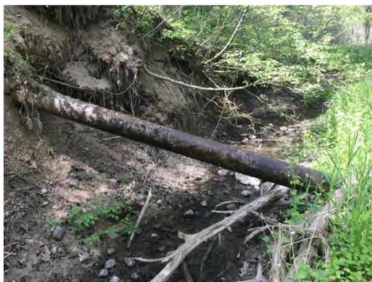
Figure 5.2-15: Erosion increasing the unsupported length of an aerial crossing
