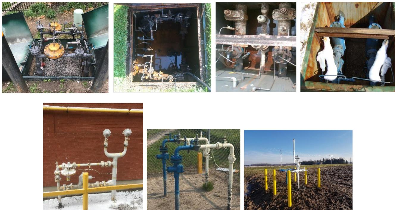
**Figure 5.2-66: Examples of Distribution System Stations**
