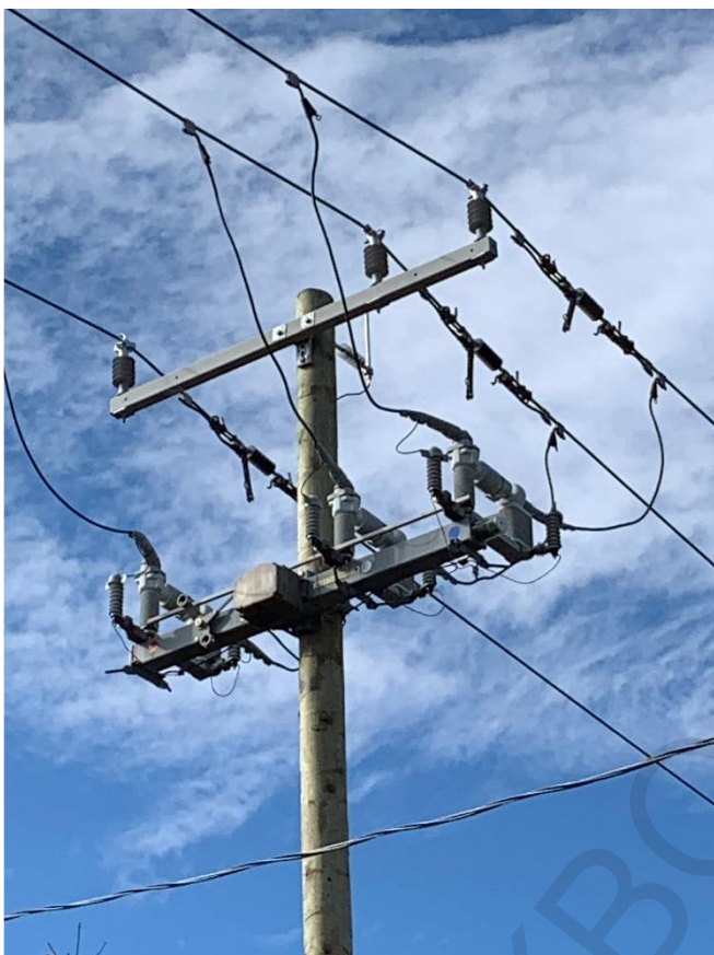
Intelligent (automated) switches
