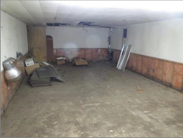
Major Concern: un-occupied room - existing flood damage Location: Basement
