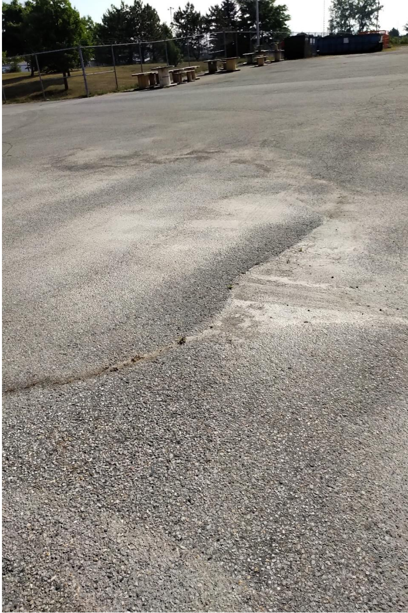
Back parking lot- minor cracking observed. Repairs/ filling required as preventative maintenance measure
