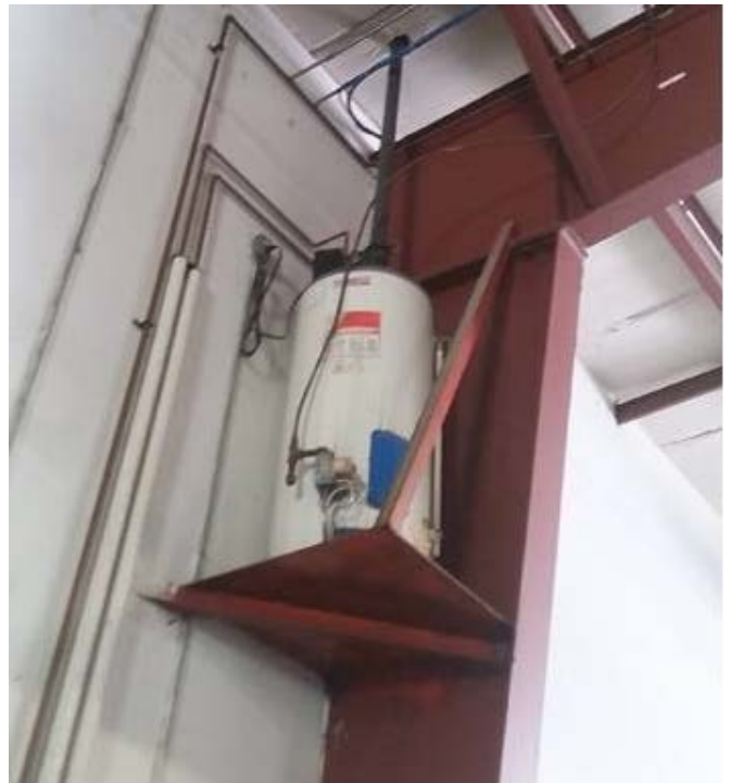
Gas Hot Water Heater Location: Garage
