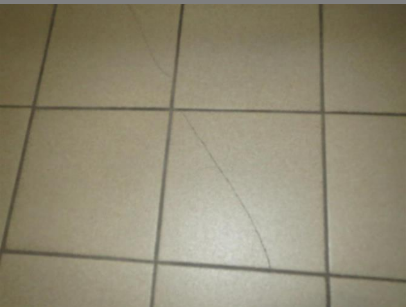
Ceramic tile in fair condition | nearing end of life cycle. Location: Corridor look at main reception
