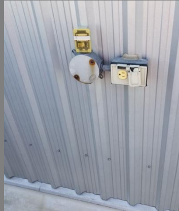
Broken Receptacle Cover Location: Roof
