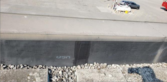
Parapet cap flashing and sample seals Location: 1986 Addition
