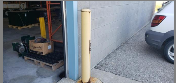
Bollard starting to rust Location: Garage
