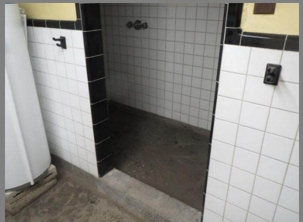
Major Concern: Basement flood. Sediment cover entire floor and unused shower. Location: Basement
