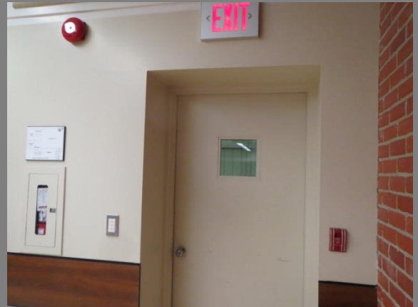
Door knob on exit door to be panic hardware.
