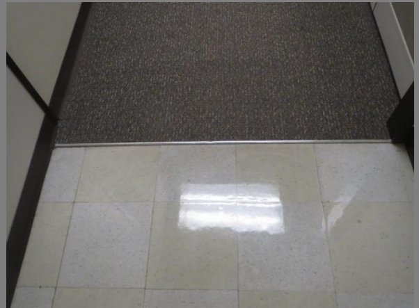
Flooring transition - VCT to Carpet Location: Office and open office area
