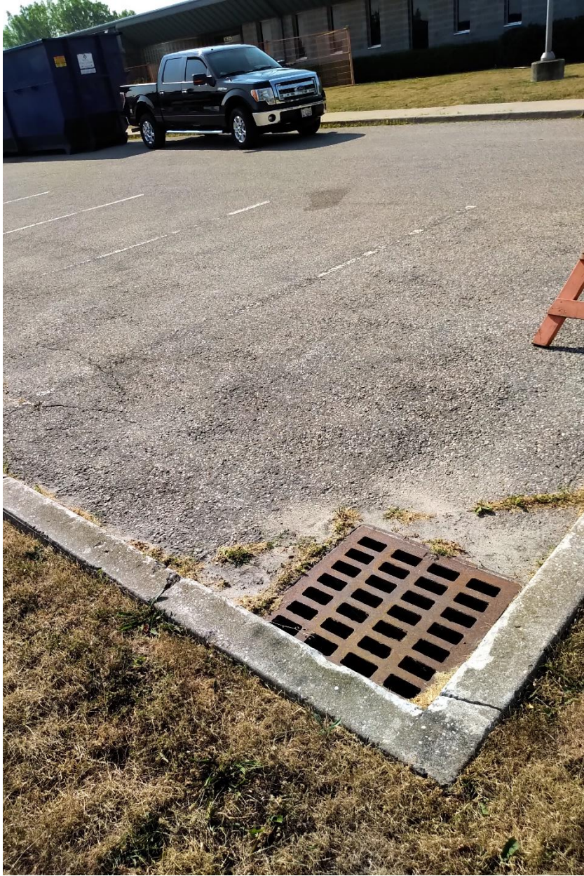
CB in visitor parking – no issues, sump and CB clean of debris
