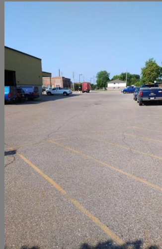
Monitor: Asphalt Cracking between CB's Location: New Pavement Area (east)
