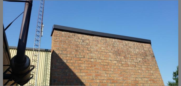
Repair: Cooling tower Wall flashing capped since 2015. Location: By Truck Bay
