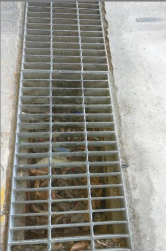
Trench drain cleaning required Location: Repair garage
