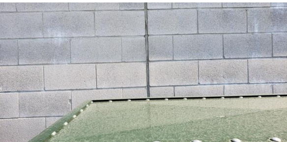
Repair: Control Joint Failing Location: Garage
