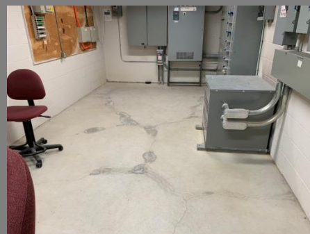
Slab on grade map cracking Electrical room
