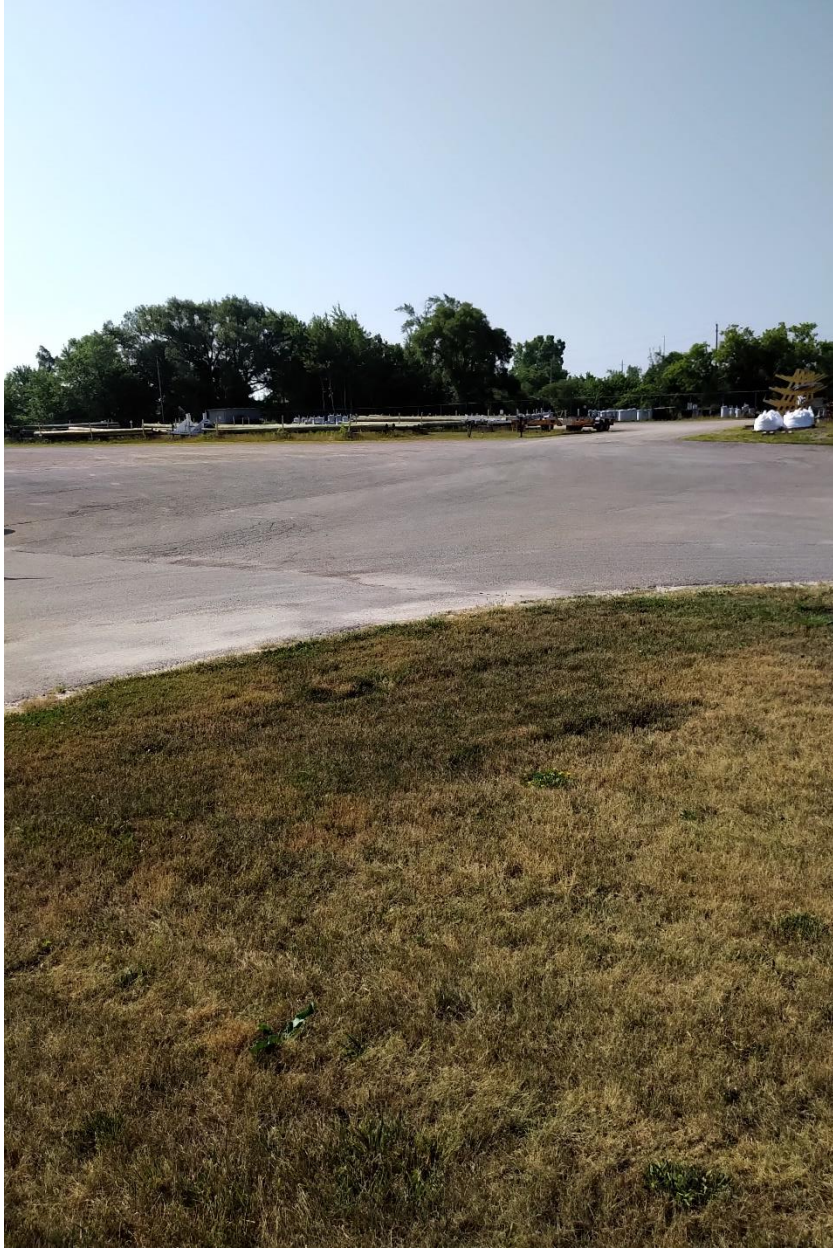
Back parking area, asphalt generally in good condition, some minor cracking. Cracks should be repaired and filled as a preventative measure
