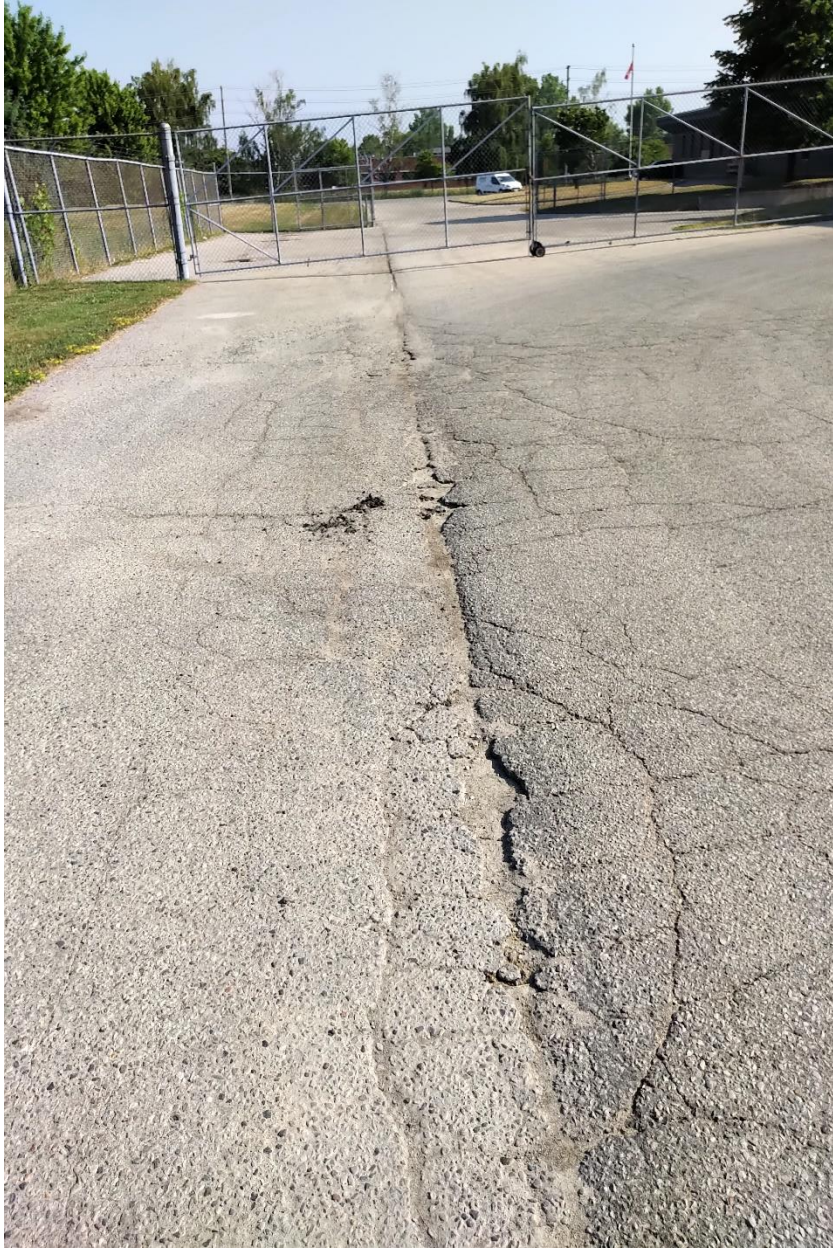
Front driveway – asphalt cracking and some separation along joint. Repair required to stop further damage and separation
