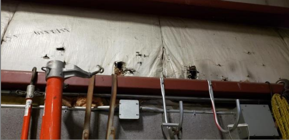
Repair: Damaged pre-eng insulation liner Location: Garage
