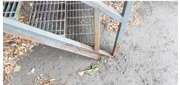
Repair: Rust forming on exposed Stairs Location: Loading Dock
