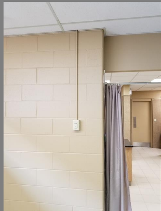
Wall Mounted Occupancy Sensor
