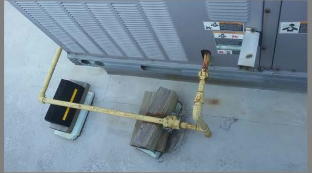
Gas piping serving HVAC Location: Roof
