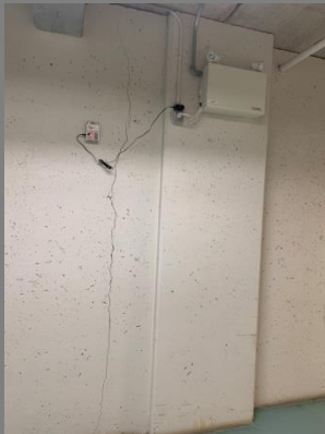
Cracks in Basement Walls
