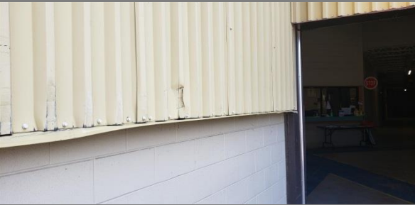
Repair: Siding Damaged Location: At Loading Dock
