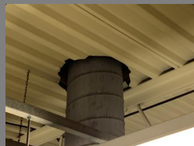
Roof penetrations Location: Storage room
