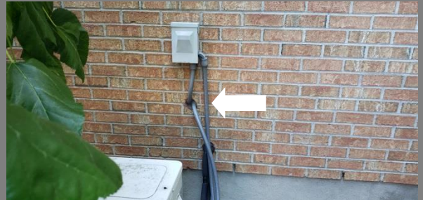
Penetrations sealed Location: West Courtyard wall
