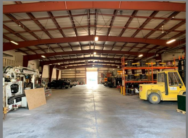
Pre-engineered rigid frame structure: Works Garage
