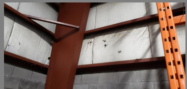
Repair: Damaged pre-eng insulation liner Location: Garage
