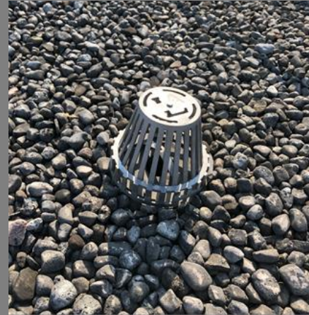
Roof drain with weir flow control device Location: Roof
