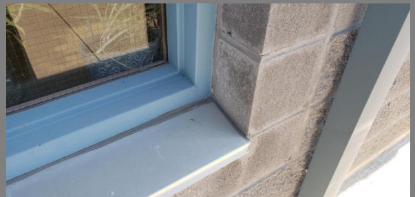
Sample of Hollow Metal Windows and Aluminum Sill Location: Main Office
