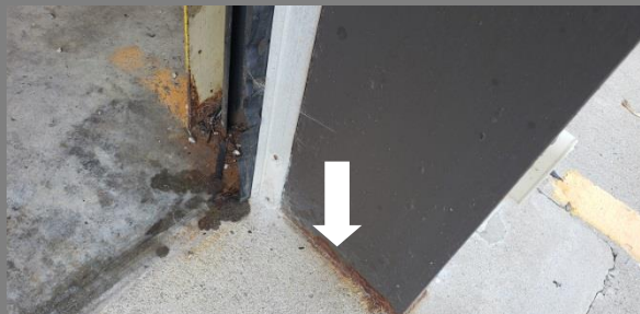
Rusting starting on Overhead Door Jamb Location: Truck Bay
