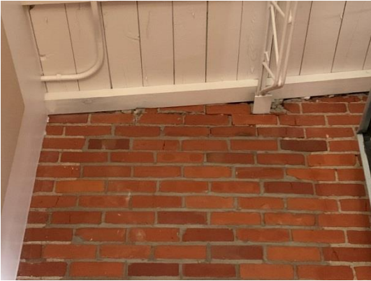
Mortar joint deterioration Location: Main Office
