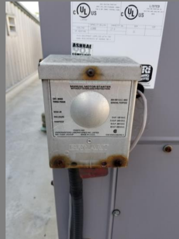
Rusty Rooftop Disconnect Switch Location: Roof
