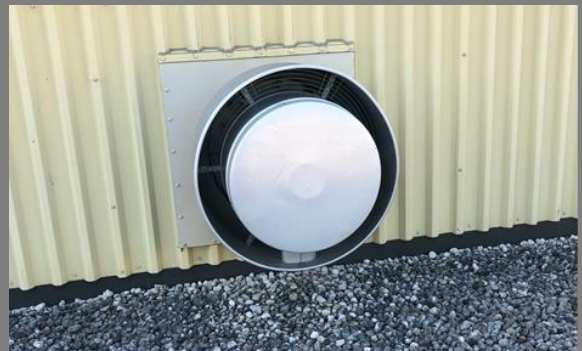
Exhaust fan through exterior wall Location: Lower Roof
