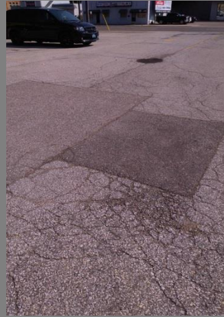
Asphalt in poor condition Location: East Parking Area
