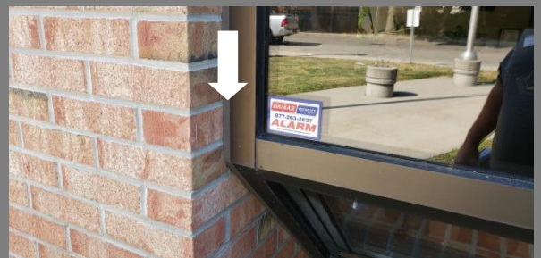
Sample of Caulking Location: 1986 Addition
