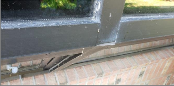
Frame gap repaired. Location: Main office – 2010 addition
