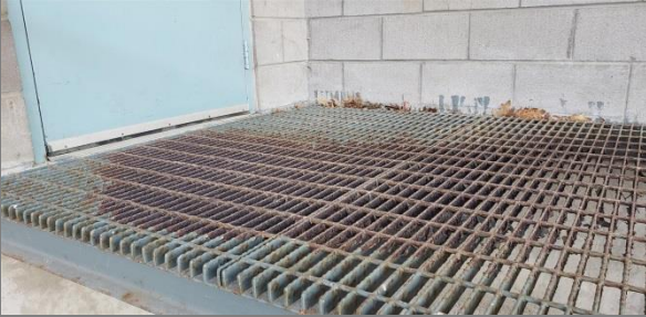
Repair: Rust forming on platform Location: Loading Dock
