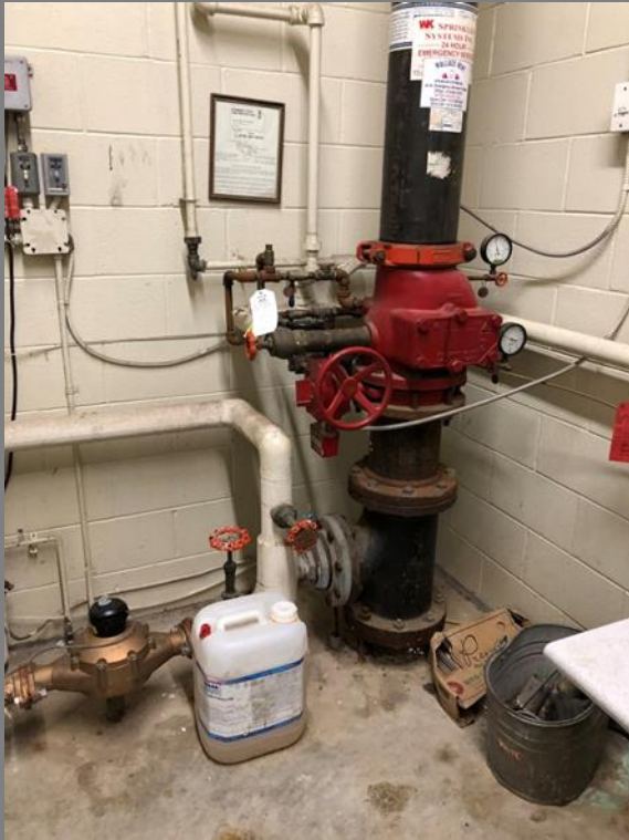
Domestic/Fire main in the Location: Mechanical Room
