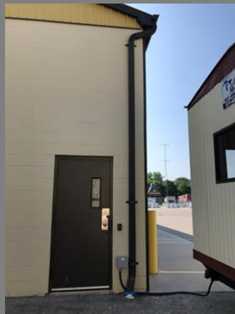
Exterior Storm water downspouts from Free Standing Garage
