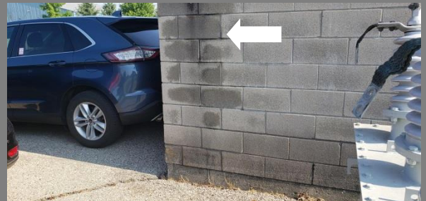
Moisture in Block by Garage, Monitor
