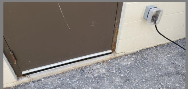
Repair: Door frame with rust starting Location: Works Garage
