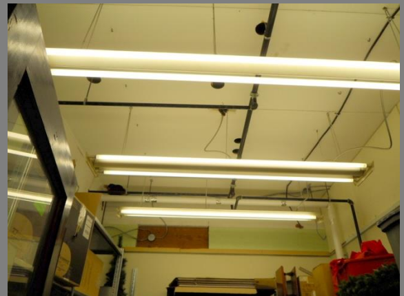
No floor to floor fire separation present in 1937 building.
