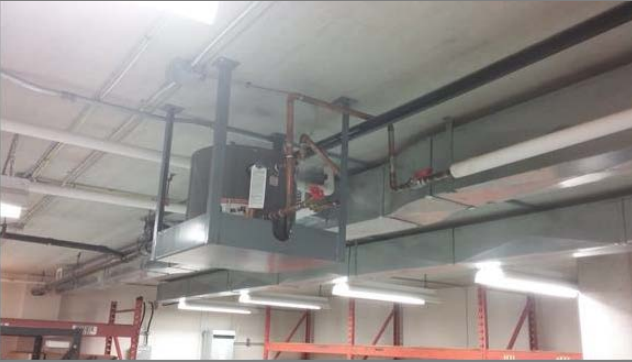
Suspended Electrical Hot Water Heater Location: Water Meter Room 011
