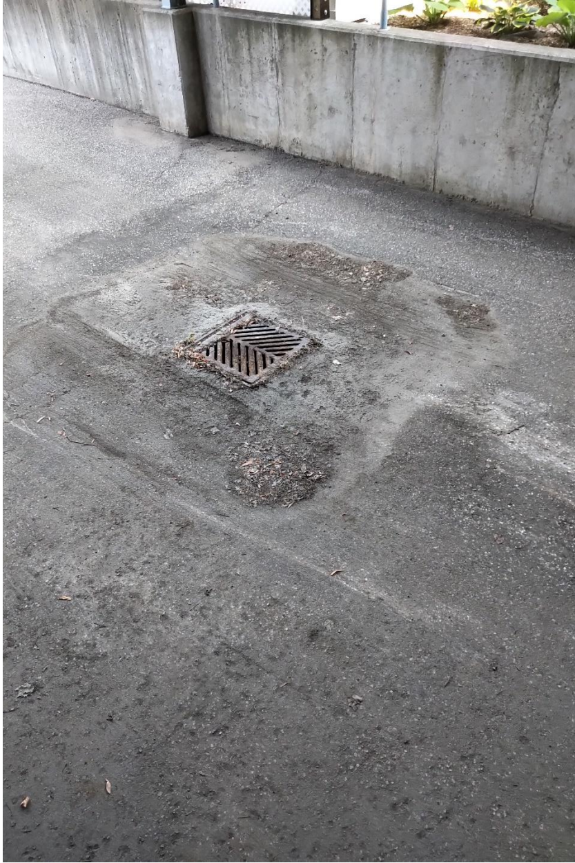
Driveway loading dock – some asphalt settlement around area that appears to have been repaired. Monitor to ensure cracking or further settlement does not occur
