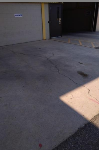
Monitor/Repair: Cracking in concrete apron Location: Rear of truck bay
