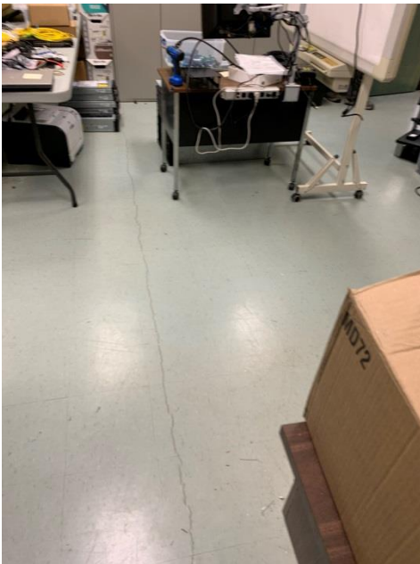
Crack in suspended floor: IT work Room.
