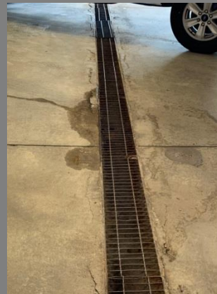
Existing trench drain in works garage
