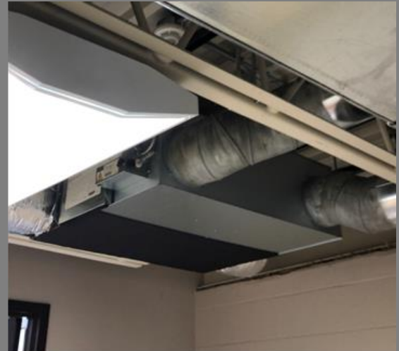
Energy Recovery Ventilator
