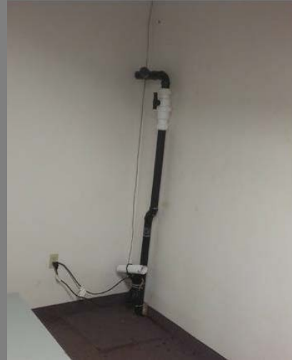
Weeping Tile Sump Pump Location: Basement Room 002
