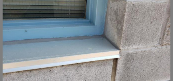
Sample: Caulking in good condition Location: Main Office
