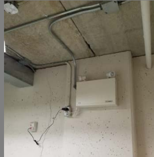
Remote Light Head/Battery Pack
