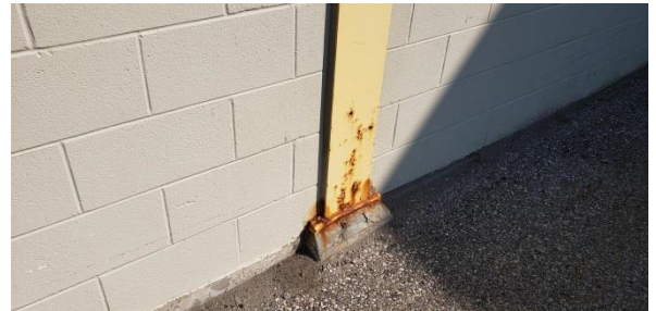
Repair: Rust forming on exposed columns Location: Various locations at Truck
