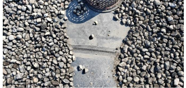
Overflow Re-seal joint starting to show wear. Location: 1986 Addition
