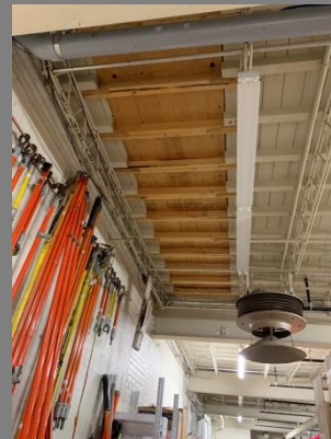
Infill of removed stair Location: Stores area
