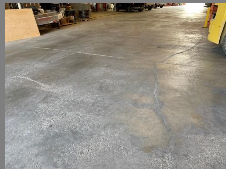
Slab on grade cracking and scaling Works Garage
