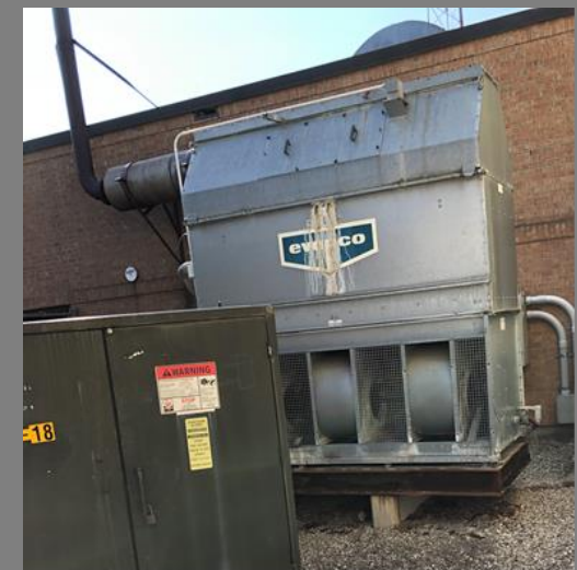
Closed Circuit Cooler
