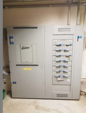
Electrical Service Switchboard Location:
