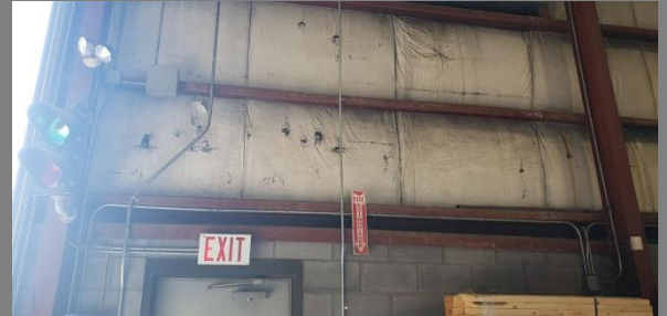
Repair: Damaged pre-eng insulation liner Location: Garage
