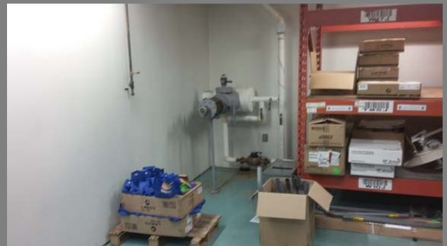
Existing Water Service Entering Building Location: Basement Room 011
