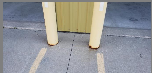
Repair: Paint Bollards due to rusting Location: Works Garage
