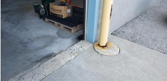
Concrete at door deteriorating Location: Garage
