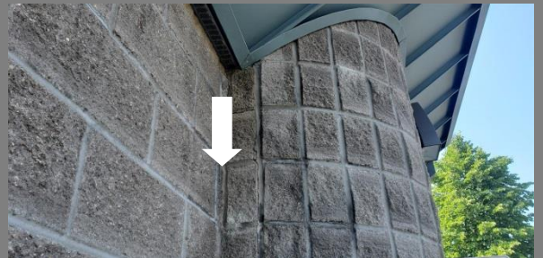
Minor cracking in architectural block
