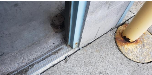
Sample: Rust staining on door frame Location: Garage
