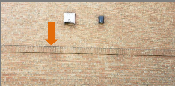
Repair: Discolouring of brick Location: 1937 Building
