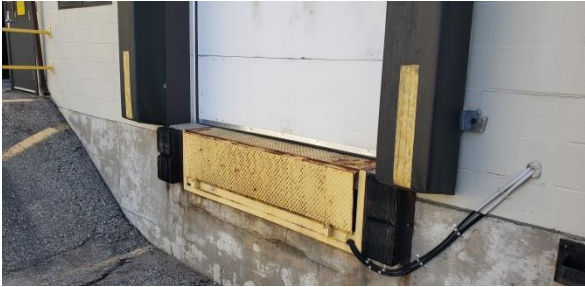
New seals around loading dock Location: Shipping & receiving
