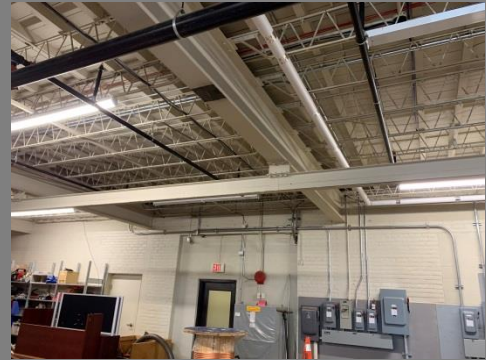
Monorail lift system Location: Stores area
