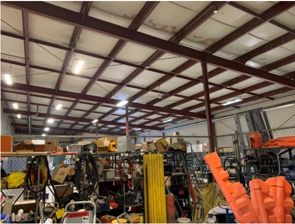
Pre-Engineered lean-to structure: Stores area
