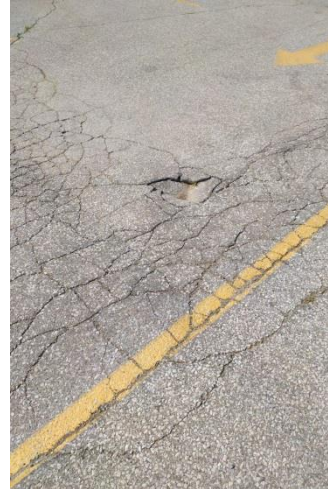
Repair: Small sink hole in asphalt & alligator cracking noted throughout Location: East parking lot
