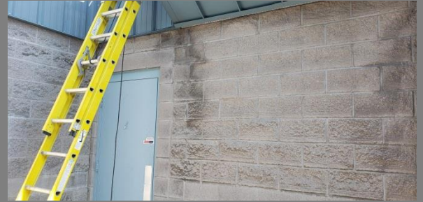
Discoloration of Architectural Block
