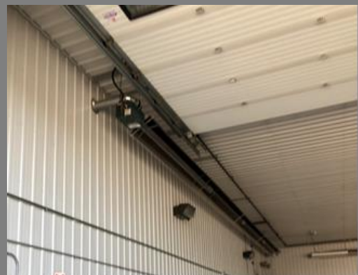
Gas fired heater Location: Garage
