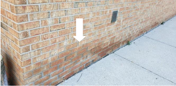
Brick repointed – no action Location: Main Entrance
