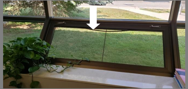
Repair: Glazing seal Location: 2010 Addition – North office
