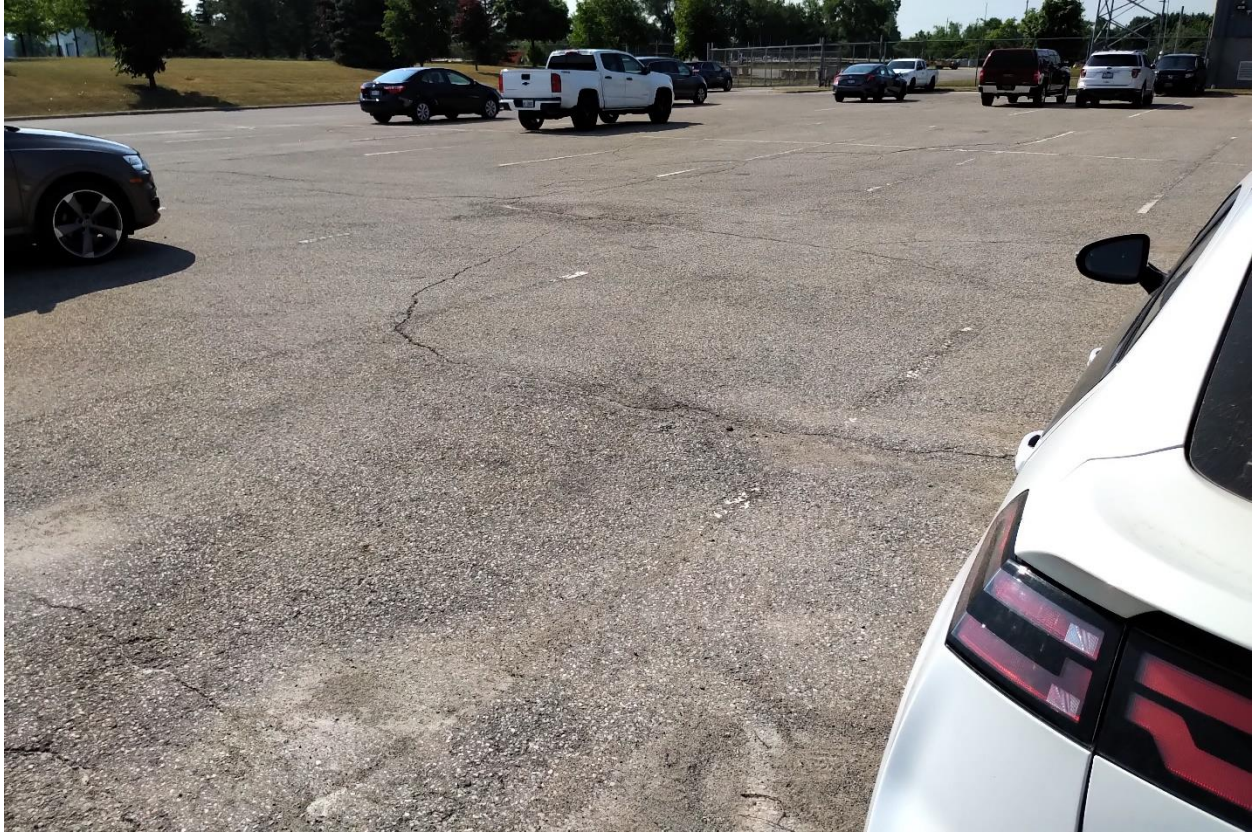
Employee parking – asphalt cracking noted in a few locations. Generally, asphalt in good shape. Minor repairs/ filling required. Monitor for further damage
