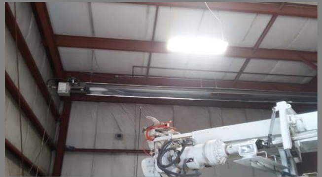
Gas fired heater Location: Garage
