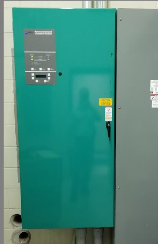
Automatic Transfer Switch
