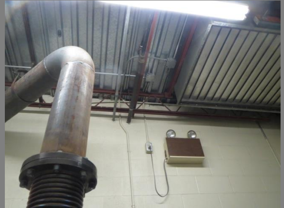
Flutes not sealed, penetrations not sealed. No Fire Separation around mechanical | electrical rooms.
