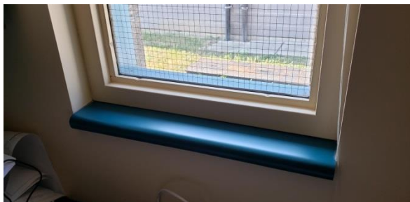
Sample: Hollow Metal Window stool in good shape. Location: Main Office Building
