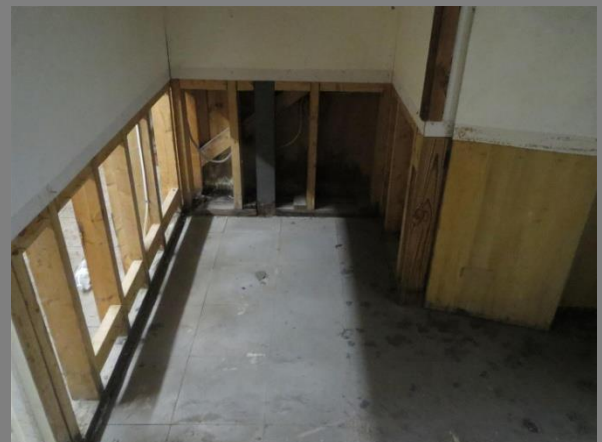
Major Concern: Plaster | Drywall removed at interior walls. Location: Basement
