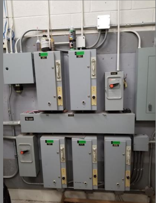
Mechanical Equipment Magnetic Starters
