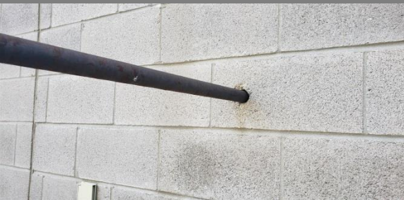
Penetration missing sealant Location: Garage
