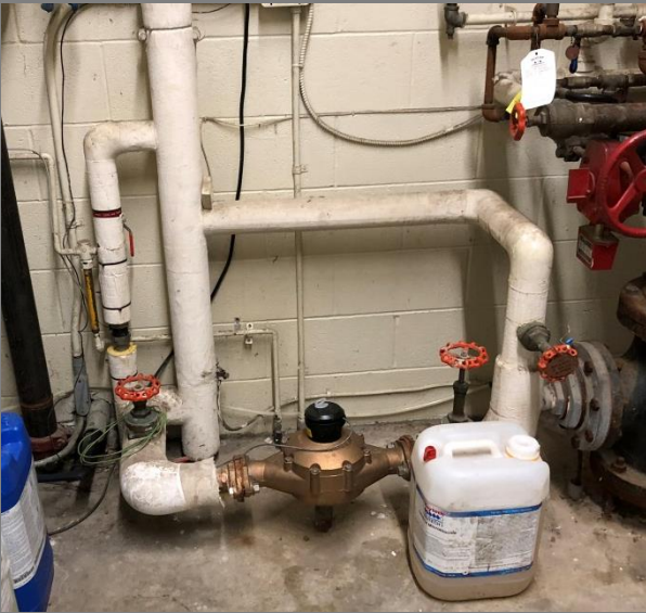
Existing water meter Location: Mechanical Room
