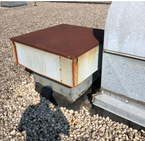
Rusted Supply Fan Hood Location: Roof
