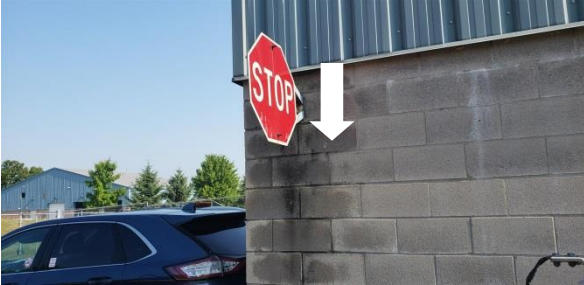
Moisture in Block by Garage, Monitor
