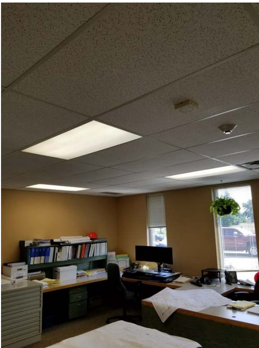
T8 Light Fixture & Ceiling Occupancy Sensor Location:
