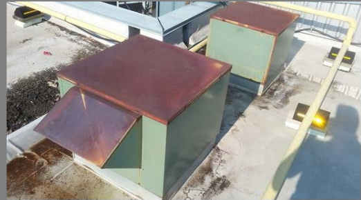
Rusted Exhaust Fan Hoods And Water on Flat Roof Location: Roof
