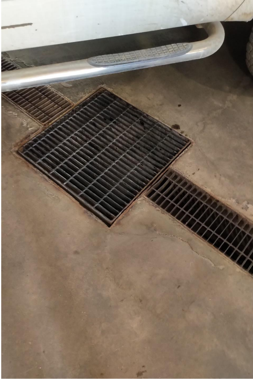
Trench Drain 2 – located in garage – clean and it good condition. CB grate clean and in good condition
