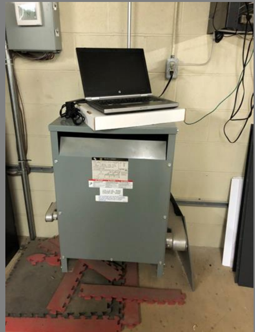
Transformer being used as a Work Station
