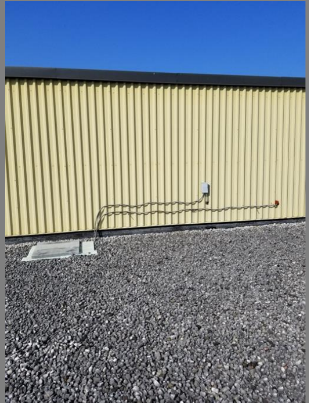
Abandoned Disconnect and Raceway Location: Roof
