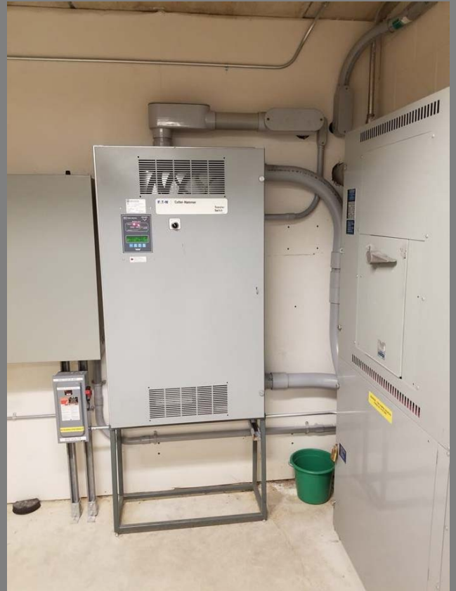
400A Automatic Transfer Switch Location:
