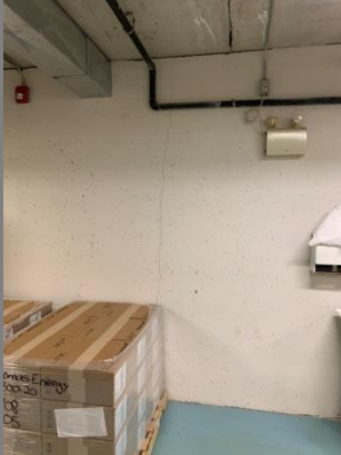
Cracks in Basement Walls
