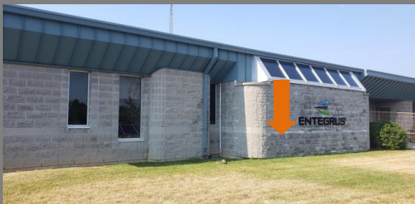
Repair: Discolouring of block Location: Main Entrance
