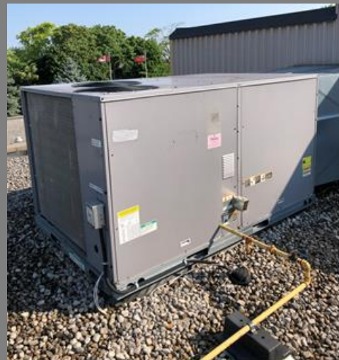
Gas piping serving HVAC Location: Roof
