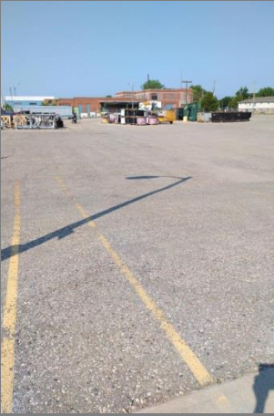
Asphalt in poor condition Location: South of Repair Garage
