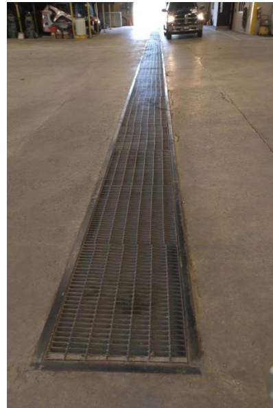
Trench Drain in Truck Bay Location: Truck Bay
