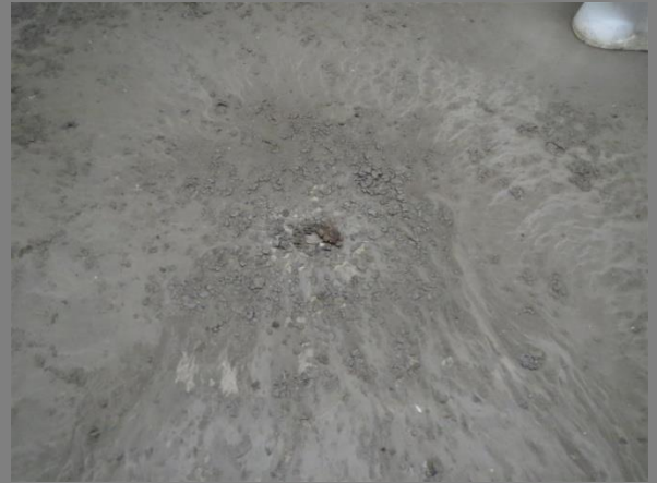
Major Concern: Capped floor drain. Sediment cover entire floor Location: Basement
