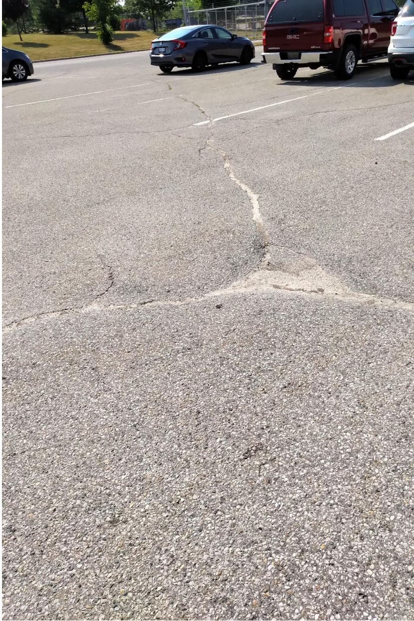
Employee parking – asphalt cracking noted in a few locations. Generally, asphalt in good shape. Minor repairs/ filling required. Monitor for further damage
