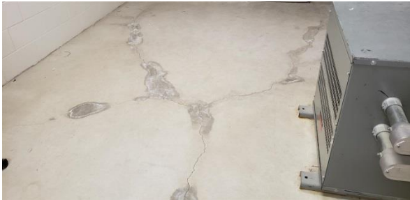
Signs of water infiltration (monitor) Location: Basement electrical room
