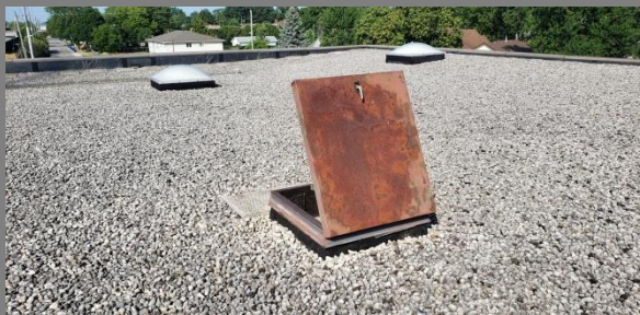
Roof Access Hatch - Rusting Location: 1986 addition
