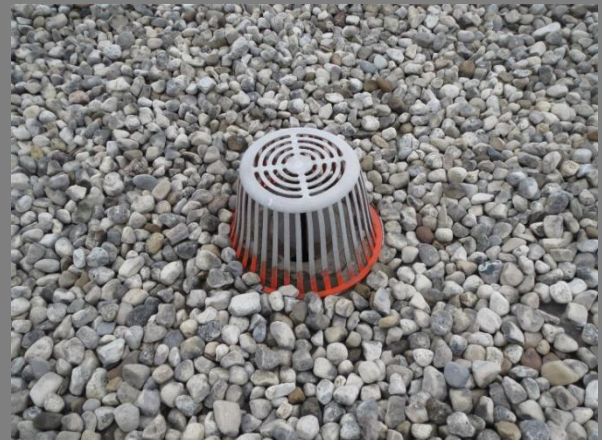
Roof Drain Location: 1986 Addition
