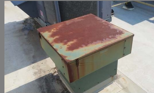
Rusted Supply Fan Hood Location: Roof
