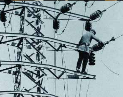
Left: Stringing of transmission line on steel towers in the Niagara area is shown in this photo, dated February, 1910.
