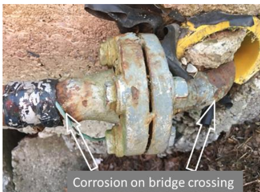
Figure 5.2-9: Severe corrosion on bridge-crossing pipe
