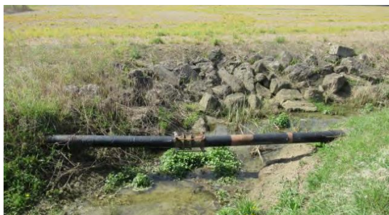
Figure 5.2-13: Aerial crossing with exposed mechanical fitting
