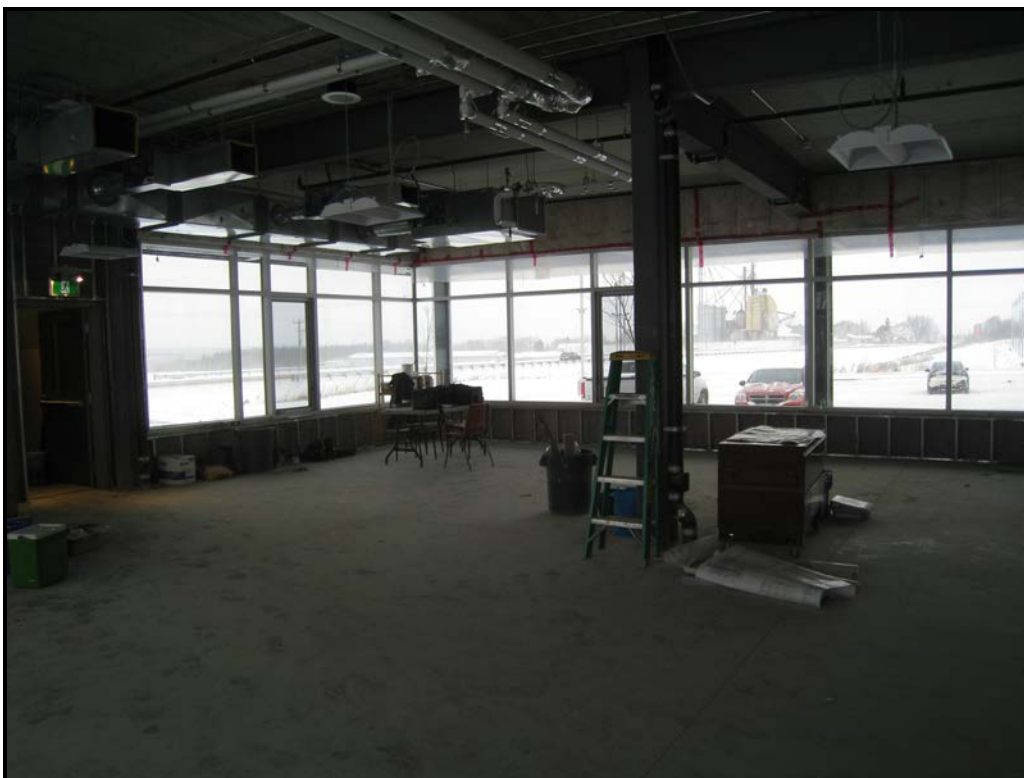
View of Main Level Unit
