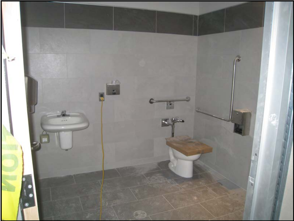
View of Bathroom
