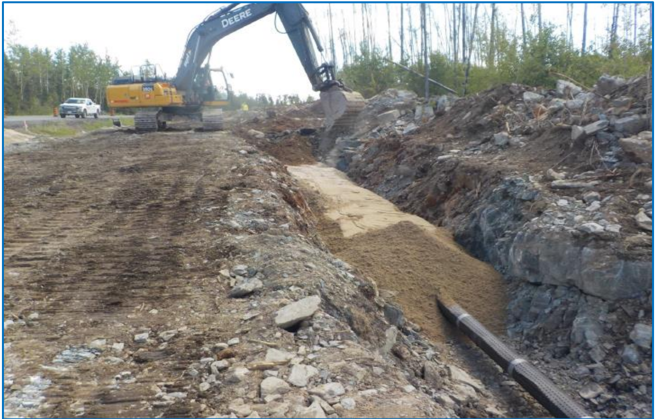
The pipeline is first backfilled with sand for protection from rocks before the natural fill is added.
