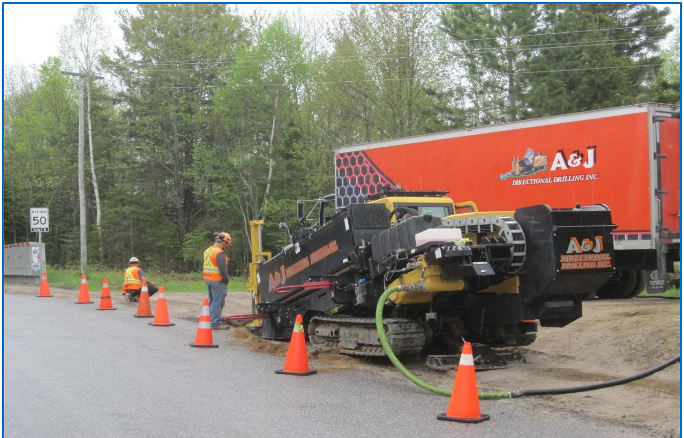
Horizontal directional drilling was used for all watercourse crossings and where ground conditions allowed.
