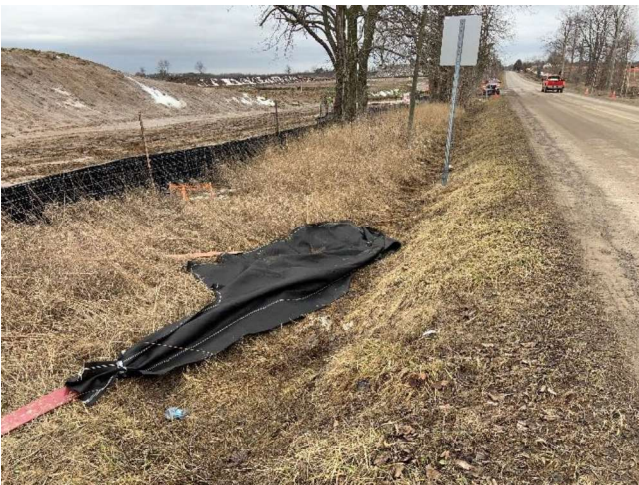
Photo 33: Sediment bag for pumping water. February 10, 2023 – Facing south.
