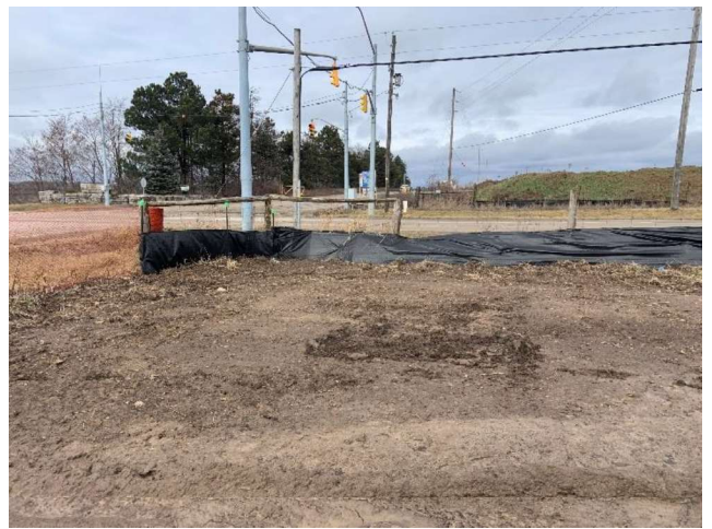
Photo 42: Silt fence was installed early in construction. January 20, 2023 – Facing north.
