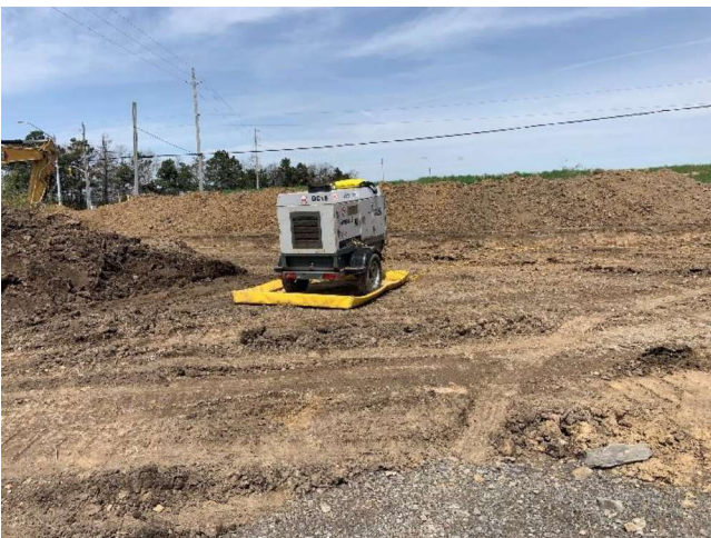
Photo 29: Portable generator with spill protection in place. May 8, 2023 – Facing north.
