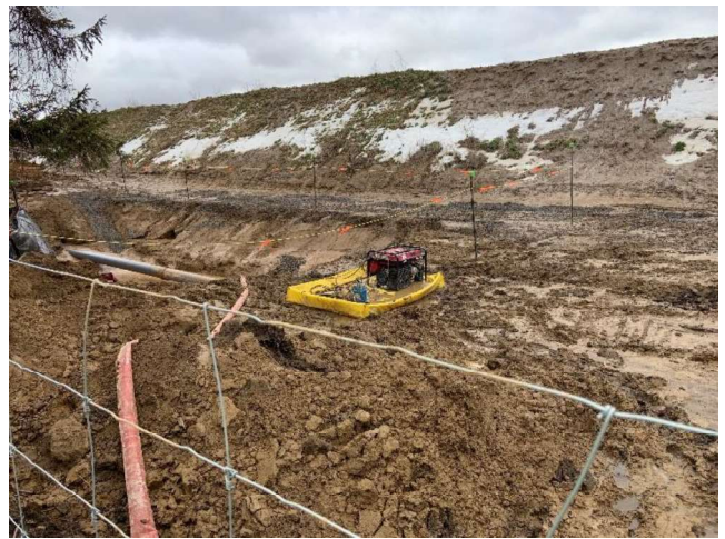
Photo 34: Portable generator protected from spills. February 10, 2023 – Facing south.
