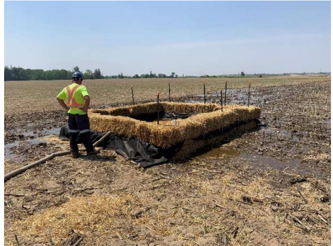
Photo 26: Sediment basin for hydrostatic test water discharge. June 6, 2023 – Facing west.
