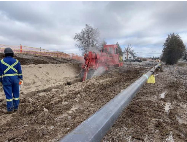
Photo 31: Bedrock grinder in action. March 7, 2023 – Facing north.
