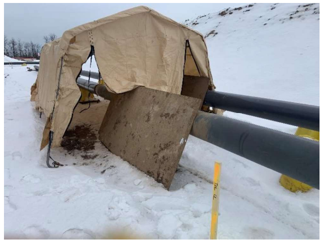
Photo 30: Plywood to catch drips and sand. January 30, 2023 – Facing east.
