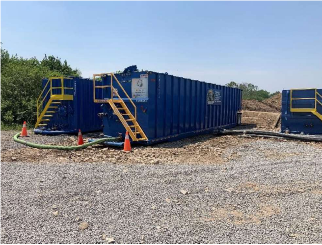
Photo 25: Weir tanks to hold hydrostatic test water. June 6, 2023 – Facing north.
