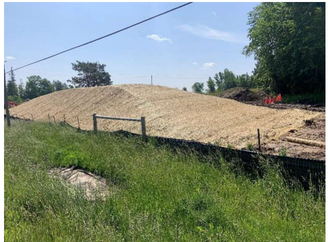
Photo 38: Erosion control matting installed to protect grades. June 13, 2023 – Facing east
