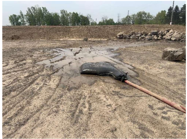
Photo 28: Dewatering of ponded water. May 19, 2023 – Facing south.
