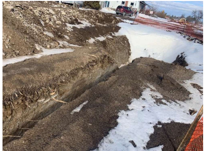
Photo 32: Trench dug by grinder. March 3, 2023 – Facing east.
