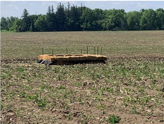
Photo 27: Sediment basin for hydrostatic test water discharge. June 6, 2023 – Facing south.
