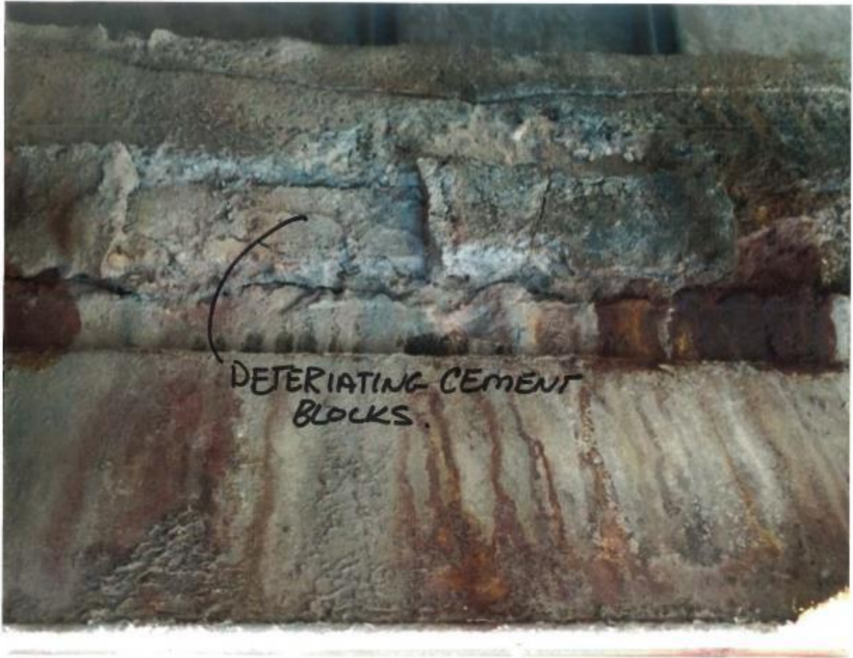
Figure A10 - 31: Lid Degradation: Cement crumbling
