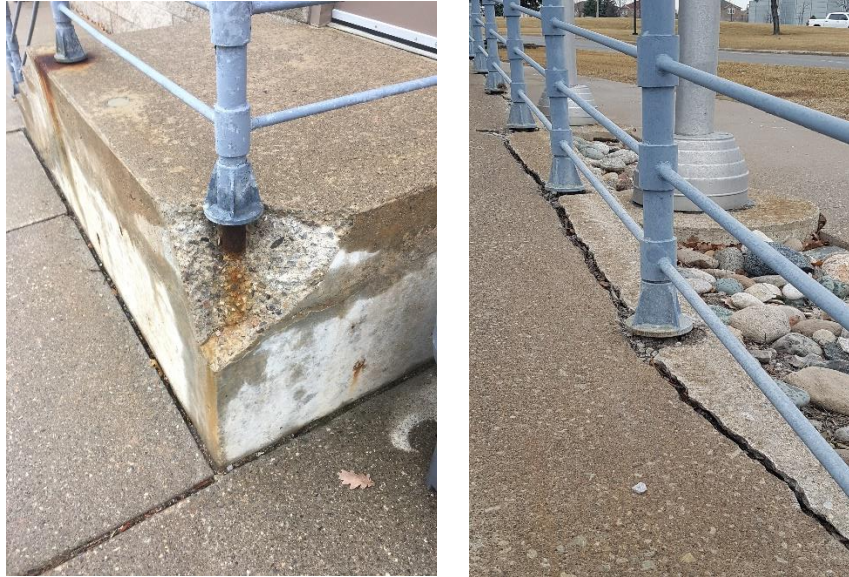
1 Figure A17 - 3: Water and Salt Damage of Wall at Sandalwood Parkway Building
