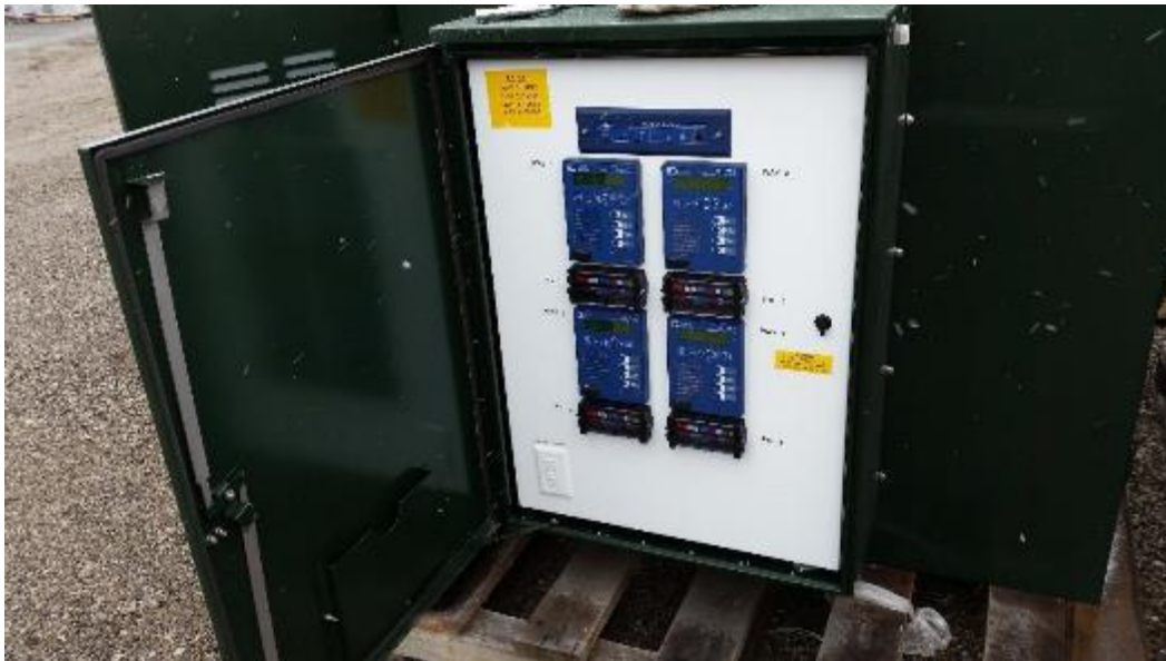
Figure A10 - 25: Automation Cabinet on Switchgear
