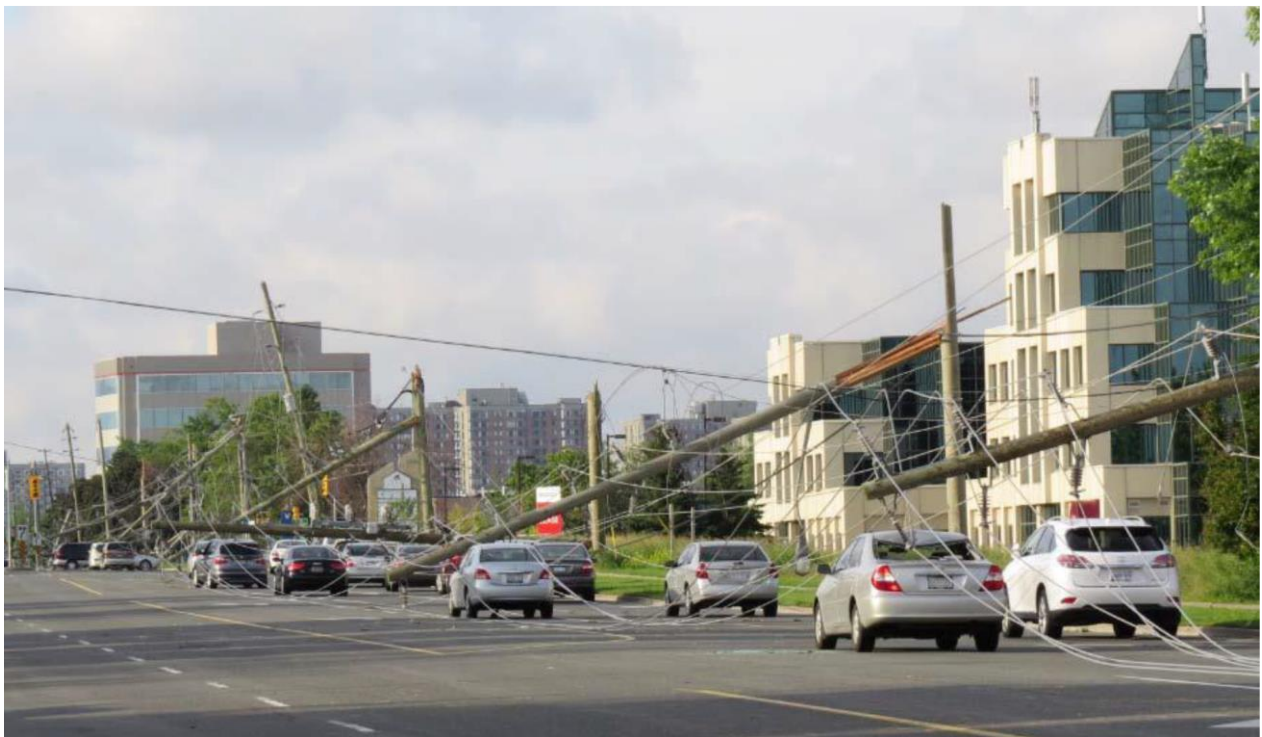
Figure A05 - 1: Downed Overhead Line on Warden Avenue in Markham in 2018
