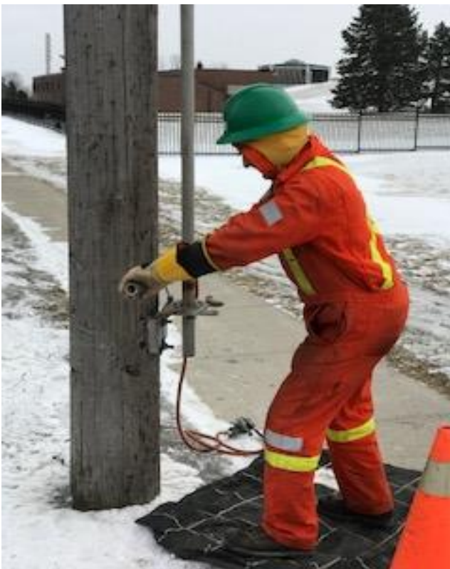
Figure A11 - 1: Manual Load Break Operation
