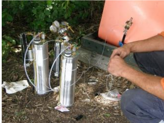
Figure A10 - 3: Underground Cable Rehabilitation by Cable Injection
