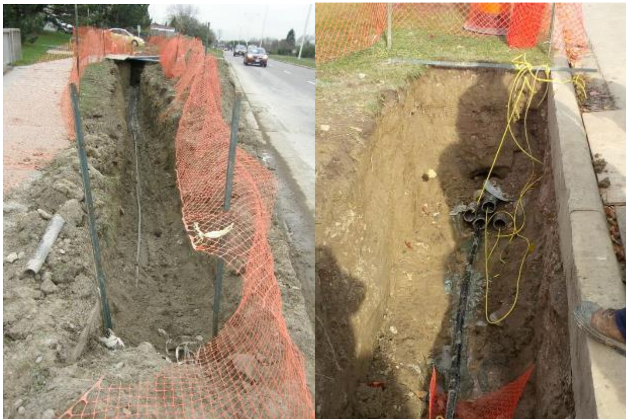
Figure A10 - 4: Underground Cable Replacement
