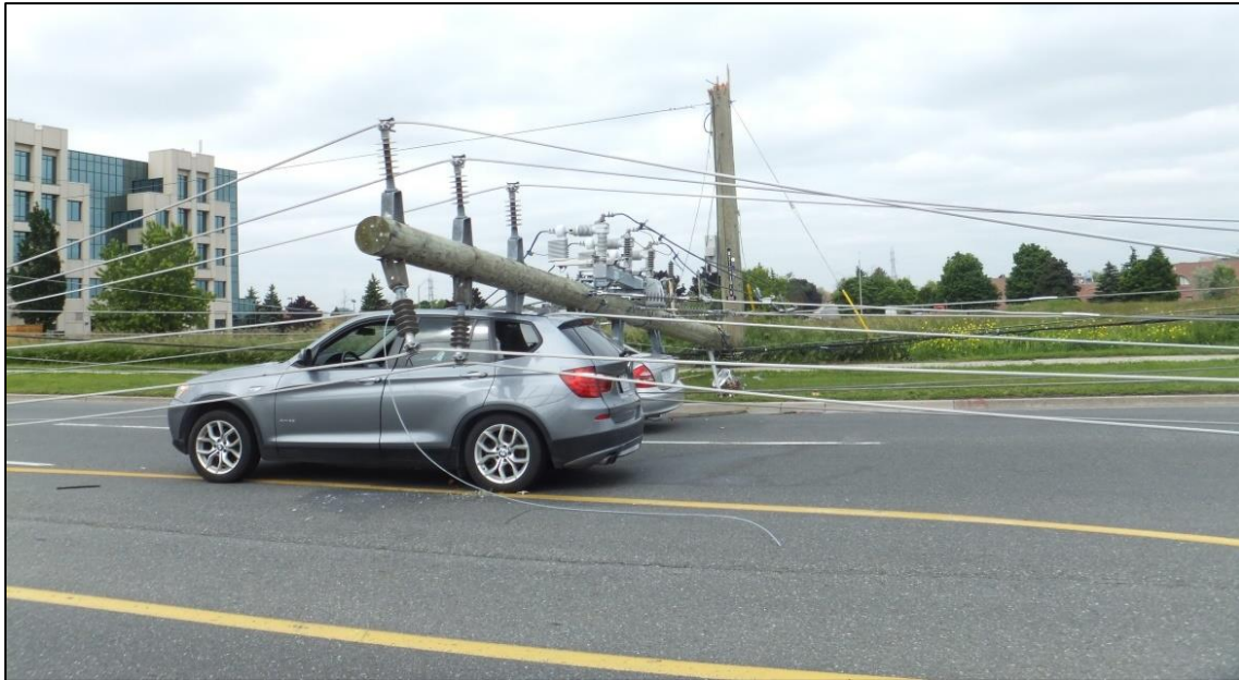
3 4 5 Figure 5.3.3 - 19: Failure of Legacy Wood Pole on Islington Avenue in Vaughan on October 15th, 2017
