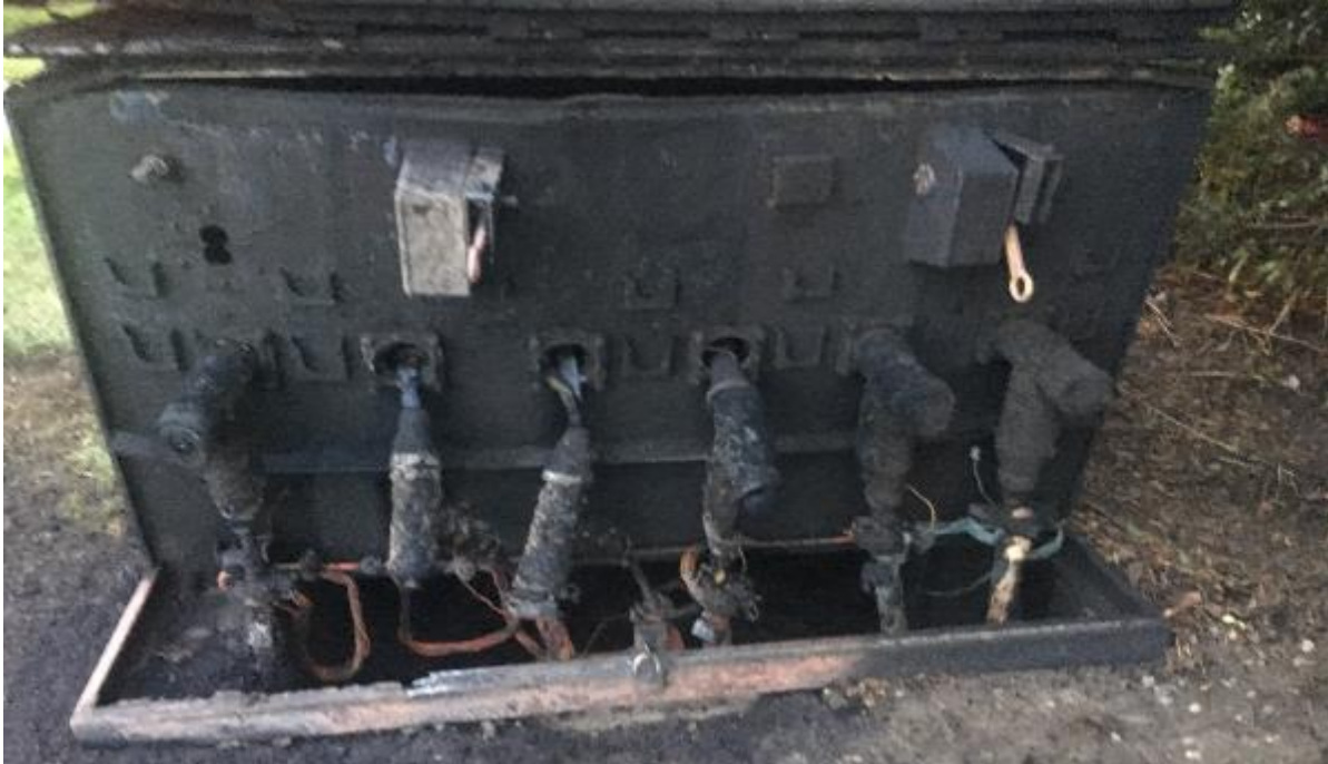
Figure A10 - 22: Failed Oil Filled Padmounted Switchgear
