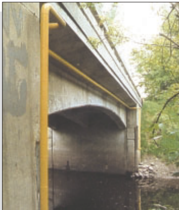
Attaching gas line on a bridge.
