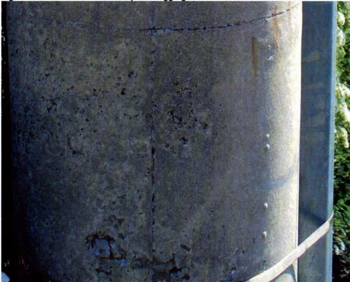
Figure 15 Concrete Pole with Exposed Aggregate
