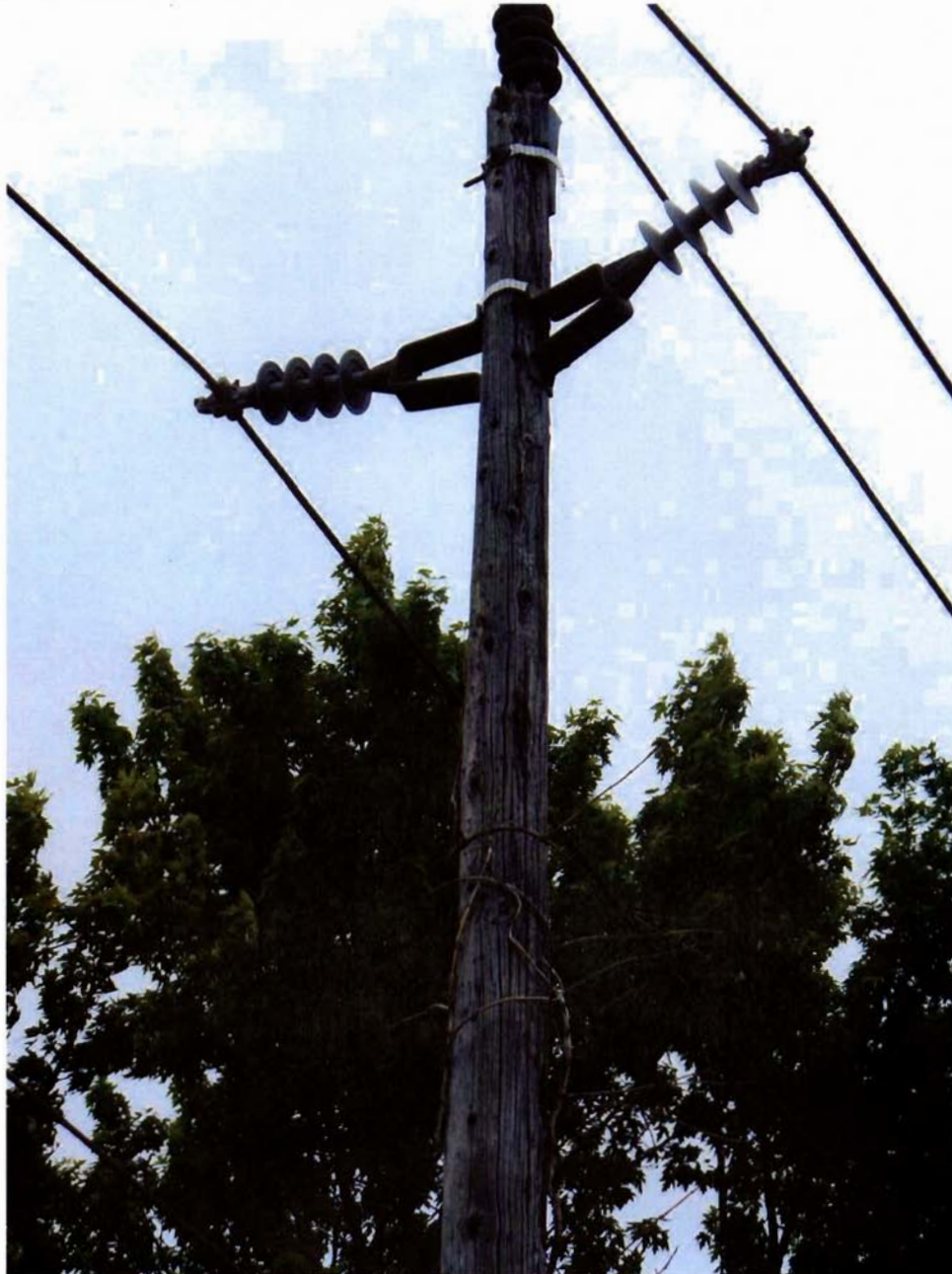
Figure 13 Old Pole with New Insulators
