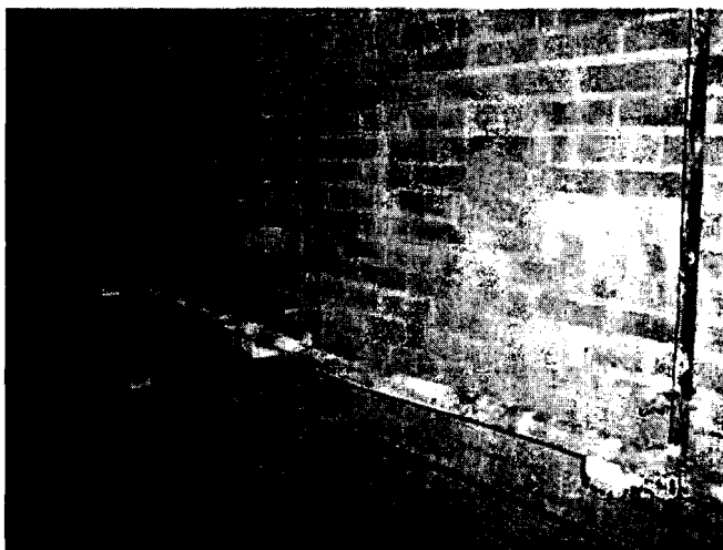
North Wall (West to East)
